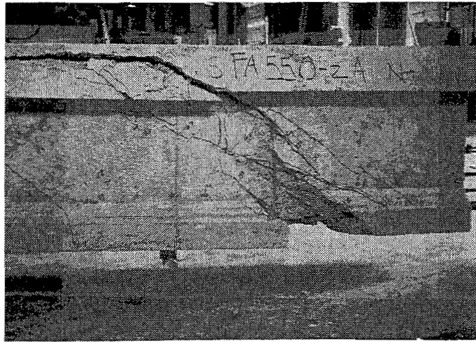
Figure 4.13 Photograph of FA550-2A Explosive Shear Failure
