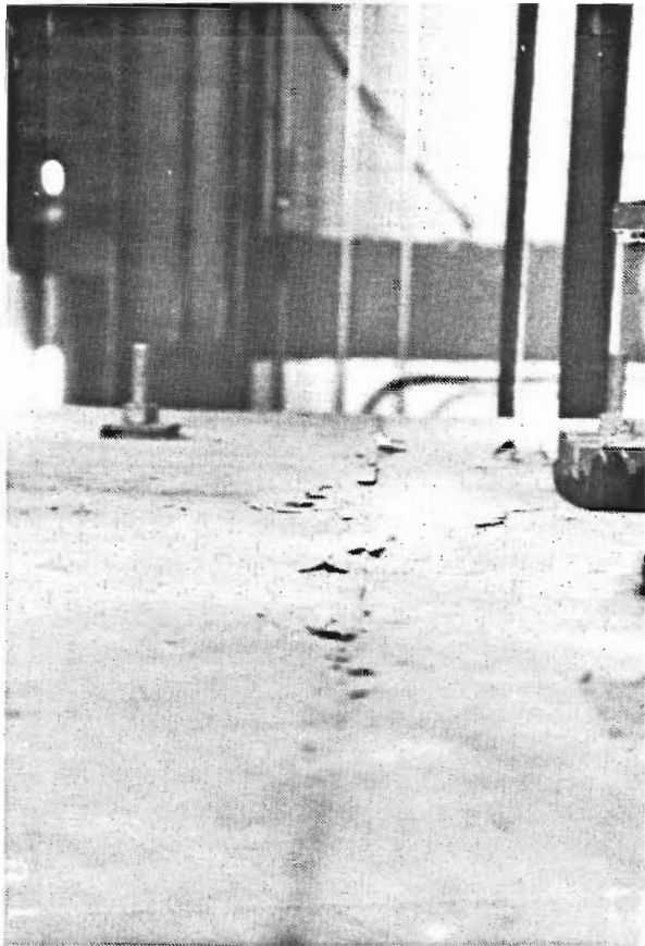
Figure 3.120 Crushed critical joint top flange.
