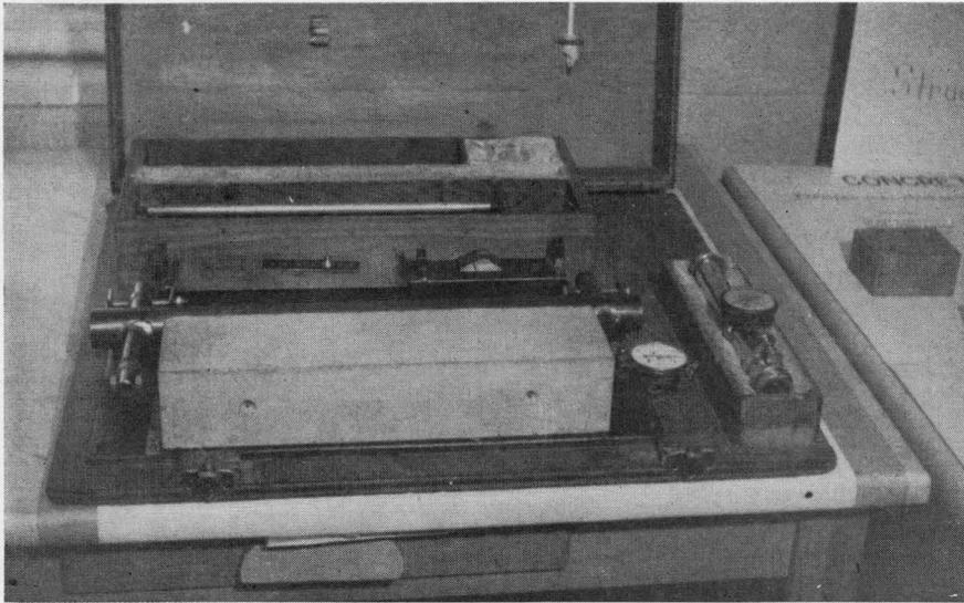
Figure 7. Device for measuring shrinkage using gage points cast in ends of specimen.
