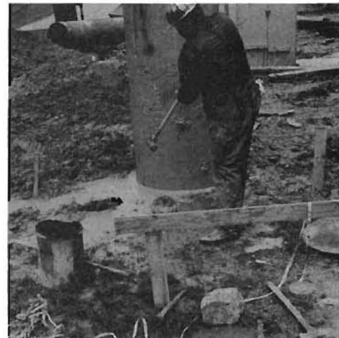
d. Drilling Mud Flowing Up from Around Casing
