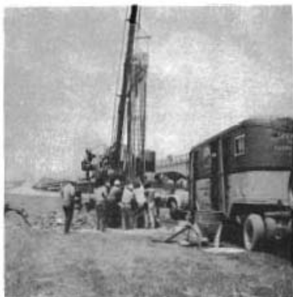
a. Placing Instrumented Cage in Borehole
