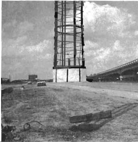
c. Pad in Place
