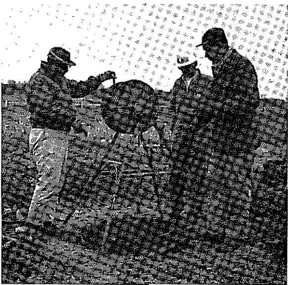
Fig 39. Apparatus used to lower man into San Antonio shaft to install cells.
