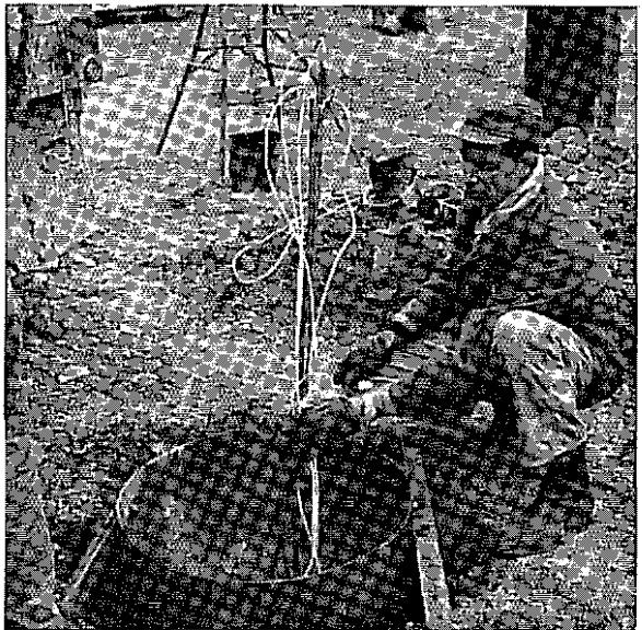
Fig 40. Cell leads protruding from San Antonio shaft after installation.
