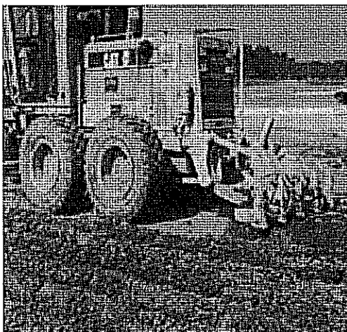
a) Scarification of base material ( www.lime.org )
