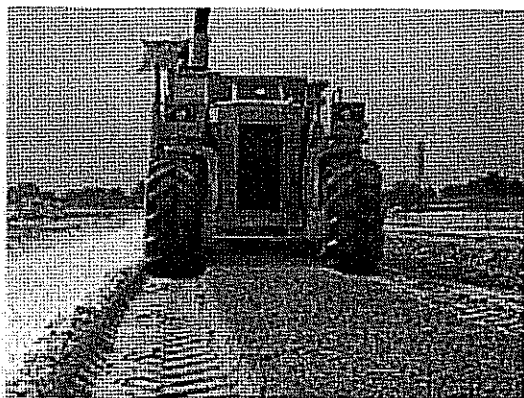
a) Mixing of lime and fly ash ( www.lime.org )
