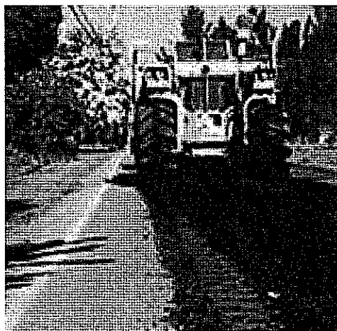
b) Pulverization of asphalt and base ( www.cement.org )
