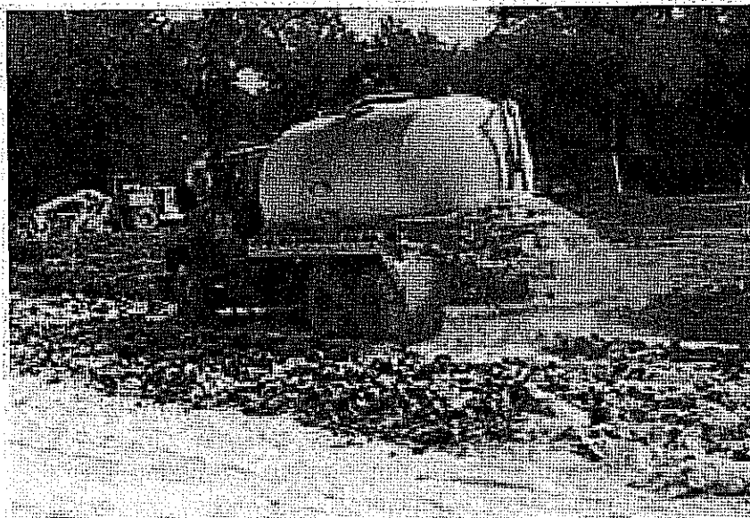
Figure 2.9 - Adding Water after Dry Stabilizer Application ( www.lime.org )
