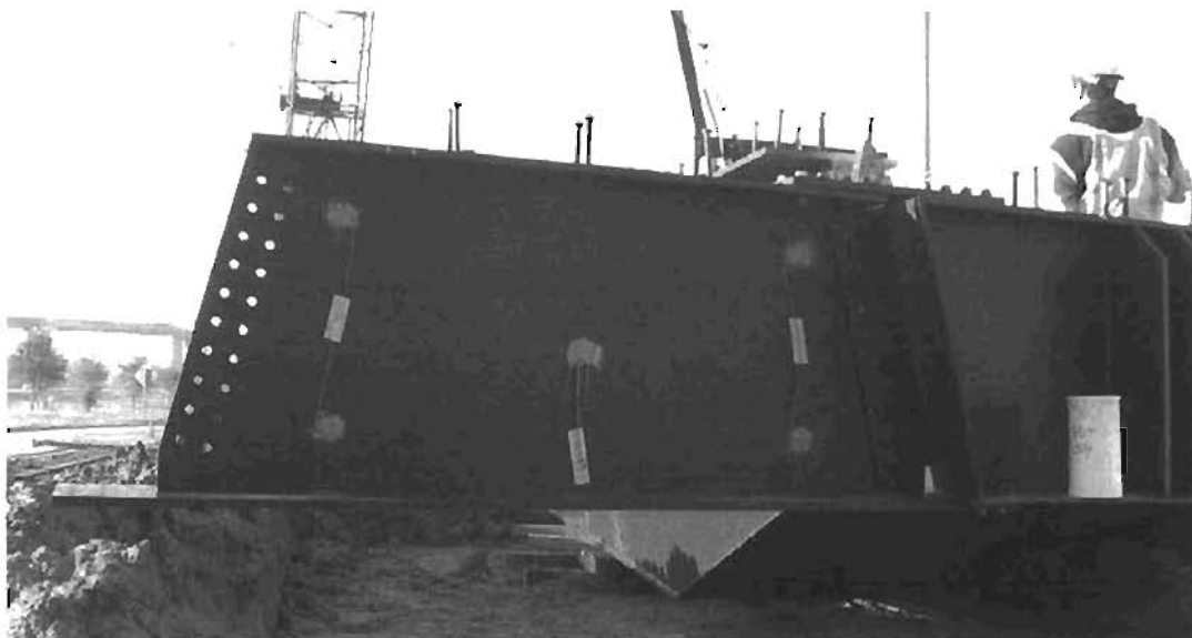
Figure 4.10 Solid External Diaphragm
