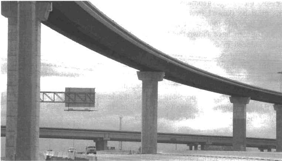
Figure 1.1 Trapezoidal Box Girder Bridge
