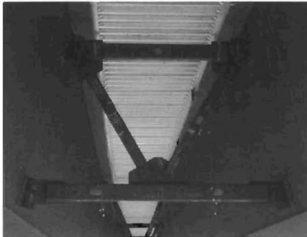
Figure 4.13 Temporary External Cross-Frame
