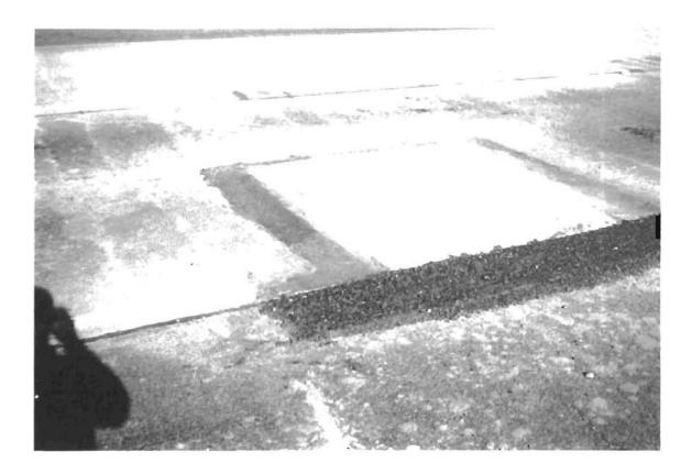
Fig 12. Completed 6' x 6' precast repair.
