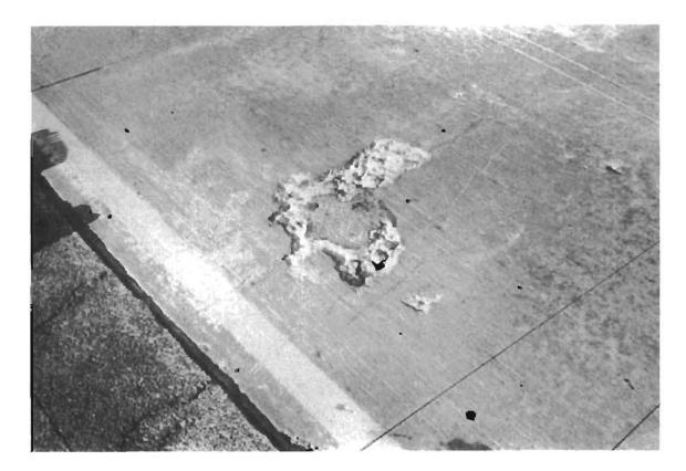
Fig 6. Repair area showing punchout
