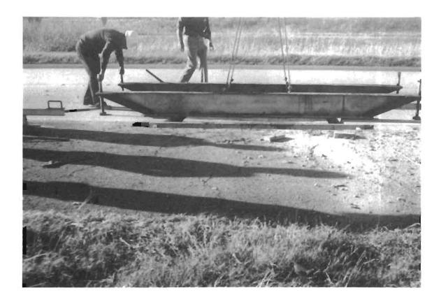
Fig 10. Precast repair showing leveling beams.
