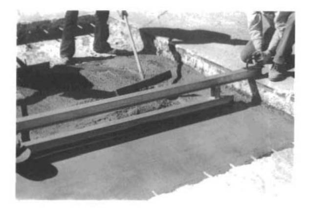
Fig 9. Work area showing bedding grout.
