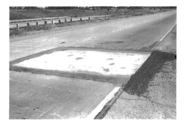
Fig 11. Completed 12' x 12' precast panel repair.
