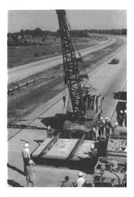
Fig 7. Repair area ready to receive precast slab.
