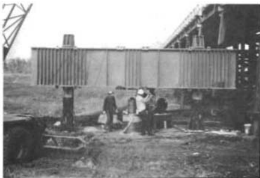
a. Reaction Beam - Test 1
