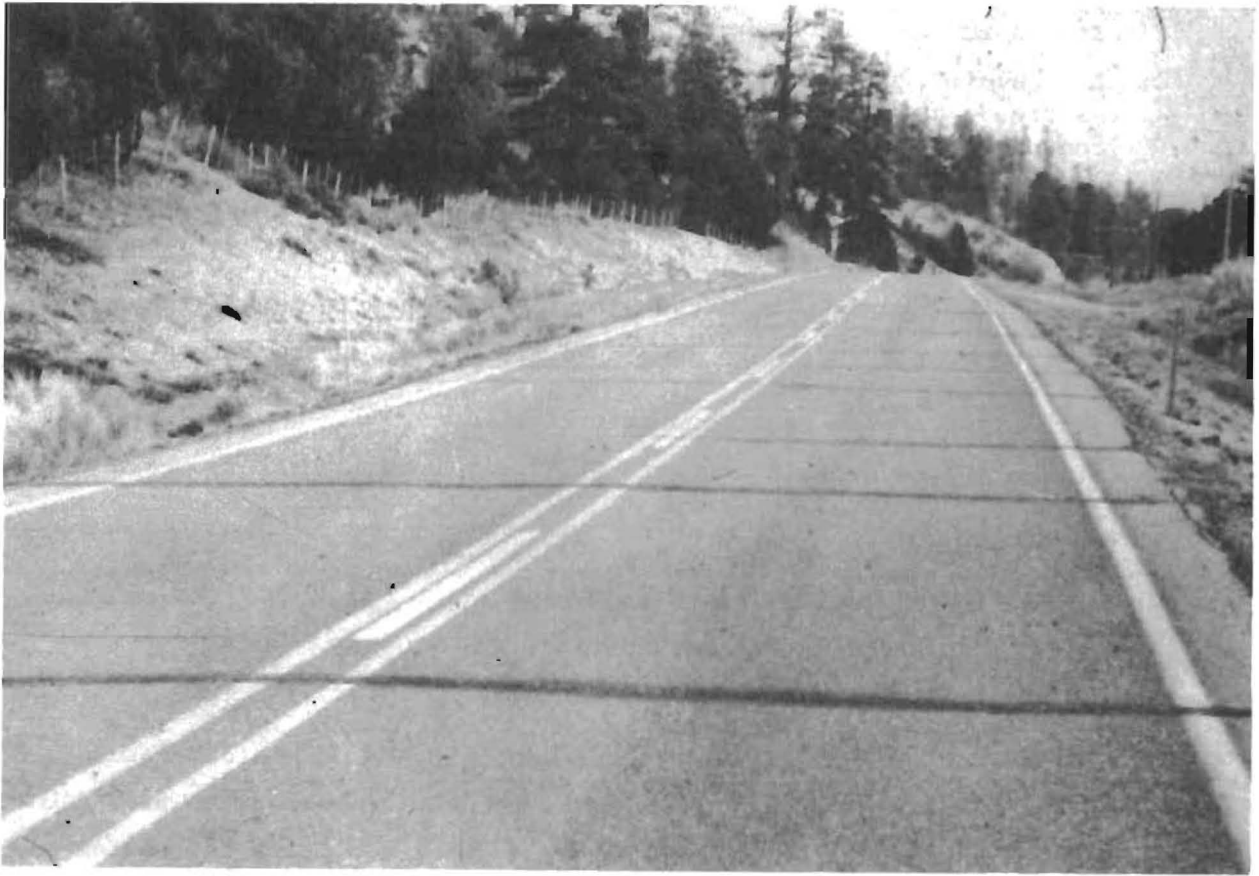
Fig 1.1. Temperature cracking in Southern Utah highways.
