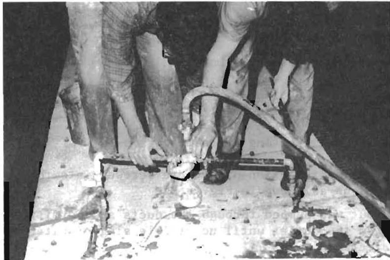
Fig. 6.22. Connection of injection pipes and inlets of tendons
