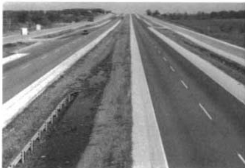
(a) Looking north at section 9. Patch in left background is just beyond limits of section 9.
