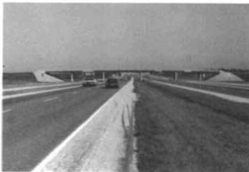
(b) Looking north, excellent condition of overlay and sealcoat in southbound main lane is shown.
