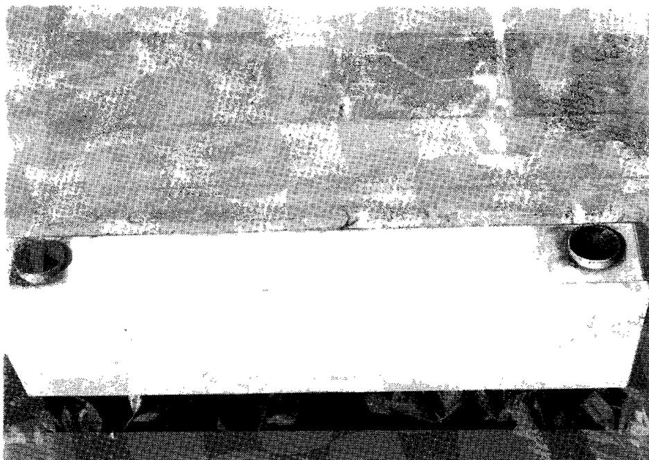
**Fig A.1. Metal box housing two Opcon infrared sensors, HOV lane in Houston.**
