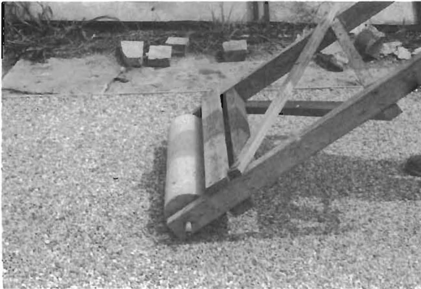
Fig. 5.4. Compacting with 6-in. Diameter Concrete Cylinder.
