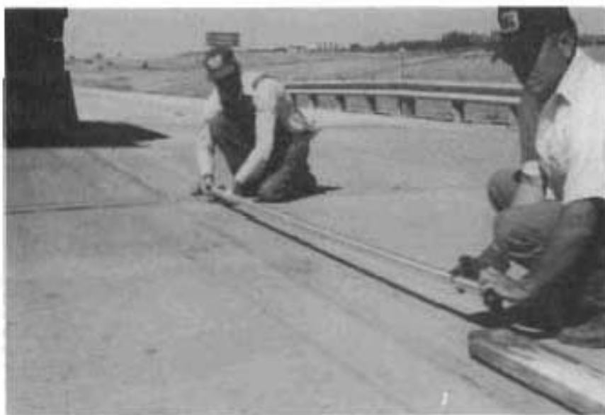
Fig. 5.13. Bonding Wood Strip to the Deck.
