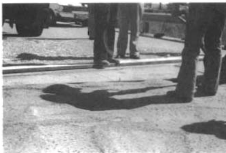
Fig. 5.16. Screeding the Sand to 1/4-in. Thickness.
