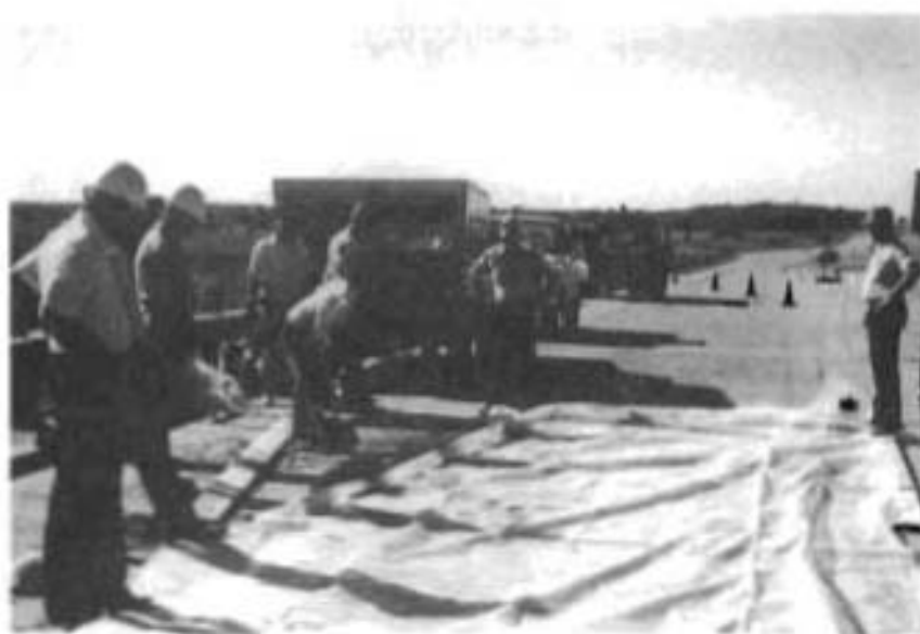
Fig. 5.21. PC Overlay Covered with Polyethylene Film While Soaking and Curing.
