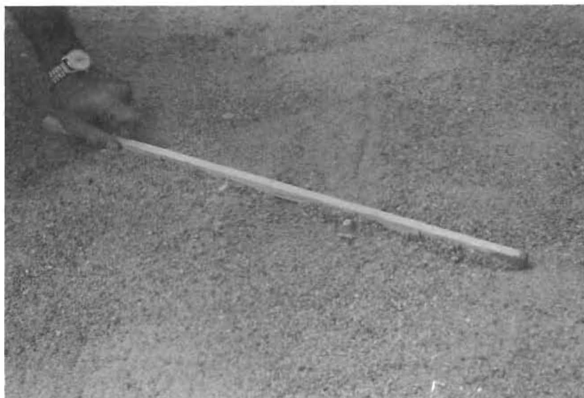
Fig. 5.1. Screeding Sand to 1/4-in. Thick.
