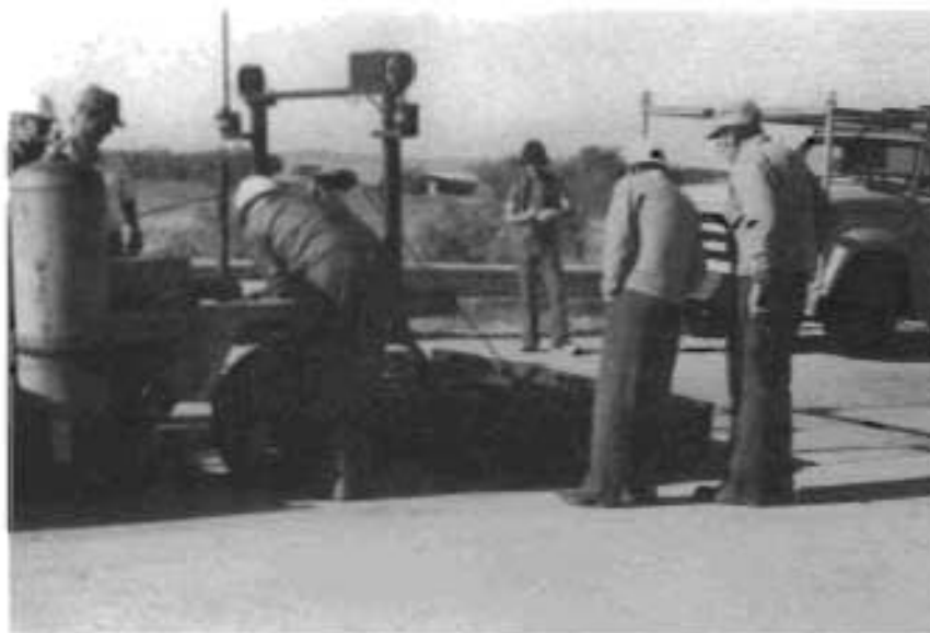
Fig. 5.10. Concrete Deck Dried by Blackwall Infra-Red Asphalt Patcher IR-96.
