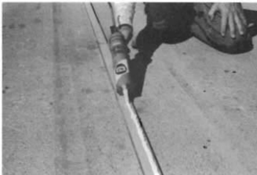
Fig. 5.12. 1/2 in. Thick Wood Strip Caulked with Latex.
