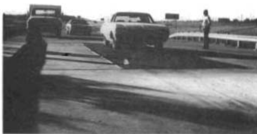
Fig. 5.22. Open to Traffic After 2-1/2 Hours.
