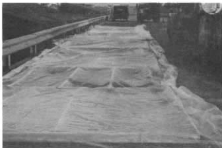
Fig. 5.24. Wood-Framed Polyethylene Film Cover.
