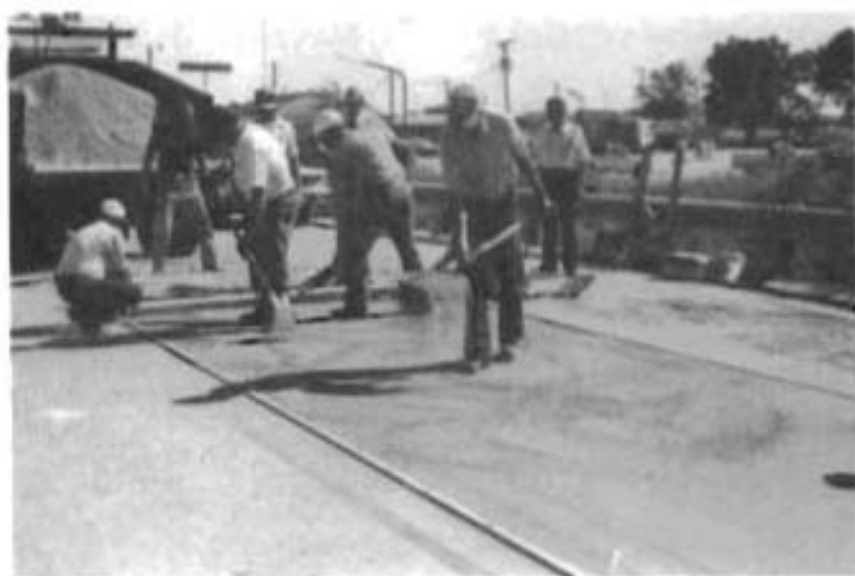
Fig. 5.15. Spreading the Concrete Sand.
