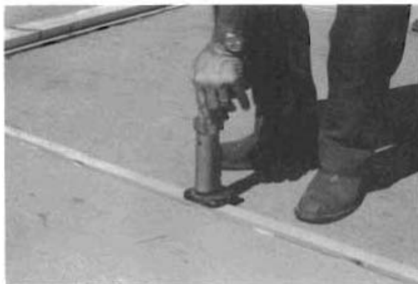
Fig. 5.14. Nailing the Wood Strip.
