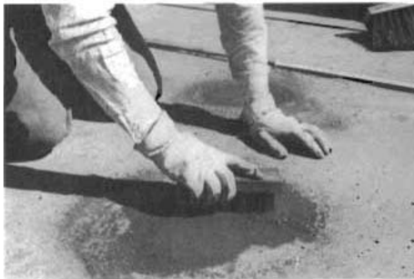
Fig. 5.9. Surface Contamination Cleaned Off.
