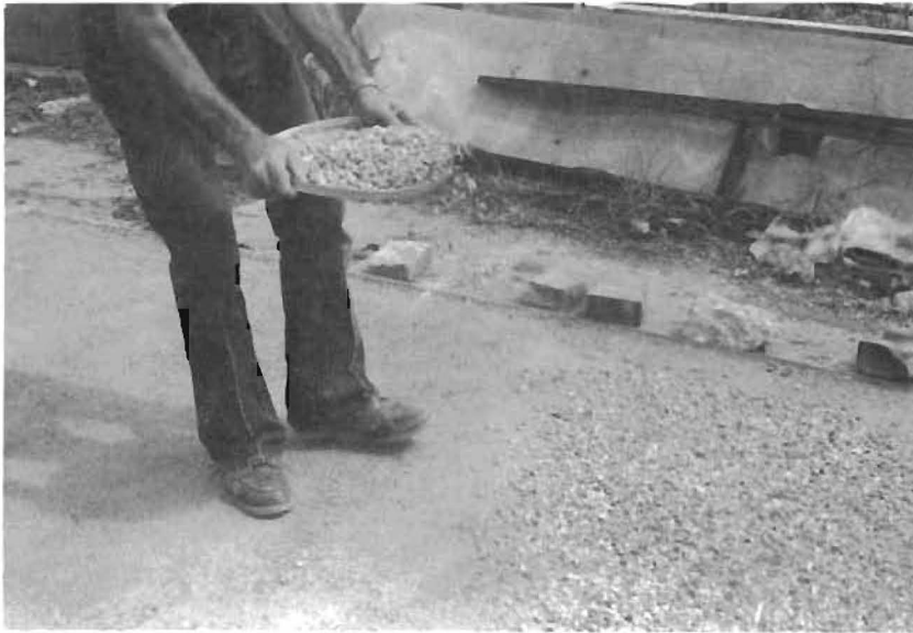
Fig. 5.3. Applying 1.8 psf of Pea Gravel to the Top of Sand.
