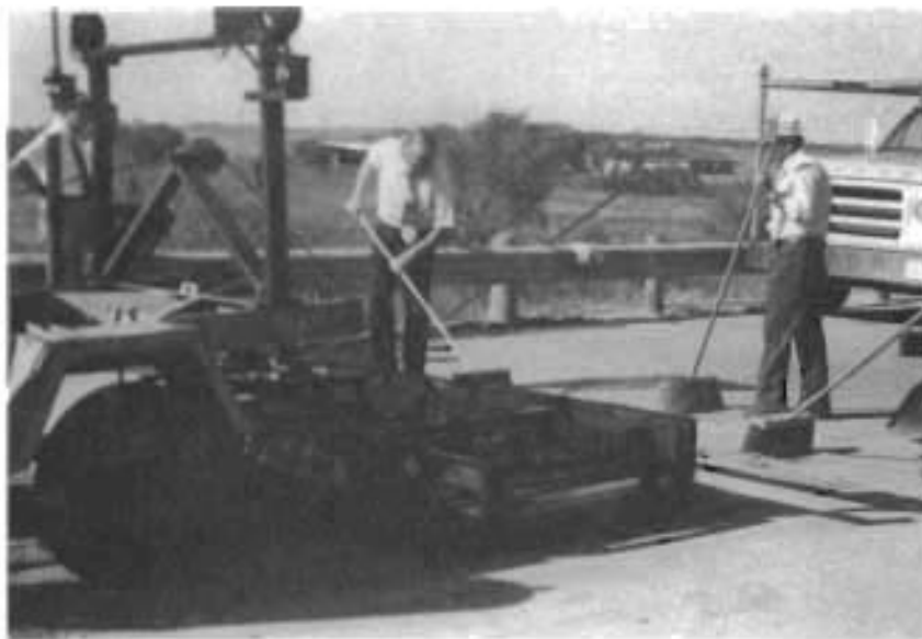
Fig. 5.11. Concrete Sand Dried by Blackwall Infra-Red Asphalt Patches IR-96
