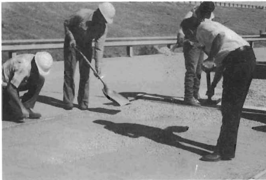
Fig. 5.17. Spreading the Coarse Aggregate.
