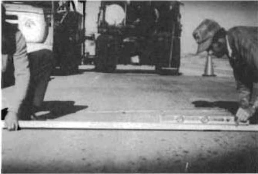
Fig. 5.7. Transverse Slope of 1/8-in. per ft.
