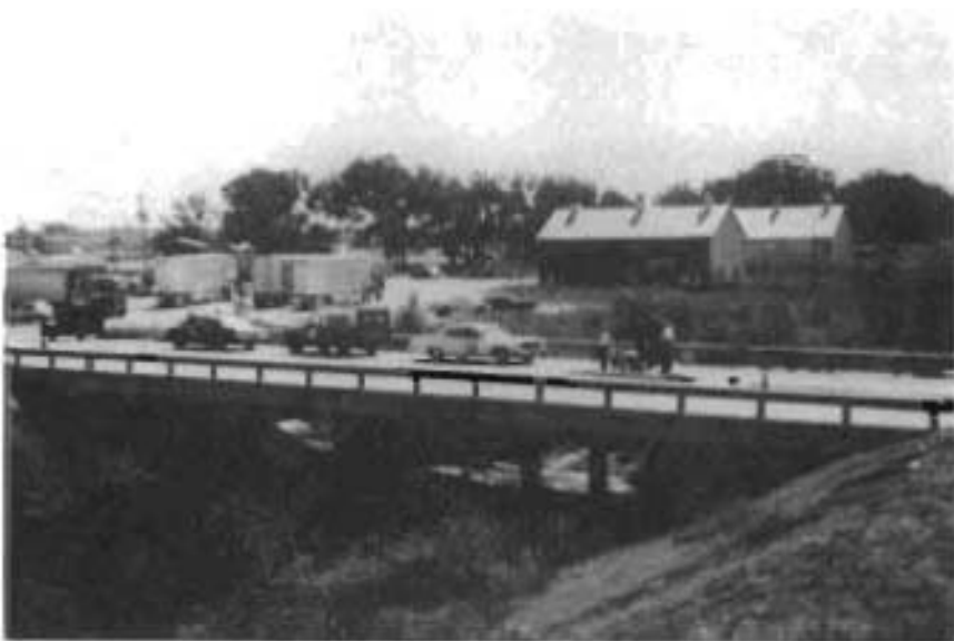
Fig. 5.8. A View of the Bridge from U.S. 287.
