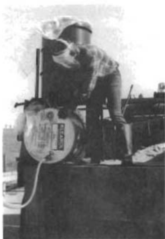
Fig. 5.20. Monomer Mixed in 55-gal. Drums Loaded on a Truck (Appendix).
