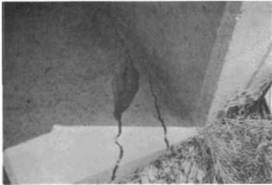
a) Cracking on the West Side
