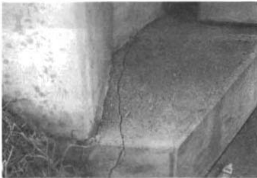
b) Cracking on the East Side
