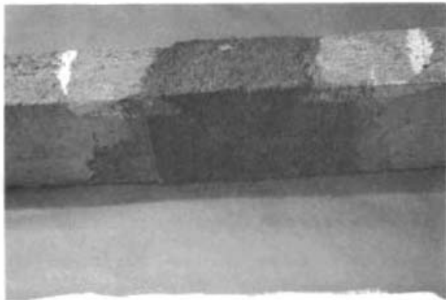
FIG. 4.4 TYPICAL BEAM AFTER REPAIR
