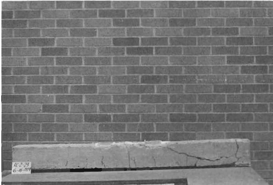
a) Original Failure Mode
