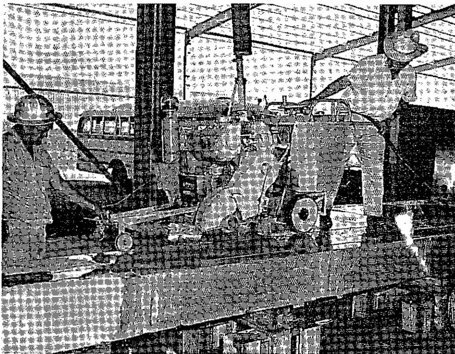
Fig. 5. Sawing out strips cutting across cracks.
