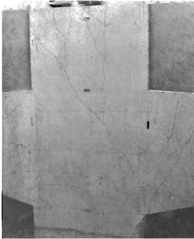
Fig. 8(a). Cracking pattern at the junction of the pylon and crossbeam.
