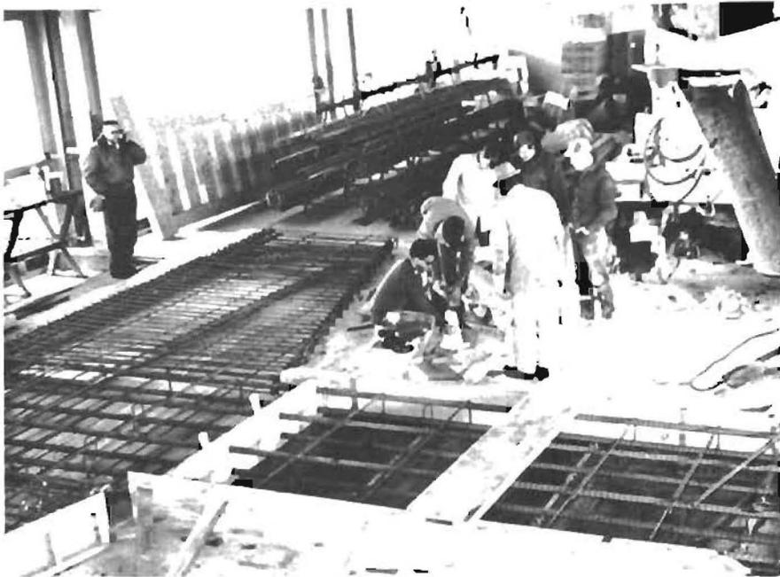
Fig. 3. Reinforcement of test specimen in place.
