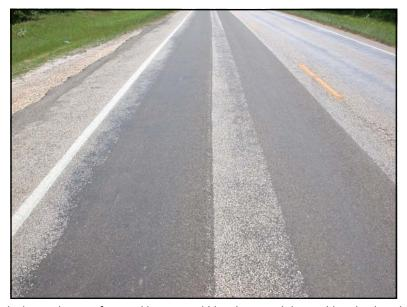
This treatment method seals the roadway surface and improves skid resistance. It is considered to be a long term solution to bleeding.
