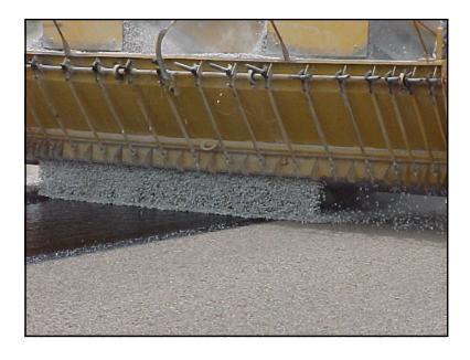
is typically around 140°F to 165°F whereas the original application temperatures for hot asphalts range from 300°F to 350°F.
