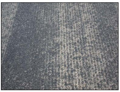
chine. The hot aggregate is rolled in using a steel wheel roller.
