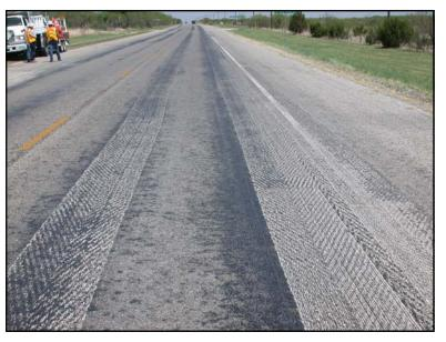
Certain seal coat materials have a tendency to gum up the milling machine in hot weather, especially the crumb rubber seal.
