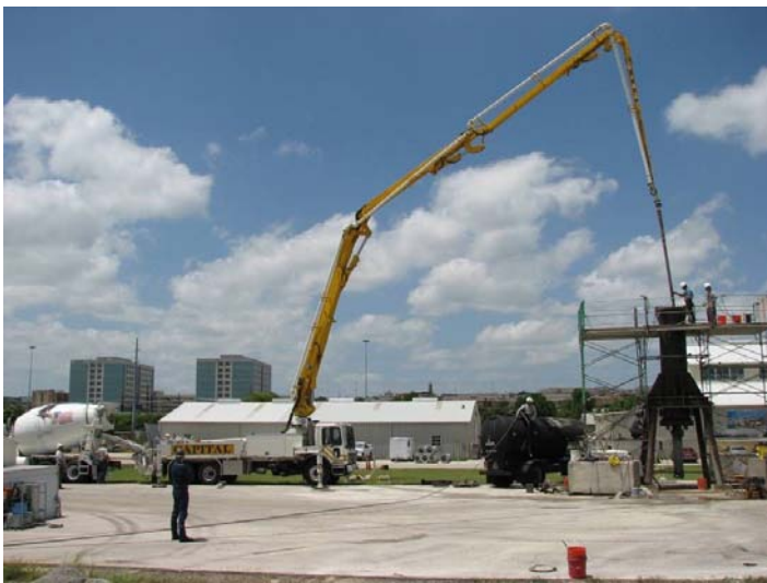
Acquisition of verification core
