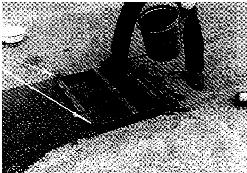
Figure 1. Mixture being placed with a lab prototype of the laydown machine
