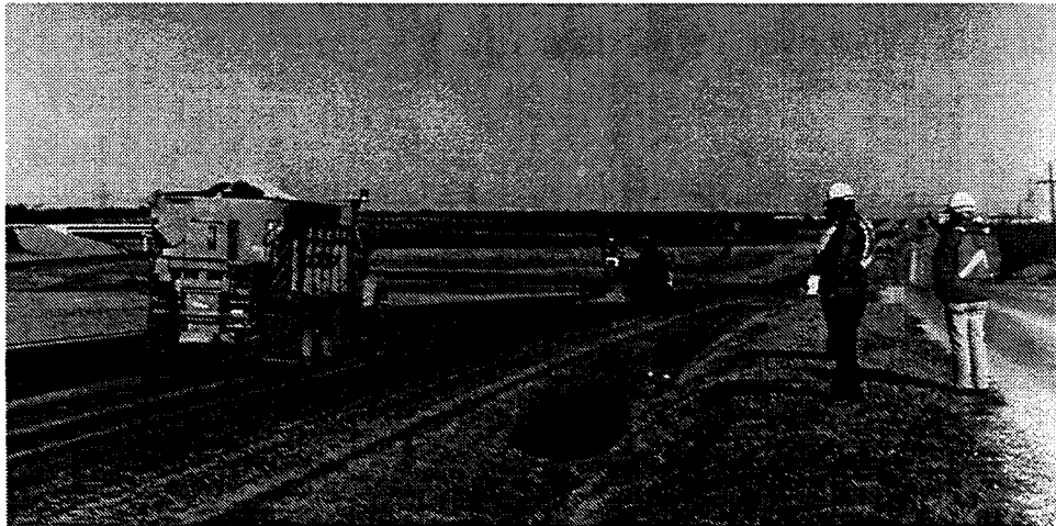
Figure 4. Emulsion being placed and aggregate spreader following the asphalt distributor
