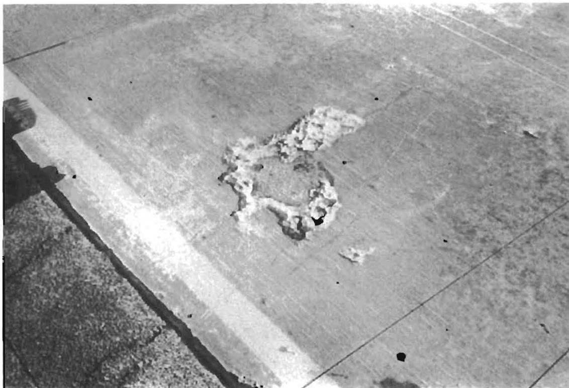
Fig 6. Repair area showing punchout
