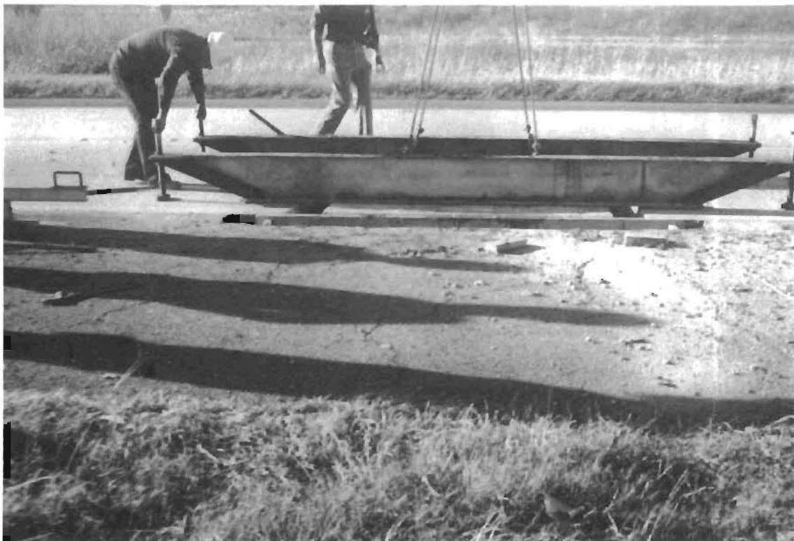
Fig 10. Precast repair showing leveling beams.
