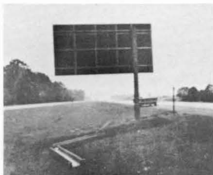
Figure D-9. Effectiveness of the break-away post is shown by crash test, above, and by roadside sign after test by an obliging—but probably disconcerted—motorist.
