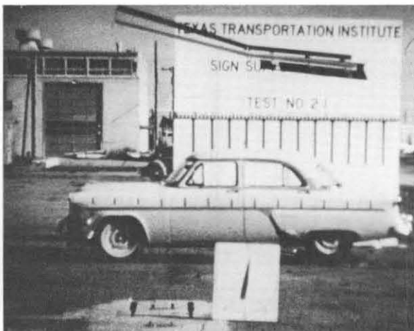
(c) 2-3I5.7 STEEL SUPPORTS INCLINED BASE 25 MPH
