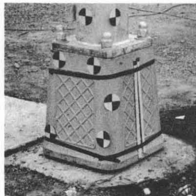
STEEL POLE - ALUMINUM TRANSFORMER BASE
