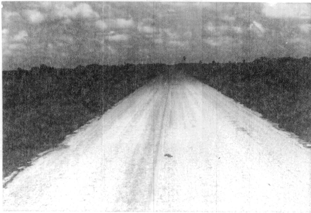
Photo 24 Day Appearance of FHWA Code 52 Traffic Paint on ACP After Eight Months Exposure
