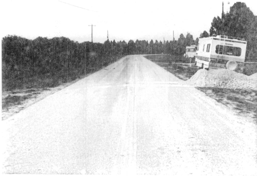
Photo 28 Day Appearance of 50/50 Mix Traffic Paint on ACP After Eight Months Exposure
