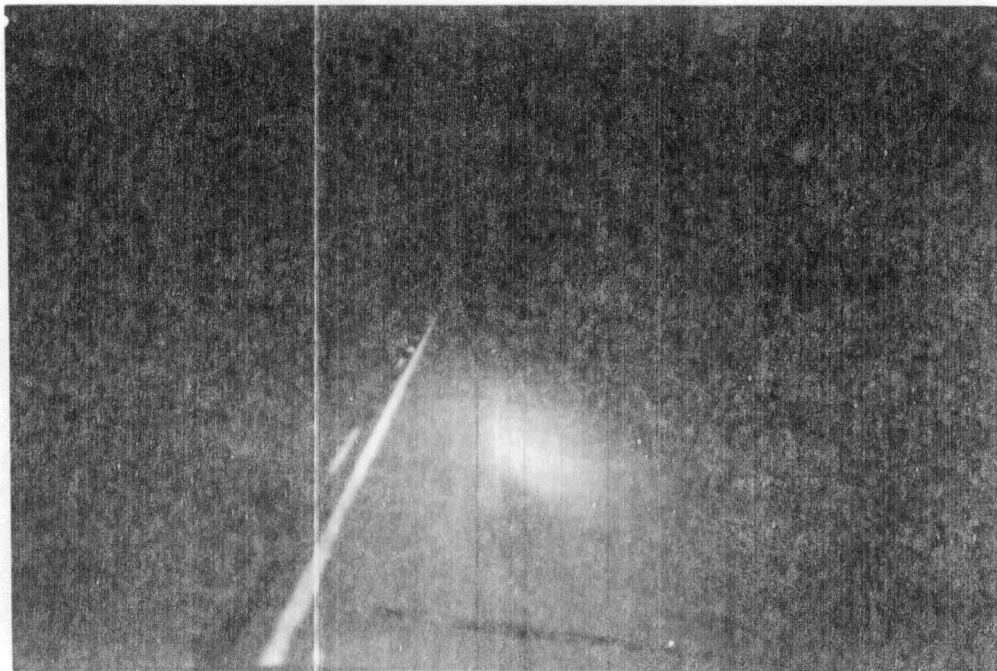
Photo 35 Night Appearance of Texas Specification Traffic Paint on PCCP After Eight Months Exposure
