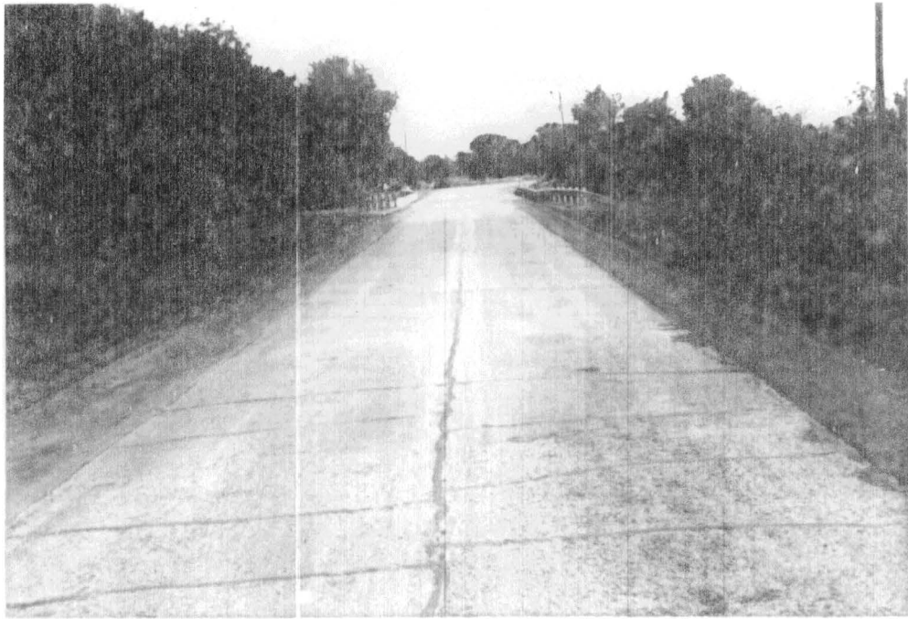
Photo 22 Day Appearance of FHWA Code 49 Traffic Paint on PCCP After Eight Months Exposure
