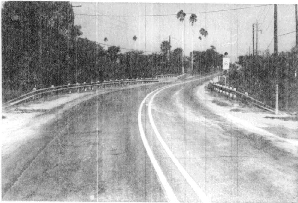
Photo 37 Day Appearance of Restripe With FHWA Code 49 Traffic Paint on PCCP
