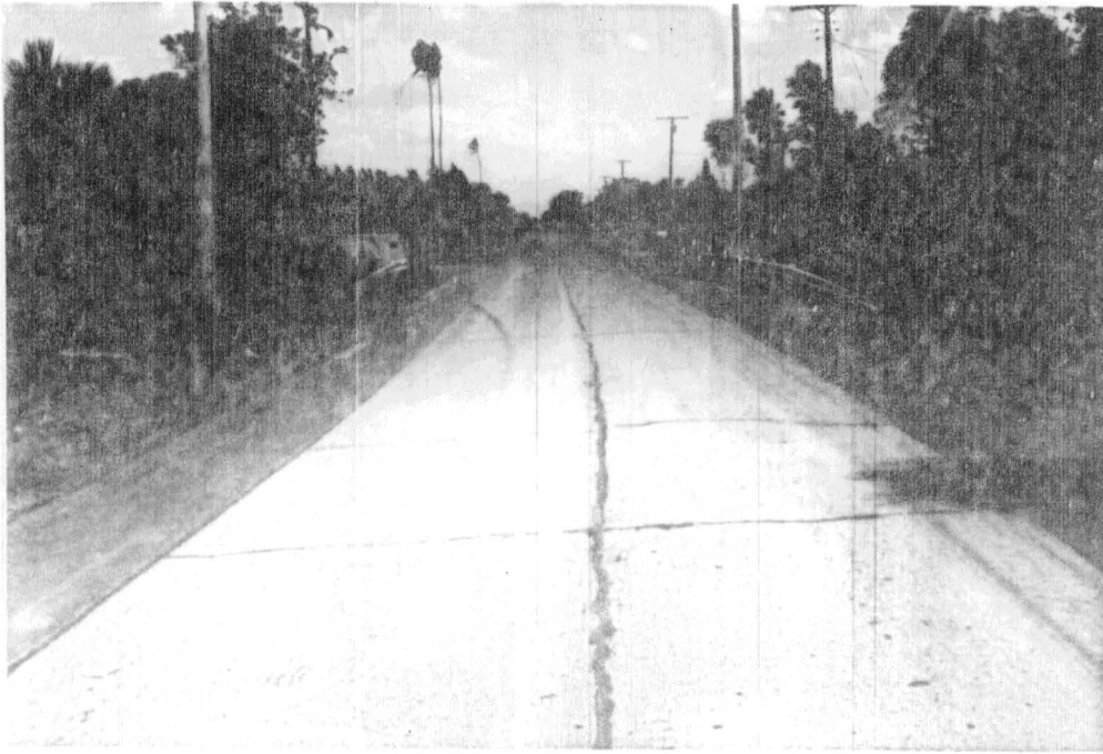
Photo 26 Day Appearance of FHWA Code 52 Traffic Paint on PCCP After Eight Months Exposure
