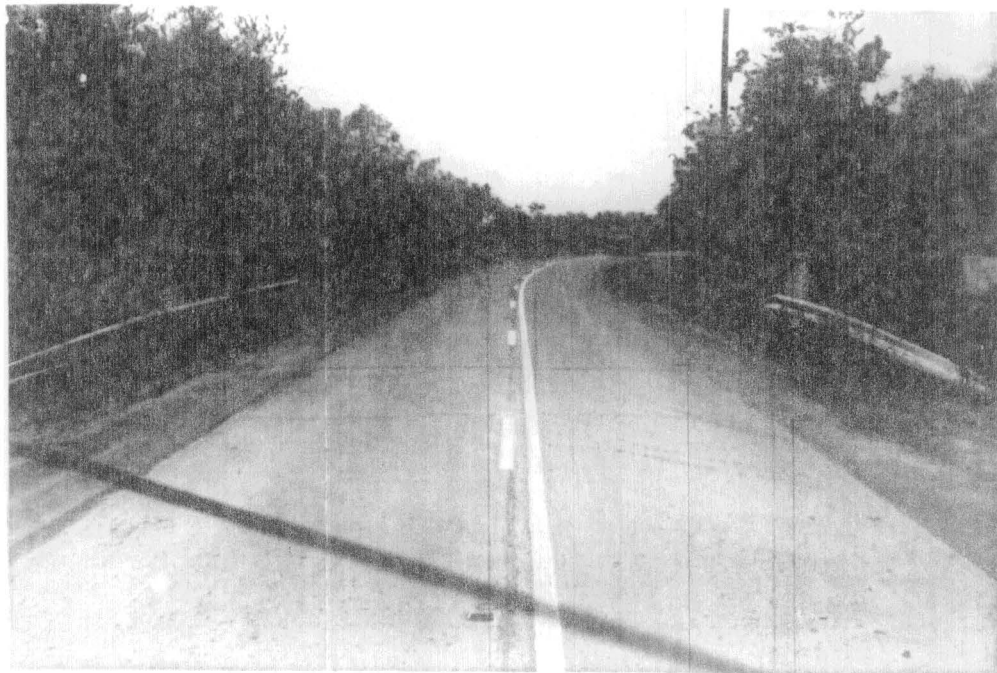
Photo 39 Day Appearance of Restripe With FHWA Code 52 Traffic Paint on PCCP
