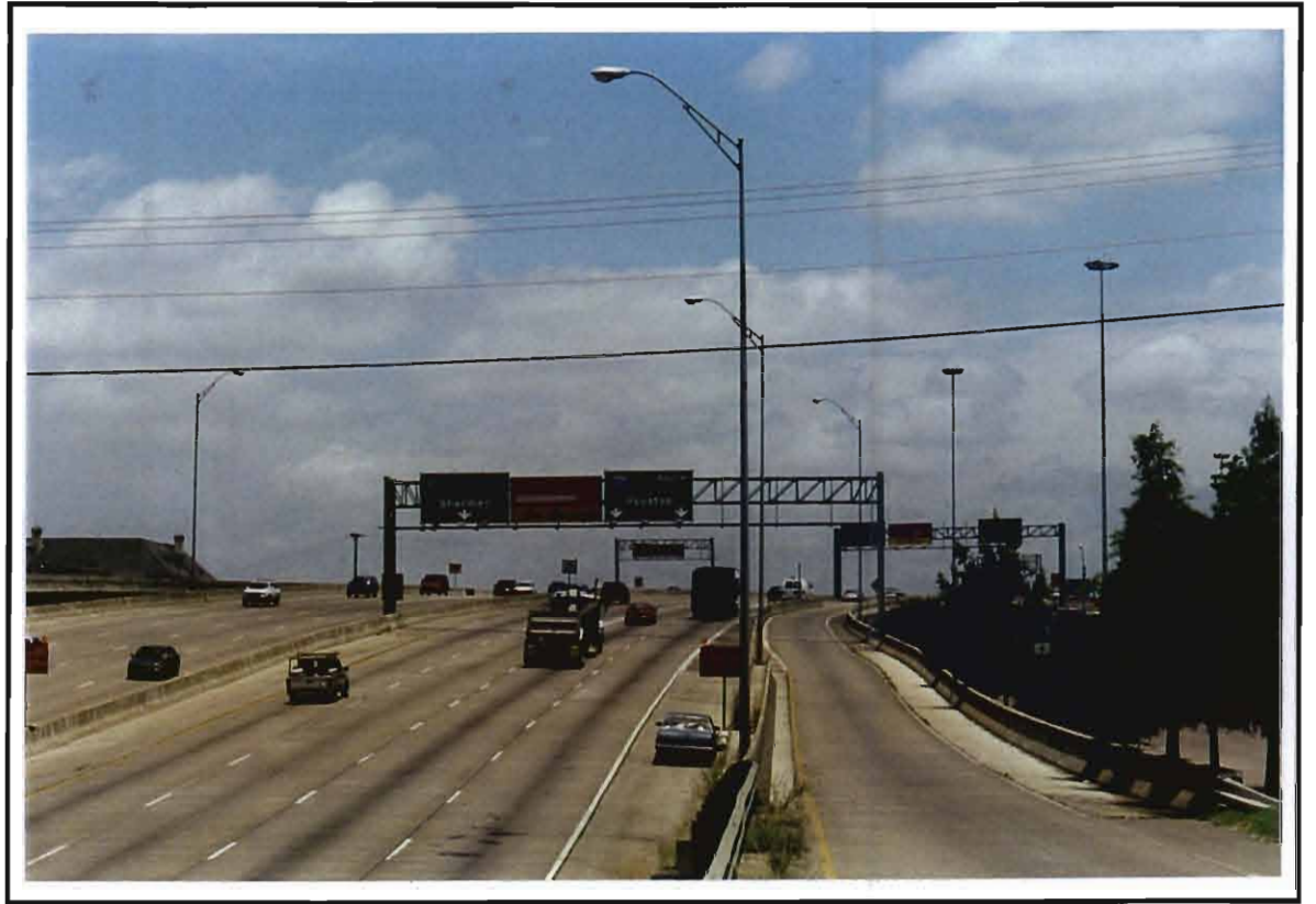
Photo 8. View of guide signs above Woodall Rodgers Freeway (view from Pearl Street entrance ramp).
