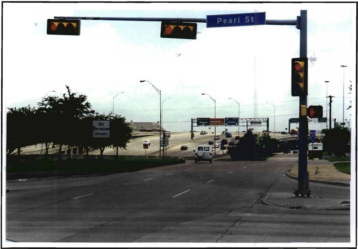
Photo 5. Existing road signs on the frontage road of Woodall Rodgers Freeway (before Pearl Street entrance ramp).
