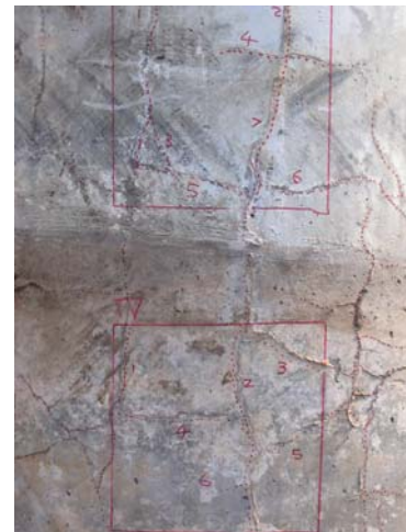
Figure 3.3 HMIP Foundation with Premature Concrete Cracking
