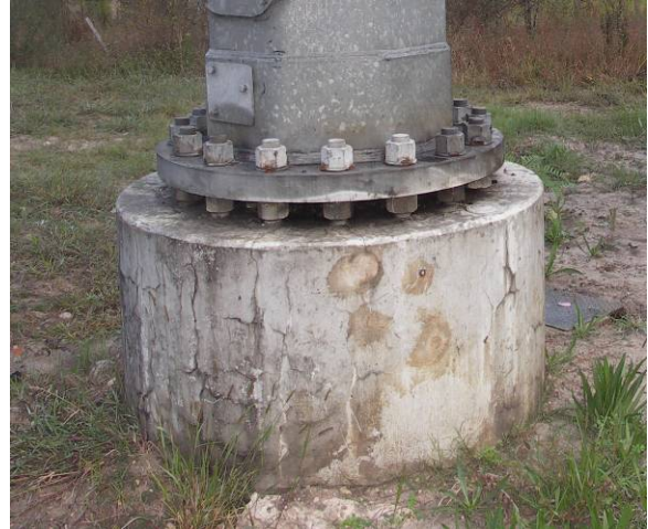
Figure 1.3 ASR/DEF Damage in Drilled Shafts
