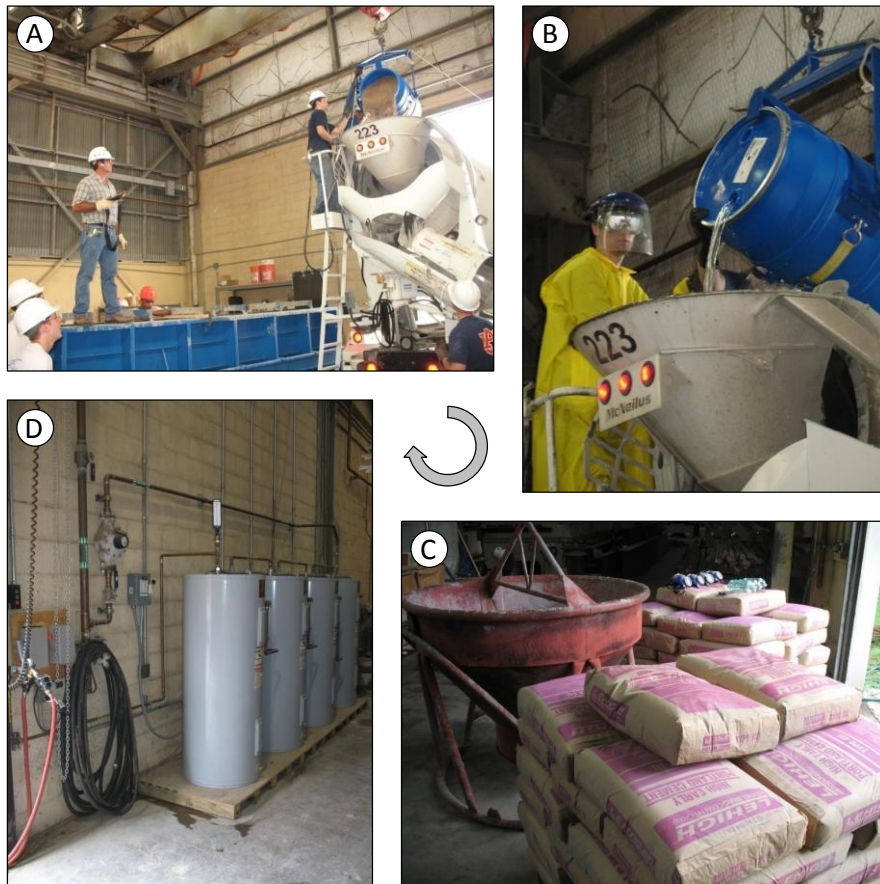
Figure 3-15: Concrete Materials Batching
