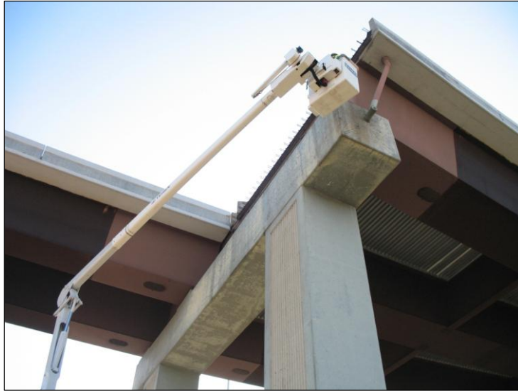
Figure 6-5: Bent 15 Inspection with Aerial Lift
