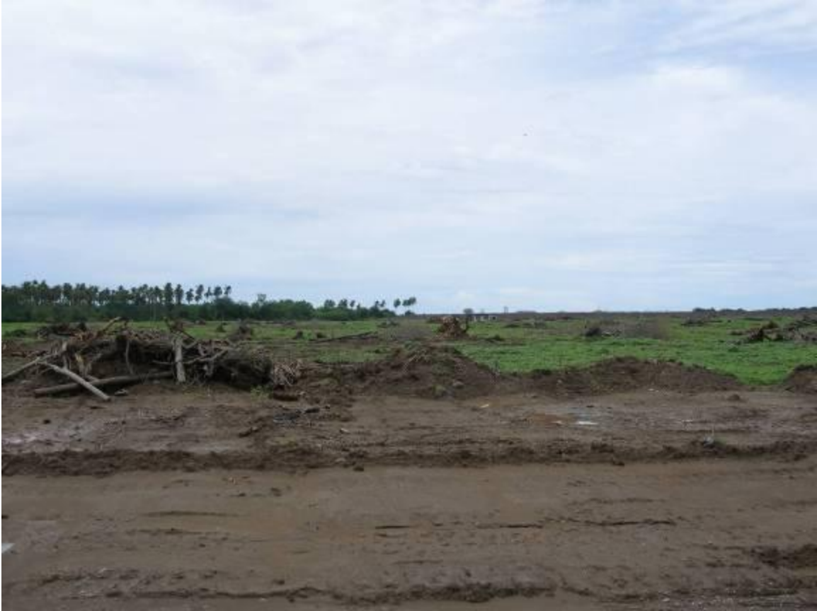
Figure 6. Site of Future Container Terminal in July 2005
