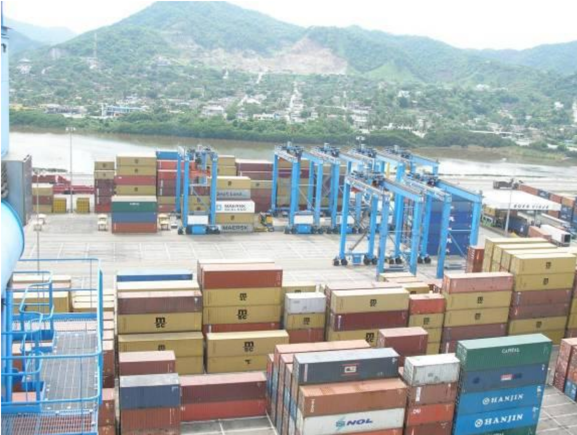
Figure 8. Manzanillo Main Container Yard
