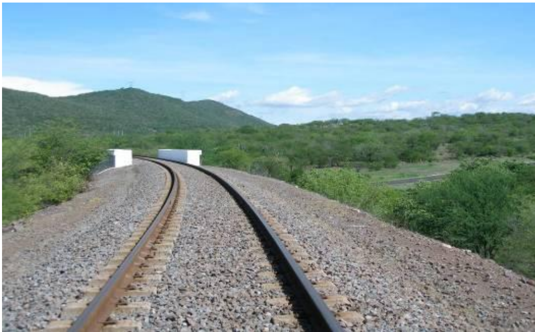
Figure 5. Grade-separated Rail Crossing near Lazaro Cardenas, July 17, 2005
