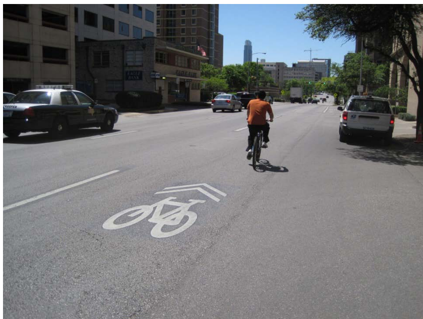
Figure B4. Central placement of sharrow resulted in thriving thermoplastic five months after installation.
