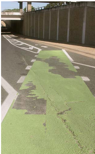
Figure B1. Deteriorating thermoplastic on one of the I-35 exit ramps (breaking up in sheets)
