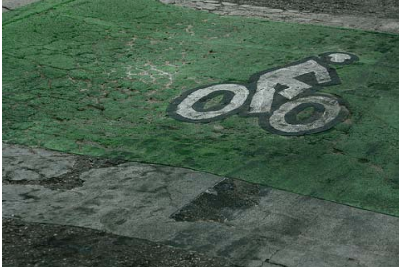
Figure B2. Poor quality of road lead to the deterioration of the thermoplastic bike boxes on Speedway Boulevard
