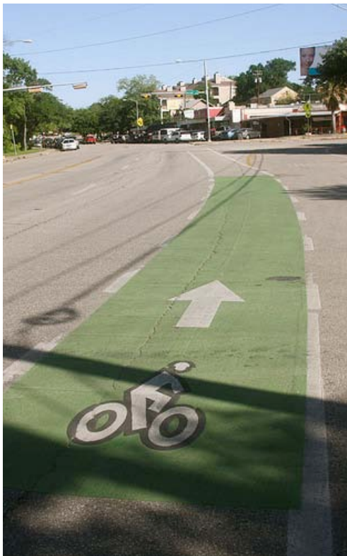
Figure 9. The colored lane installed on San Jacinto Boulevard
