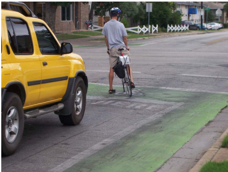
Figure B3. Poor quality of road lead to the deterioration of the thermoplastic bike boxes on Speedway Boulevard
