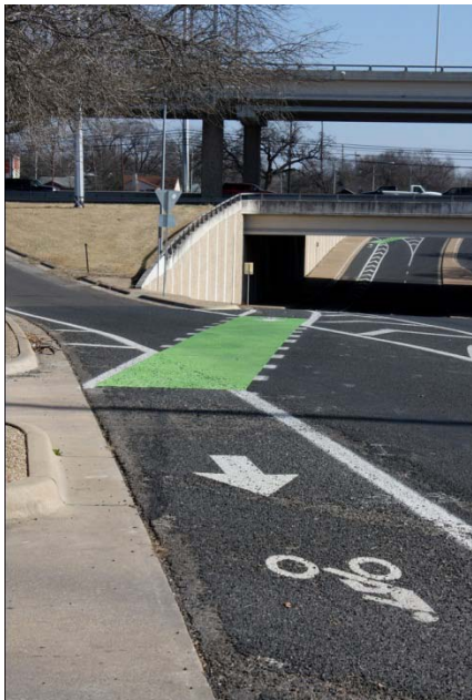
Figure 1. A colored bicycle lane in Austin emphasizes the conflict zone between the bicycle lane and the highway exit ramp
