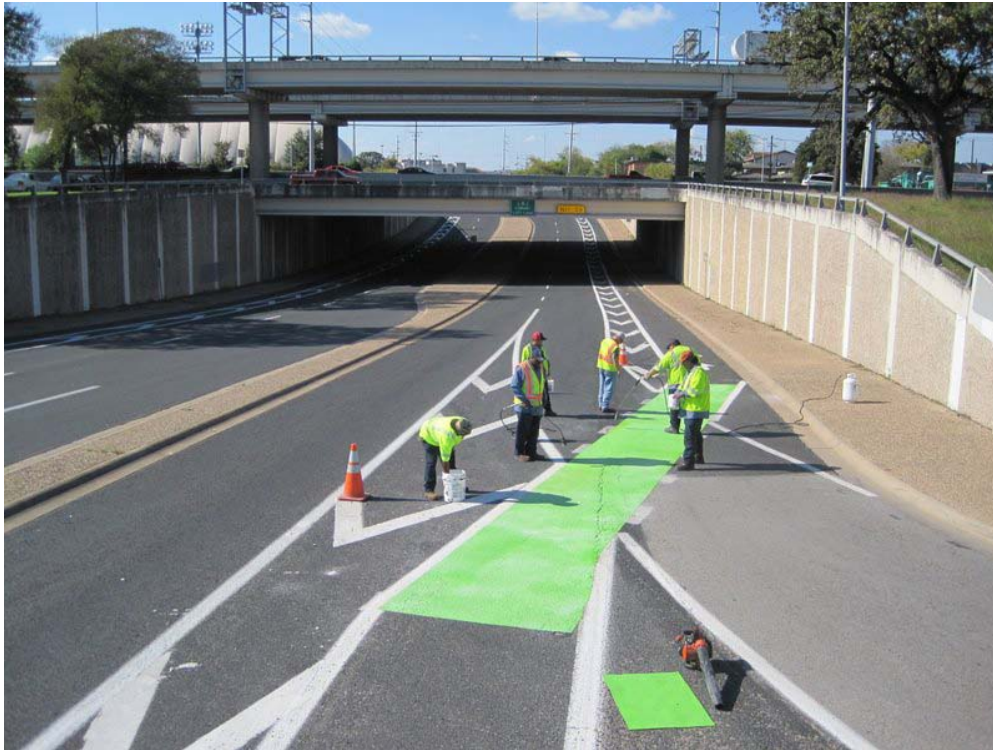
Figure 2. Thermoplastic colored lane during installation on Dean Keeton Street
