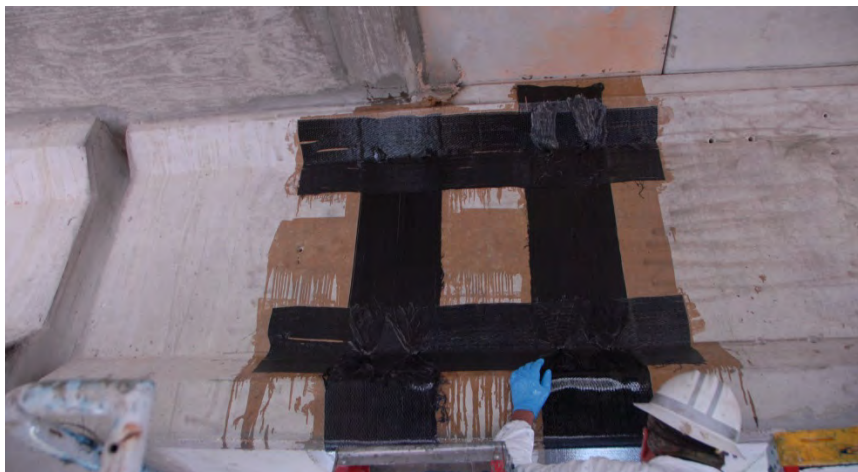
Figure 11: Installation of anchors
