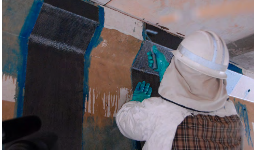
Figure 17: Saturation of dry sheet with epoxy
