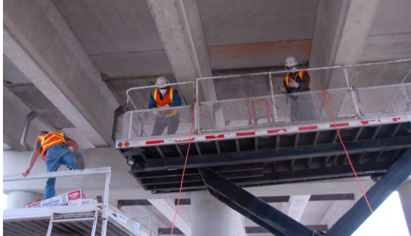
Figure 5: Work platform in position
