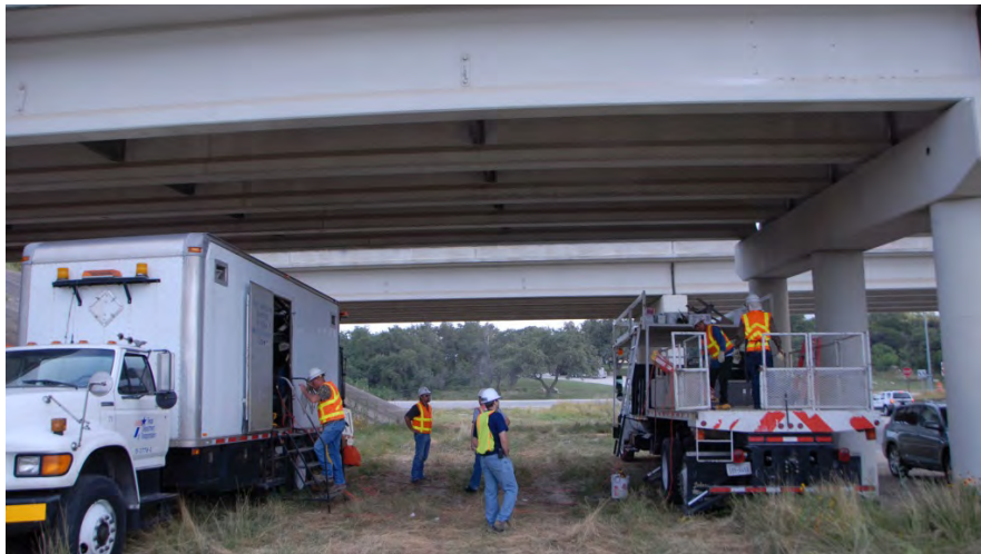
Figure 4: Maintenance vehicles in position
