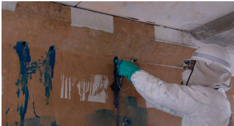
Figure 15: Application of epoxy to concrete surface and anchor holes
