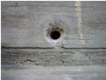
Final clean hole
