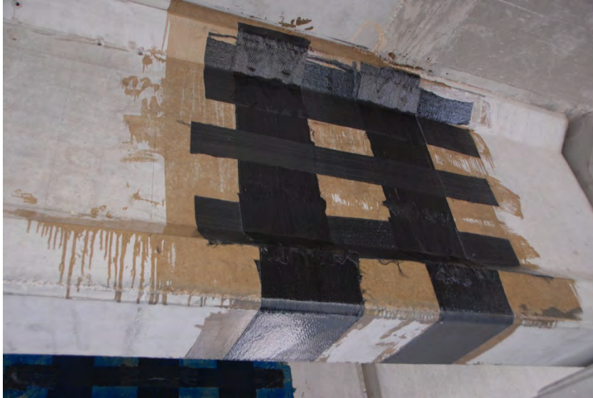
Figure 12: Completed wet layup installation
