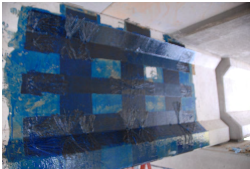
Figure 19: Completed dry layup installation
