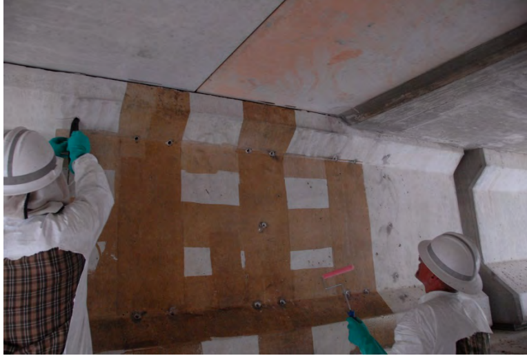
Figure 14: Application of primer epoxy coat
