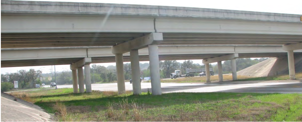
Figure 1: View of bridge selected for trial installation
