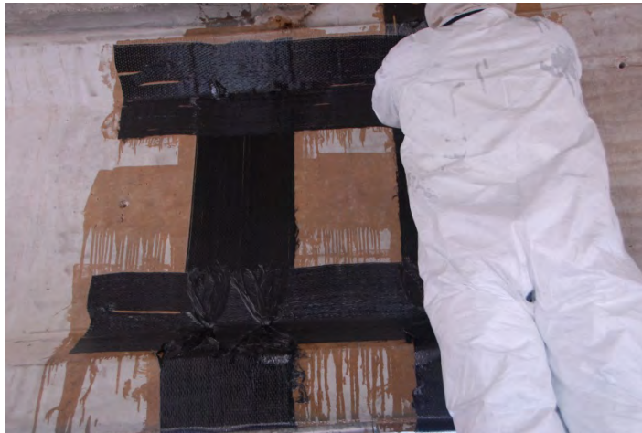
Figure 10: Application of epoxy to concrete surface, including holes, and placement of saturated sheets
