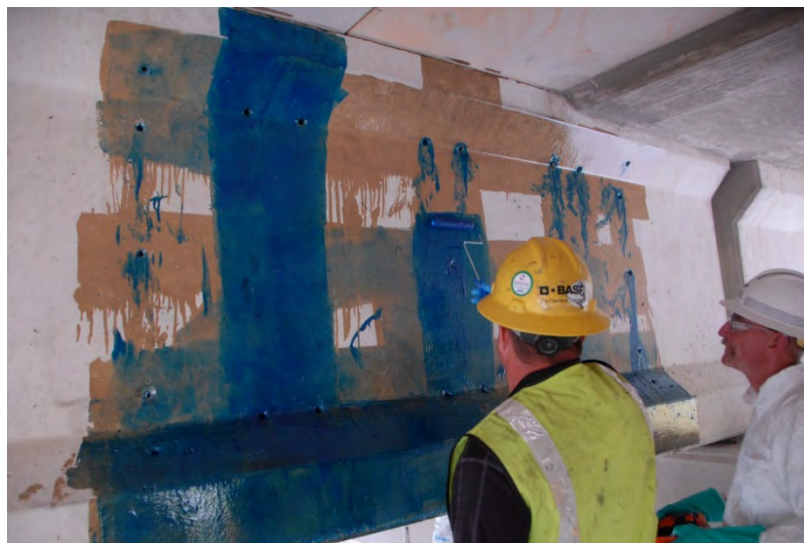
Figure 16: Installation of dry CFRP sheets on epoxy coated surface
