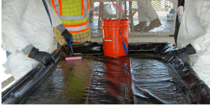
Figure 9: Saturation of CFRP sheets with epoxy (wet layup)
