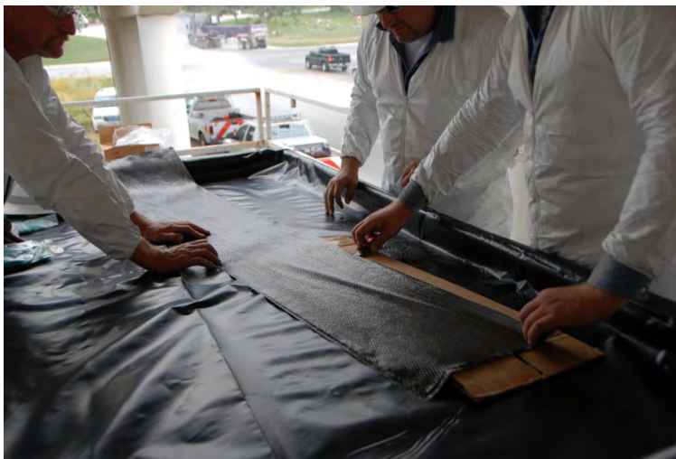
Figure 13: Preparation of CFRP sheets (dry layup)
