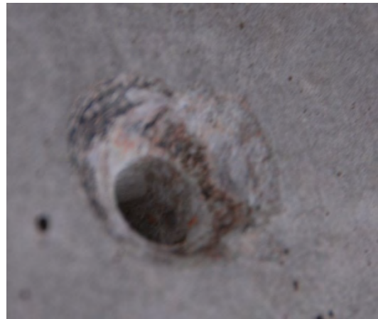
Figure 7: Hole with rounded edge for anchor
