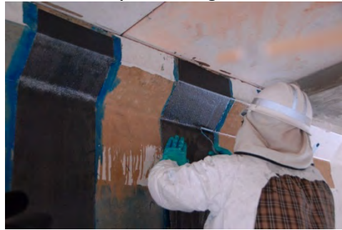
Step b on an I-girder
