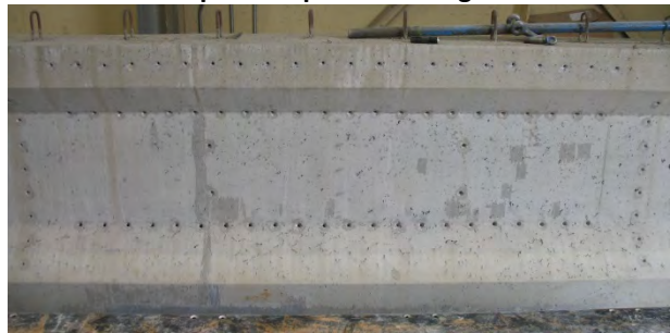
Sample hole pattern for I-girder
