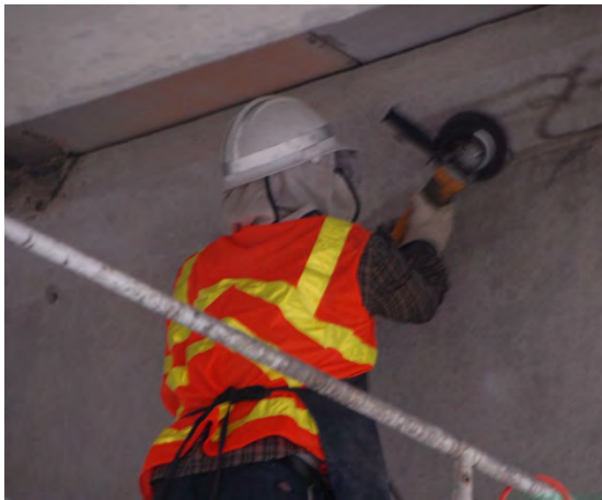
Figure 6: Preparation of concrete surface
