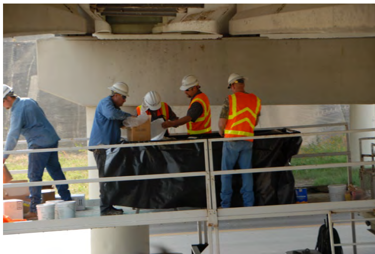
Figure 8: Work area for preparation of CFRP sheets
