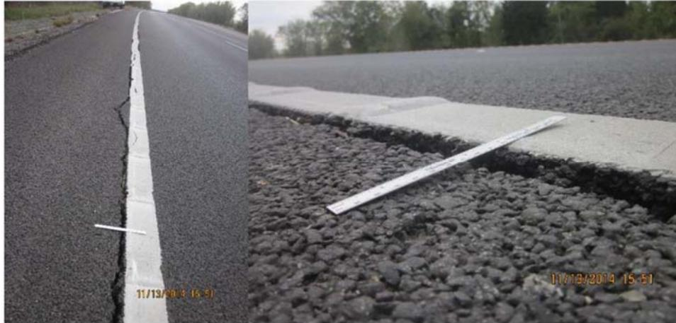
Figure 4.132: Edge Cracking at SH-21 (Garcia 2015)
