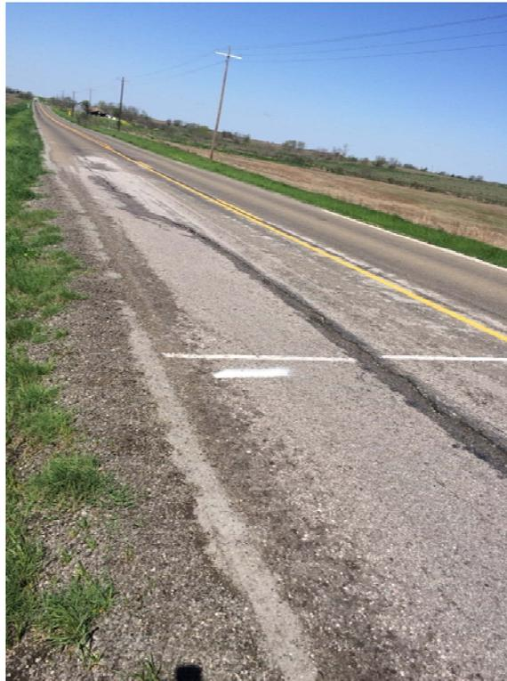
*Figure 5.55: Longitudinal Crack at FM 972*
