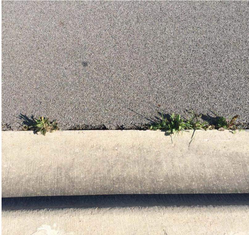
*Figure 4.94: Gap between Curb and Asphalt at Site 6*
