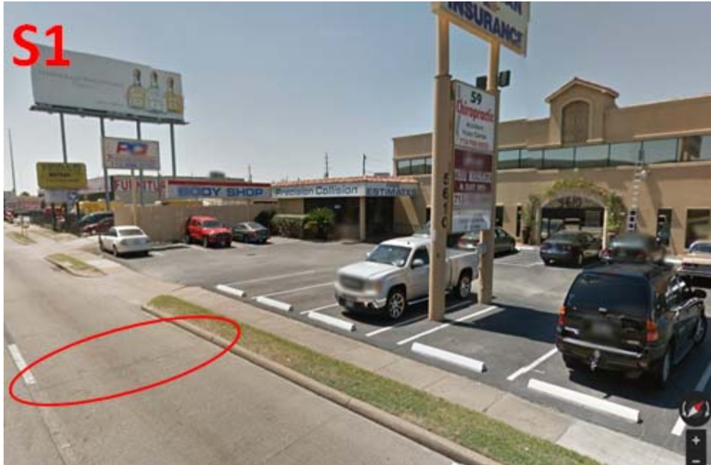
Figure 2.17: One Joint with High Deflection Scheduled for a Saw and Seal Operation
