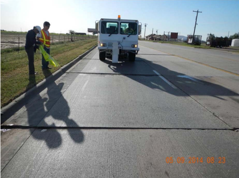
Figure 2.26: Transverse Joints Showing Faulting on Westbound Lane of US 287 in Quanah, TX
