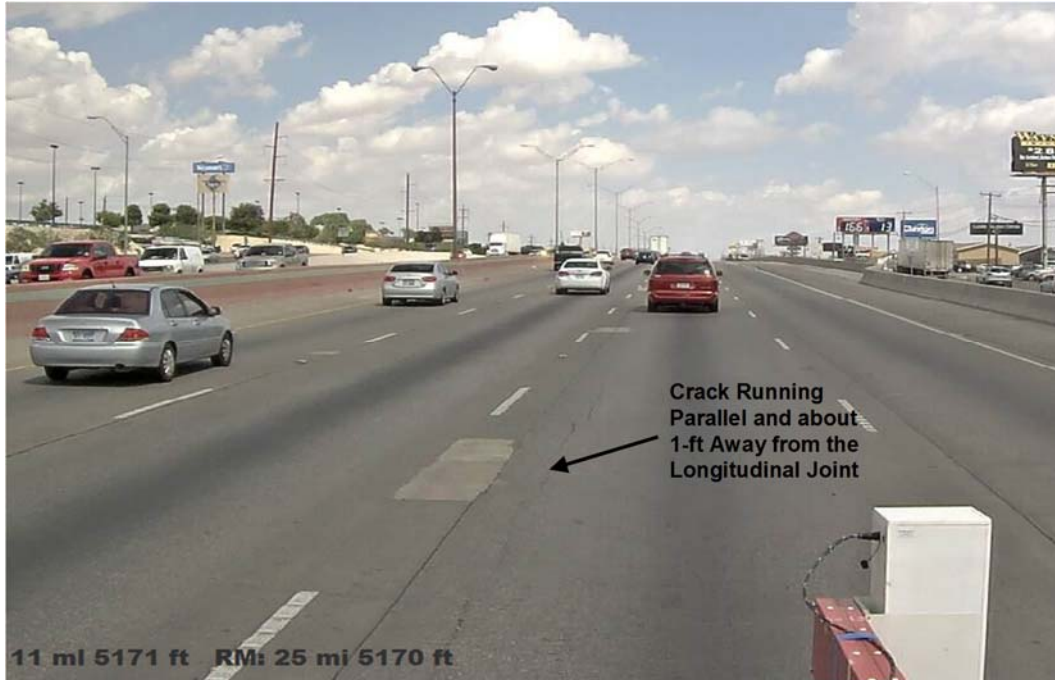
Figure 2.11: Distressed and Repaired Areas on IH 10 from TRMs 25.5 to 27
