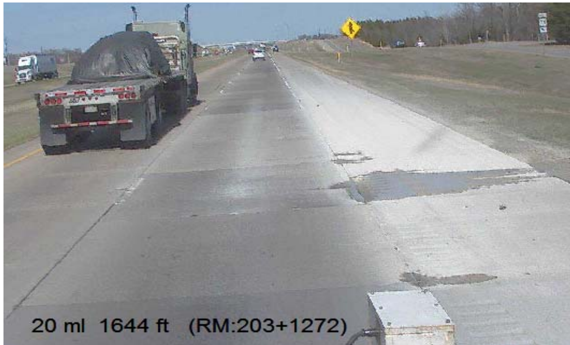
Figure 2.8: Badly Distressed Section of US 75 Just North of Sherman, TX
