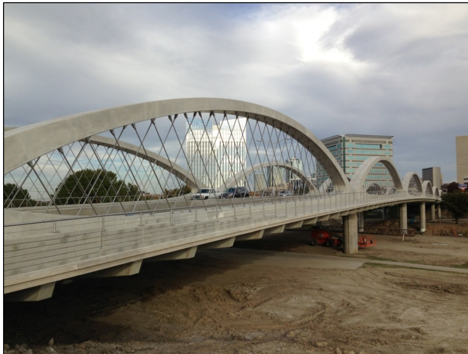
Figure 1.2- The new West 7 th Street Bridge.
