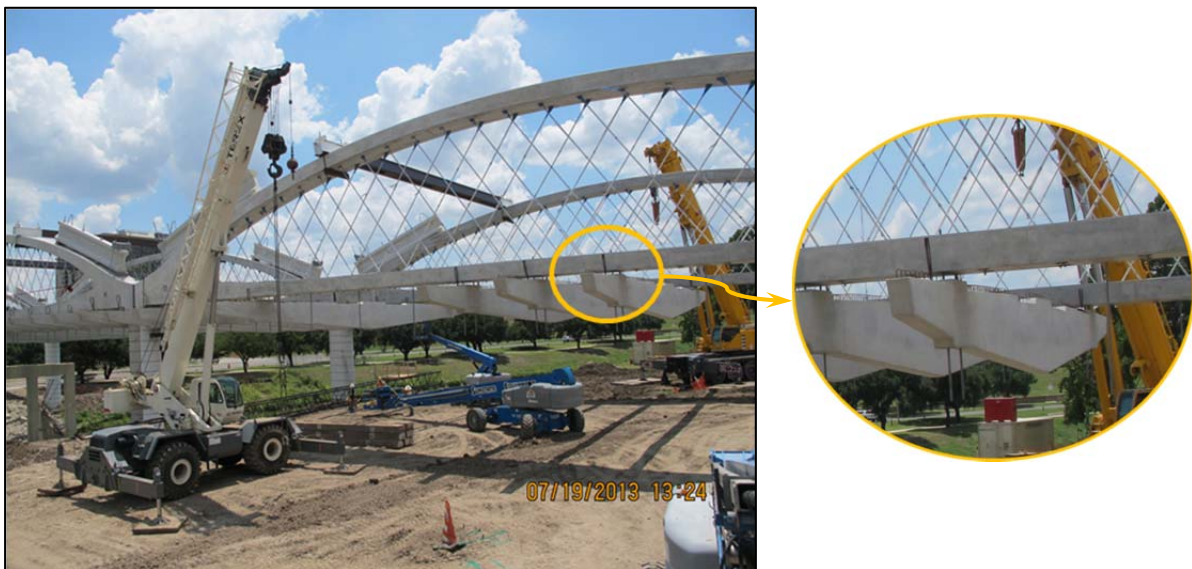
Figure 2.18- Initial hanging of the floor beams.
