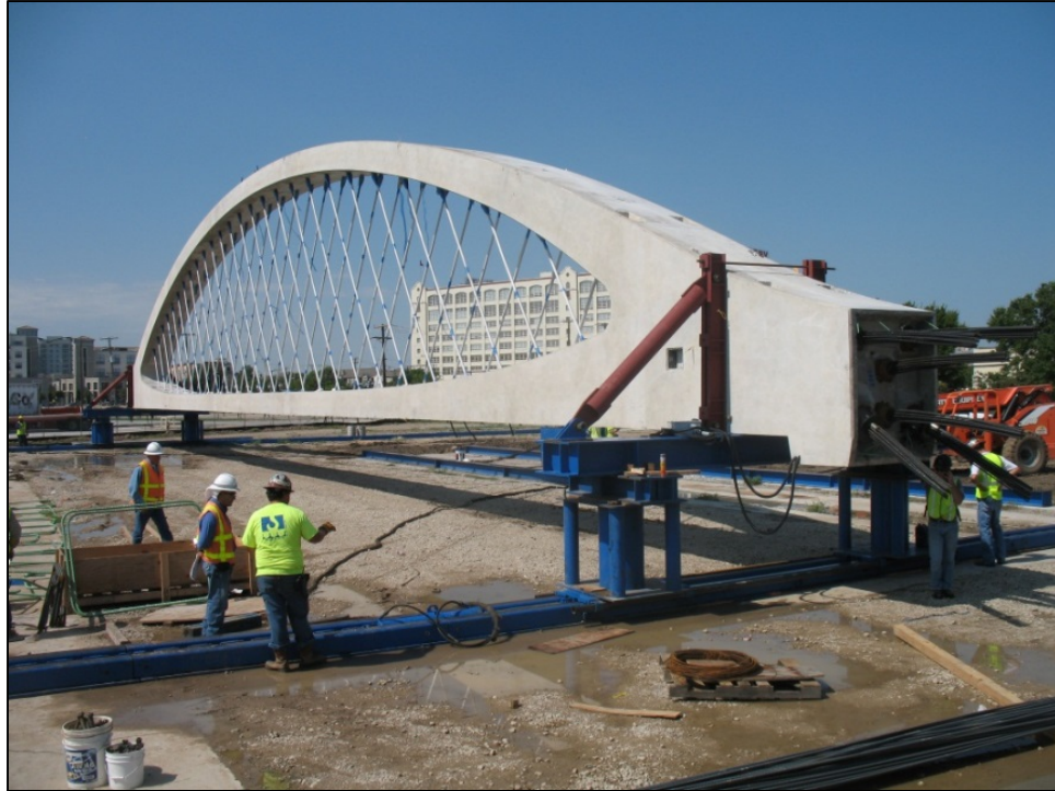
Figure 2.13- Sliding operation on one of the arches.
