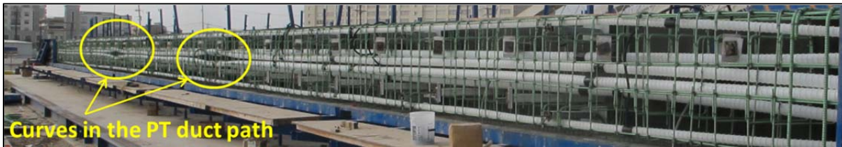
Figure 2.12- Intentional curves in the duct paths.
