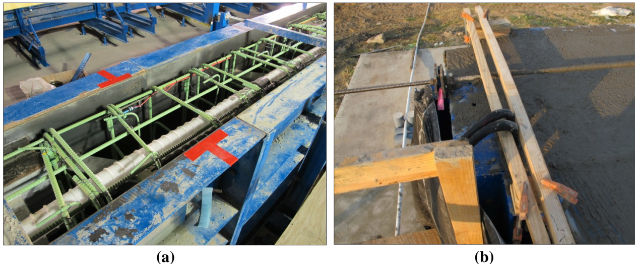
Figure 4.13- VWG installation process (continued). (a) Labeling the locations of the VWGs on the formwork. (b) Fixing the gauge cables at the exit location.
