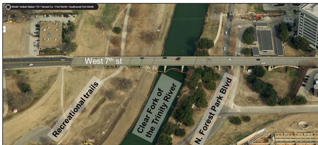
Figure 1.1- The location of the West 7 th Street Bridge [1].
