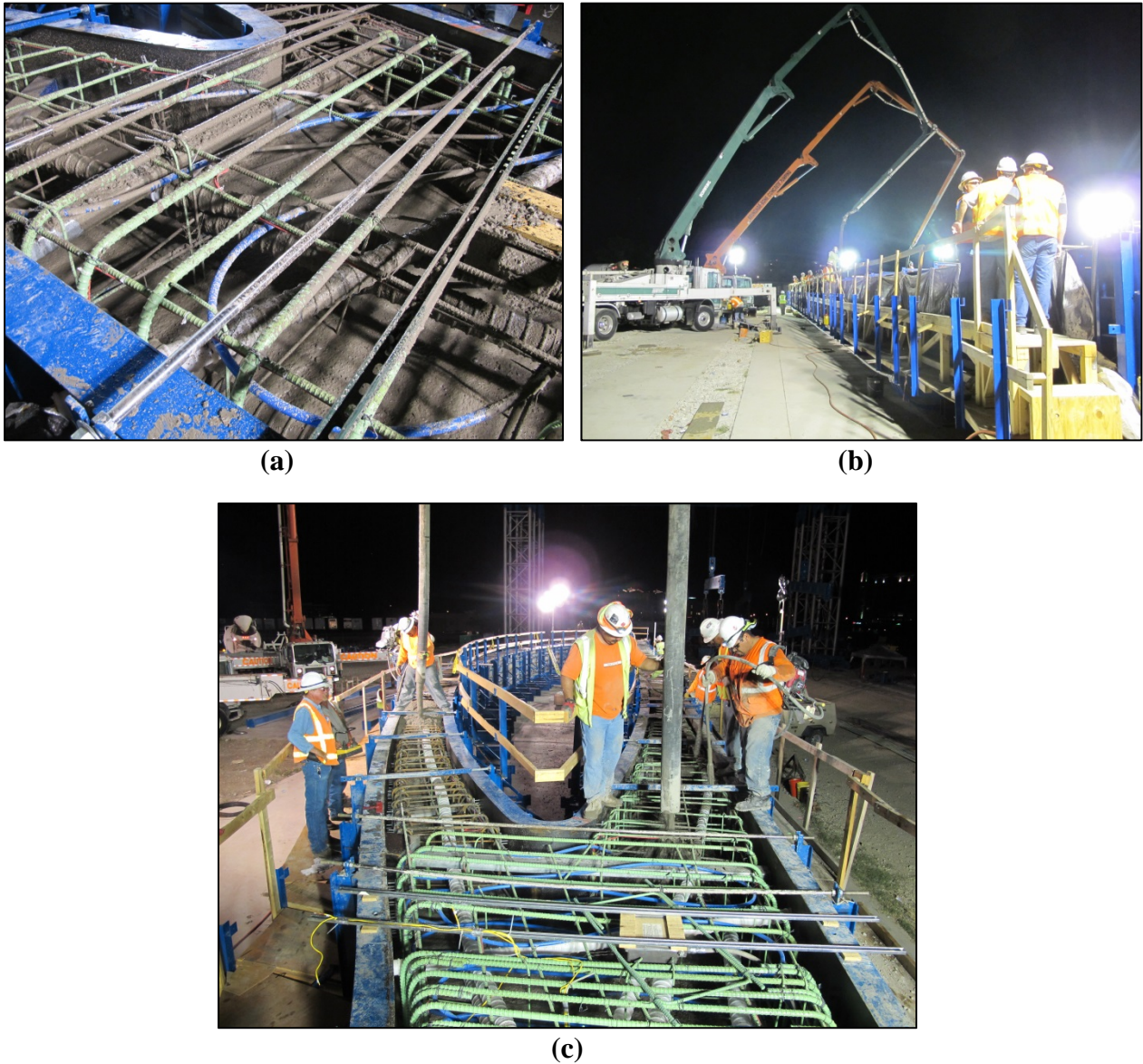
Figure 2.6- Concrete casting operations. (a) Cooling pipes in the knuckle region. (b) The two concrete pumps used for casting the arch. (c) Simultaneous casting of the rib and the tie.
