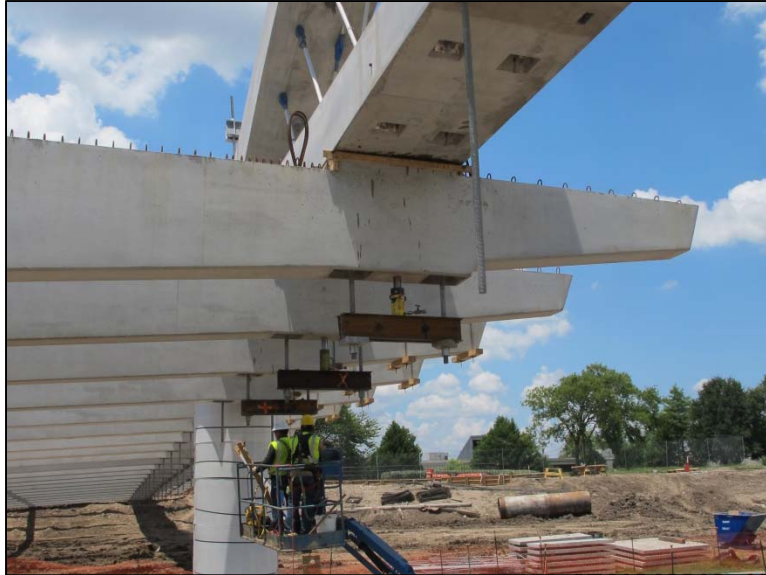
Figure 2.19- Post tensioning the floor beam bars.
