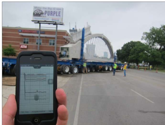
Figure 4.20- Using a smart phone to track stress changes in the structure.
