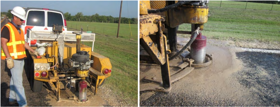
Figure 3.13 Equipment used for coring of the pavement sections.
