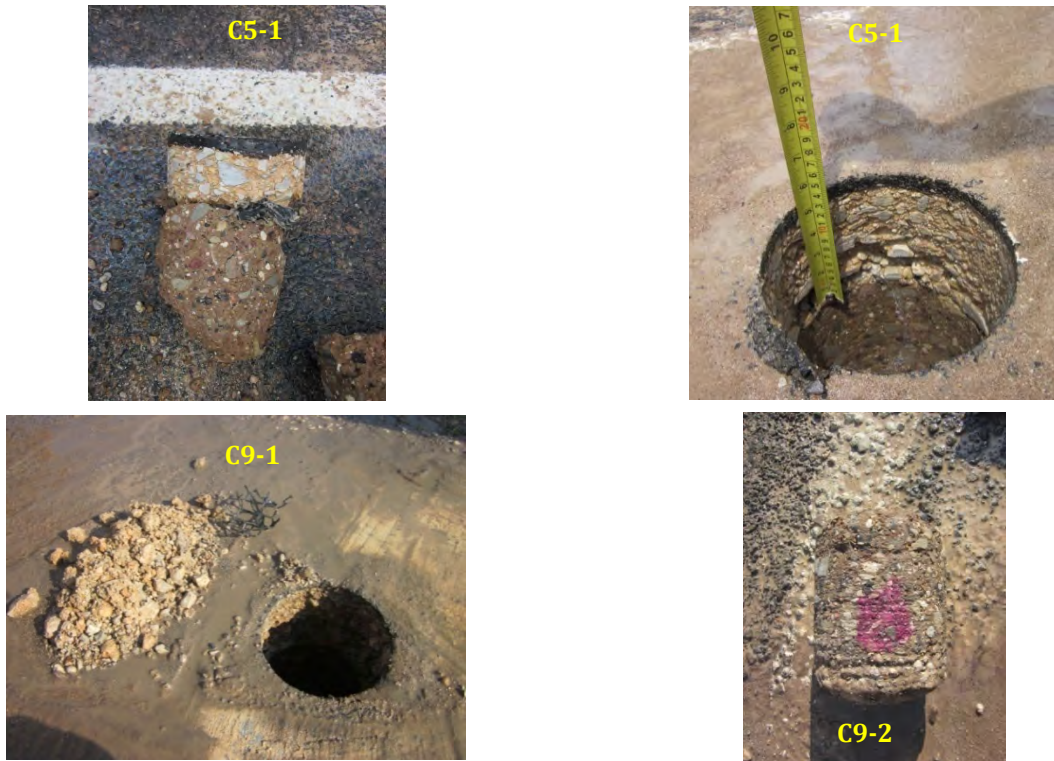
Figure 3.14 Sample pictures from coring operation in August 2012.
