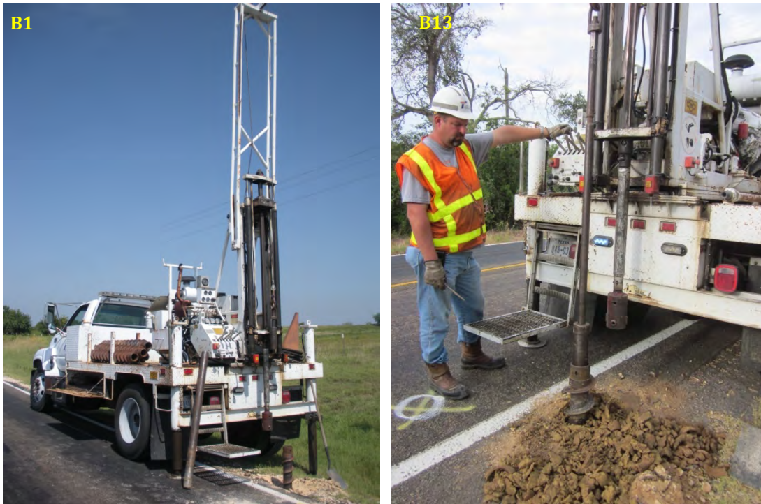
Figure 3.21 Boring operation in August 2012.
