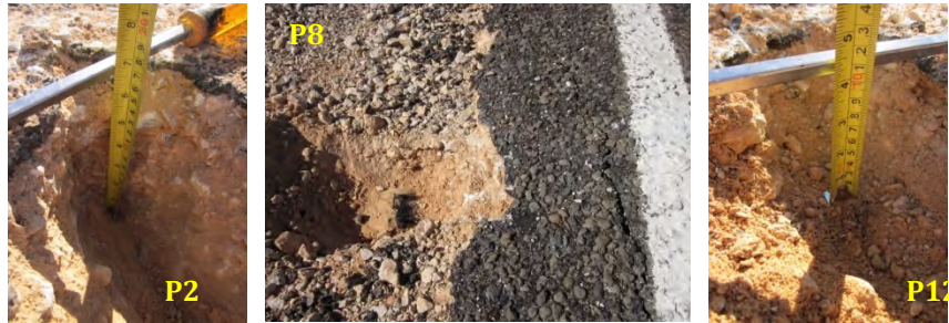
Figure 3.17 Sample pictures of the additional holes excavated in November 2012.
