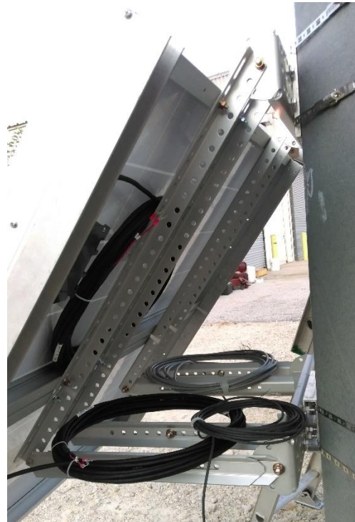
(b) Solar Panel Frames
