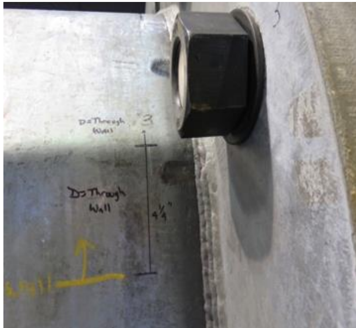
Figure 5.38: Sample of Crack Markings Indicating the Crack Locations, Lengths, and Depths Documented in a Fatigue Test
