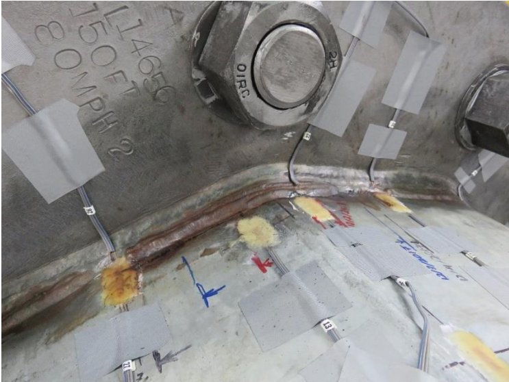
Figure 8.46: Weld-Repaired Specimen 33-3-12-TX-A3 – Bend 1 Following the Fatigue Test: Close-up View
