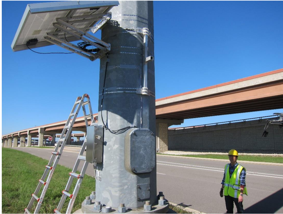
Figure 6.39: Solar Panel Installed on the South Side of the HMIP in Austin
