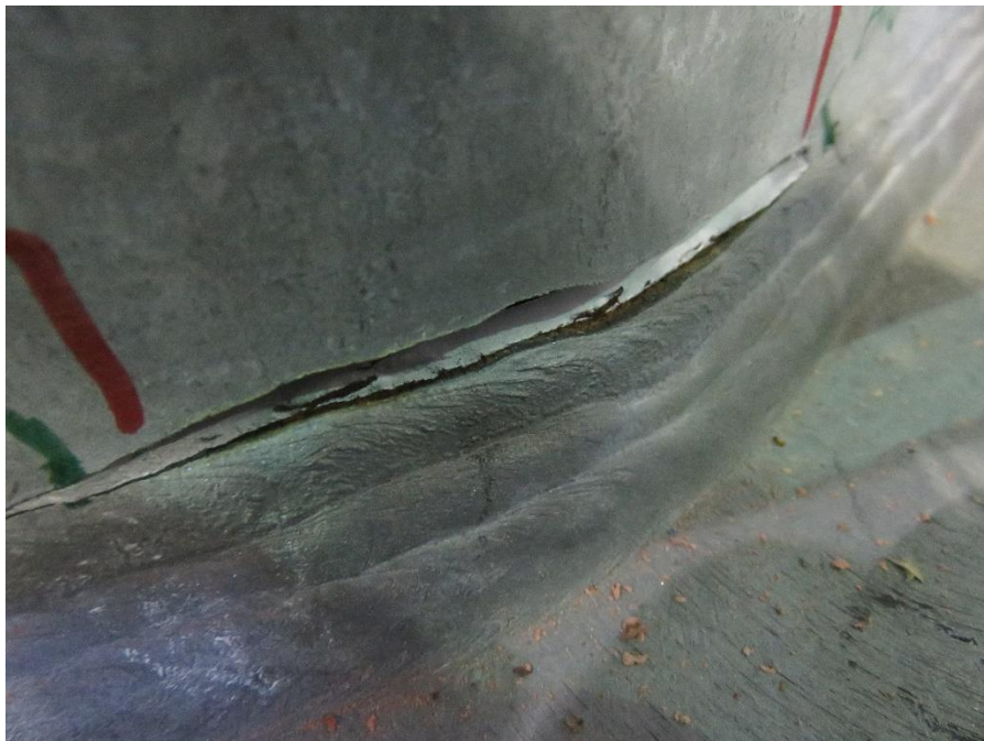
Figure 5.109: Close-up of Cracks on Bend 11 of the Damaged Specimen 33-3-12-TX-A1 – Cracks from a Fatigue test at a stress range of 6 ksi and from the Ultimate Strength Test
