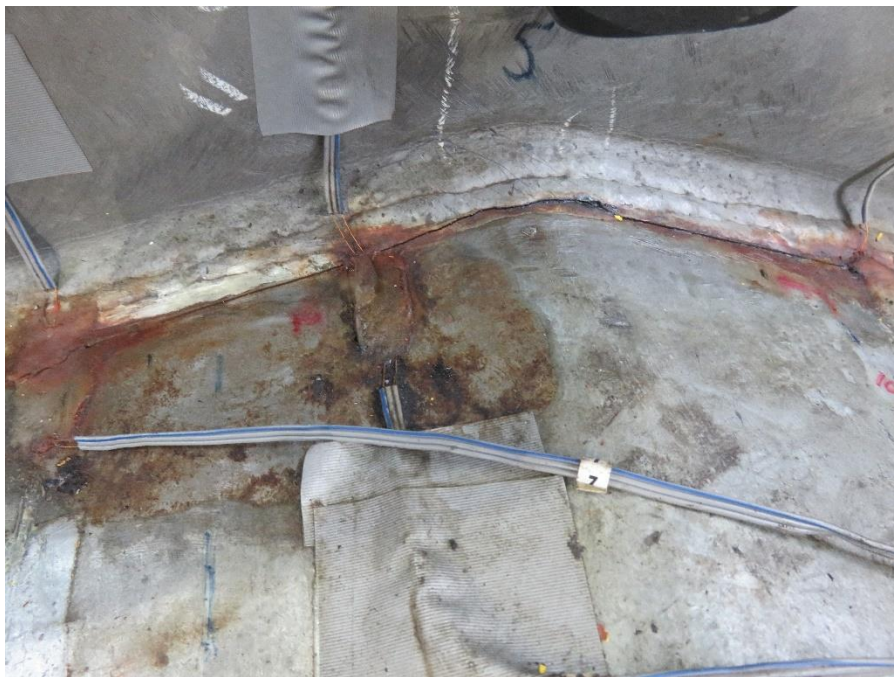
Figure 5.60: Specimen 33-3-12-TX-A6 following the Fatigue Test 2 at the Stress Range of 3 ksi (Fatigue Cracks after 169.0 Million Cycles)
