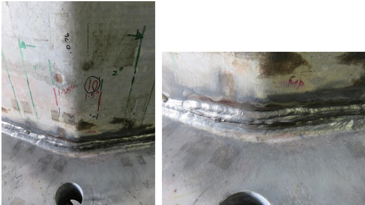
Figure 8.39: Specimen 33-3-12-TX-A3 – Bend 10 Following the Weld-Repair
