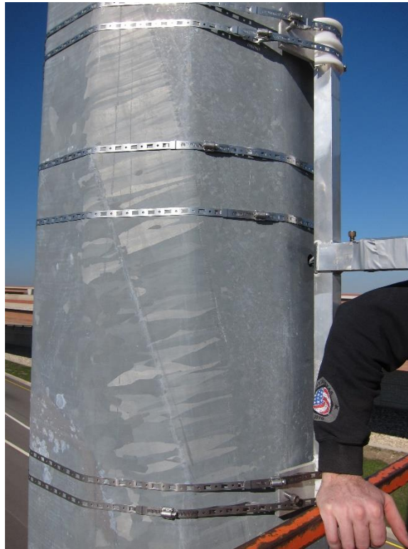
Figure 6.30: Attachment Details for the Anemometer Arms
