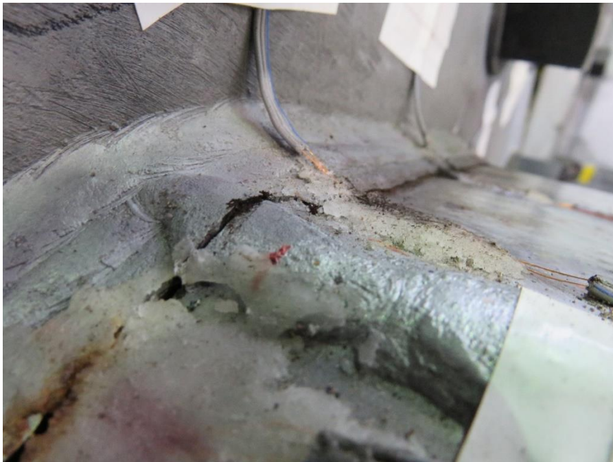
Figure 5.51: Specimen 33-3-12-TX-A1 following the Fatigue Test 1 at the Stress Range of 6 ksi (Fatigue Cracks at Bend 1 [Tested Bend] after 19.4 Million Cycles)
