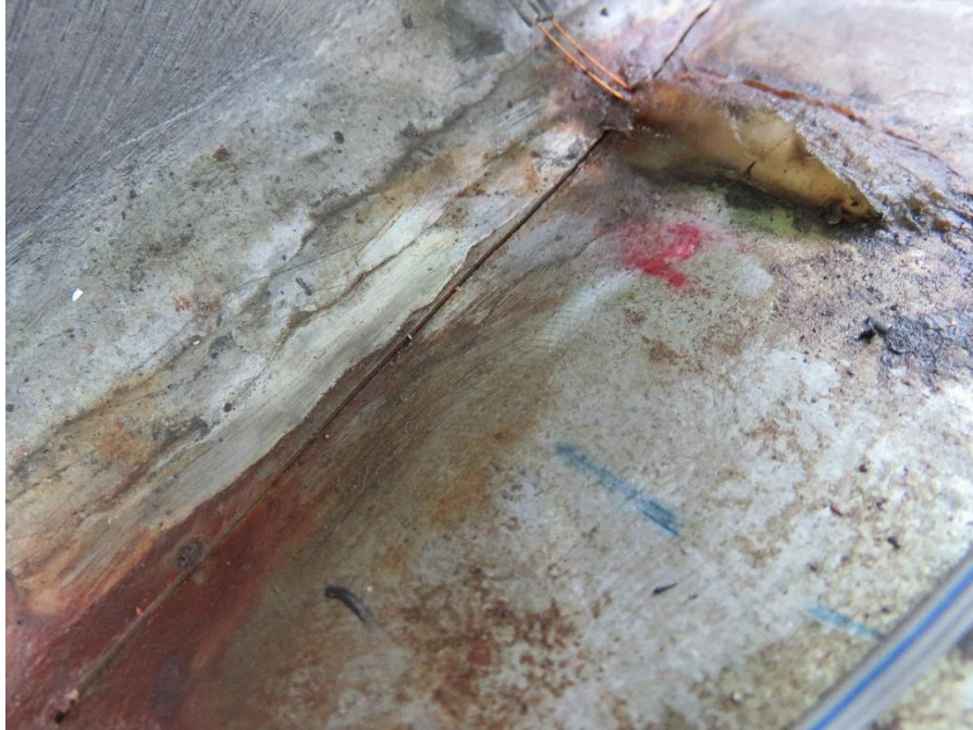
Figure 5.61: Specimen 33-3-12-TX-A6 following the Fatigue Test 2 at the Stress Range of 3 ksi (Fatigue Cracks Close to Bend 5 [Flat 5-6] after 169.0 Million Cycles)
