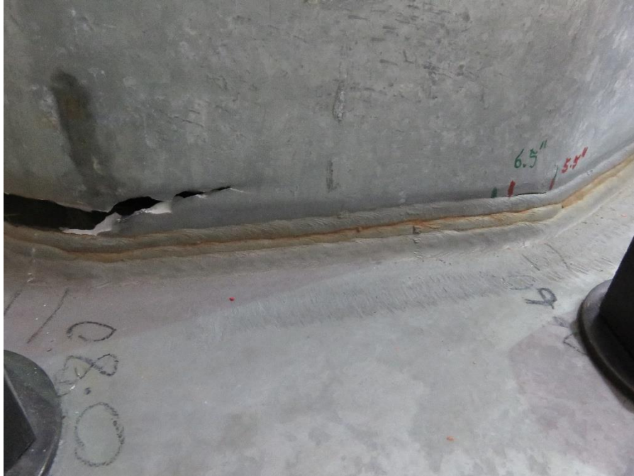
Figure 5.108: Propagation of Cracks from Bends 3 and 4 towards the flat Following the Ultimate Strength Test on the Damaged Specimen 33-3-12-TX-A1
