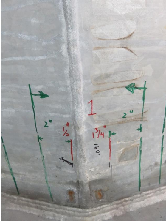
Figure 8.23: State of Cracks: Specimen 33-3-12-TX-A3 – Bend 1
