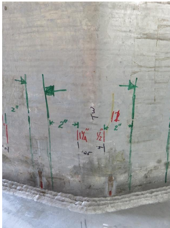
Figure 8.28: State of Cracks: Specimen 33-3-12-TX-A3 – Bend 11
