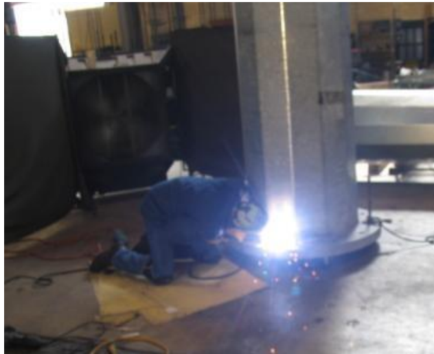
Figure 8.6: The Application of the Field-Repair Procedure at Ferguson Laboratory (Pool 2010)
