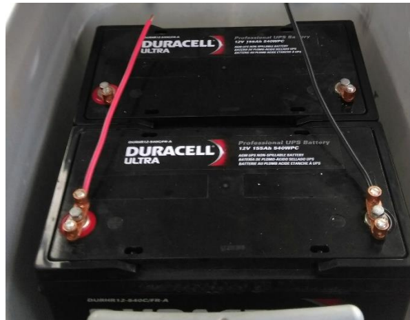
Figure 6.20: AGM Batteries from Duracell
