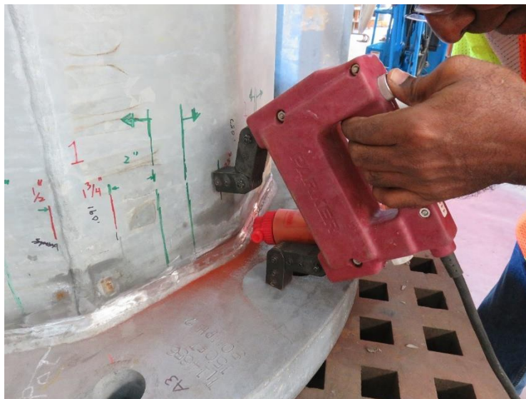
Figure 8.34: Magnetic Particle Testing to Trace the Cracks: Specimen 33-3-12-TX-A3 – Bend 10
