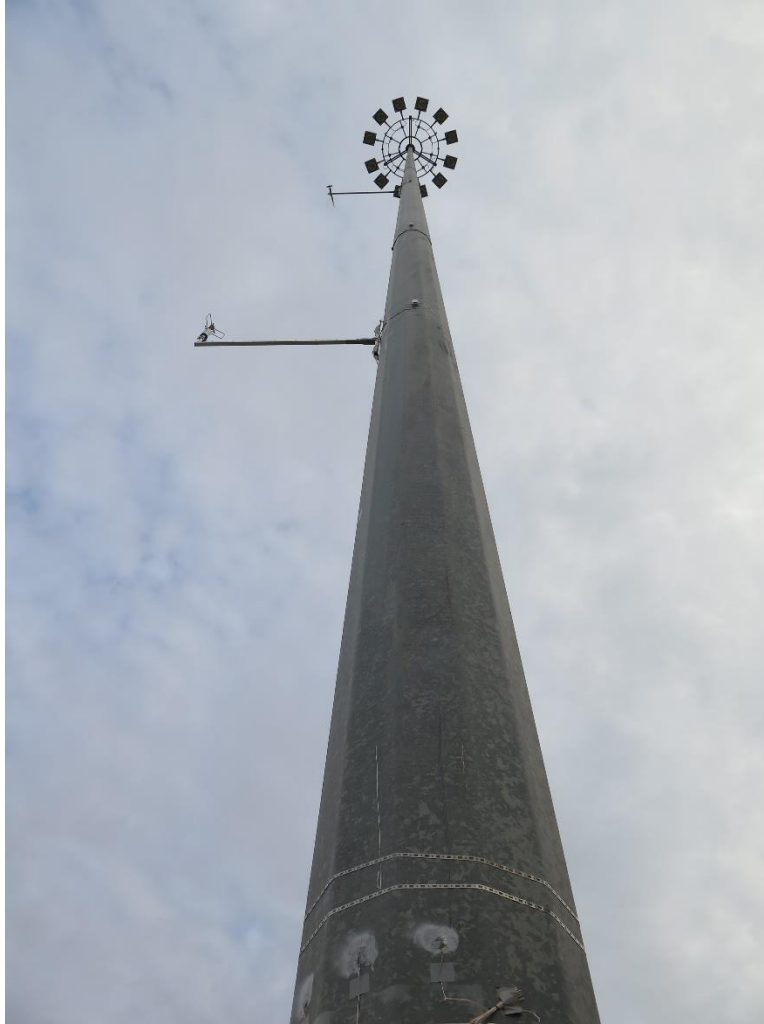
Figure 6.54: Instrumented HMIP in Laredo
