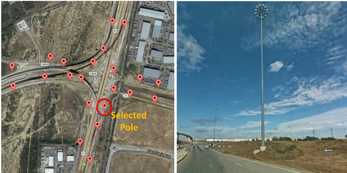
Figure 6.12: Pole for the Field Monitoring in Laredo District
