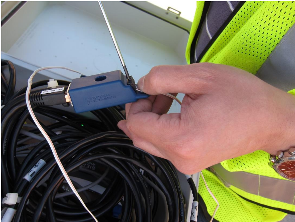
Figure 6.42: Connecting Strain Gauge Cables to the Data Acquisition System
