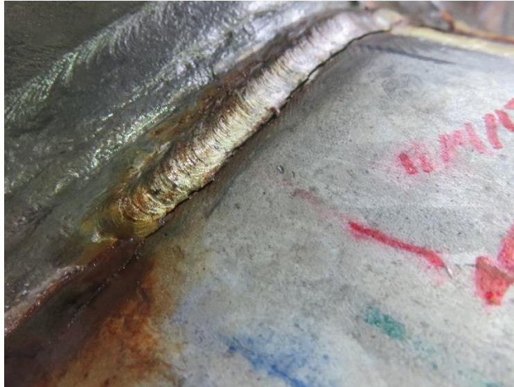
Figure 8.43: Weld-Repaired Specimen 33-3-12-TX-A2 – Bend 5 Following the Fatigue Test: Close-up View
