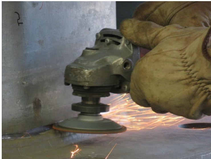
Figure 8.31: Grinding the Shaft Wall Adjacent to the Weld Toe to Remove Cracks – Grinding Technique
