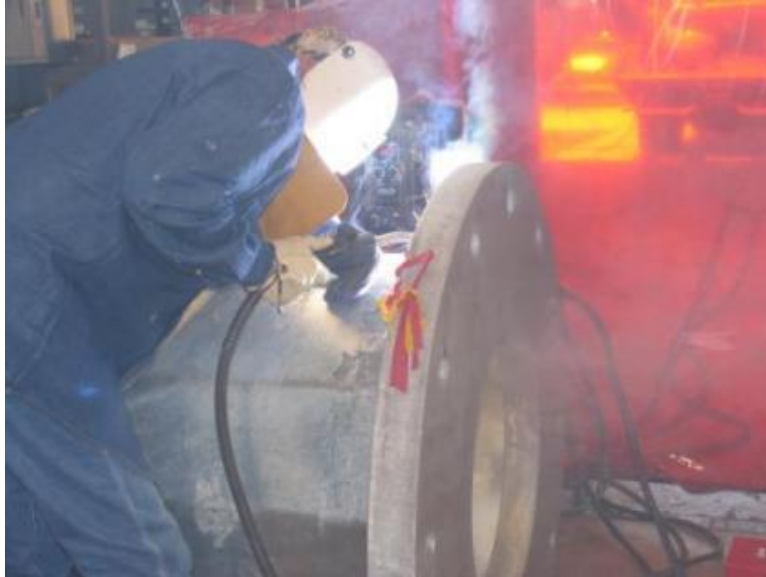
Figure 8.5: FCAW Being Performed at the Ferguson Lab (Pool 2010)
