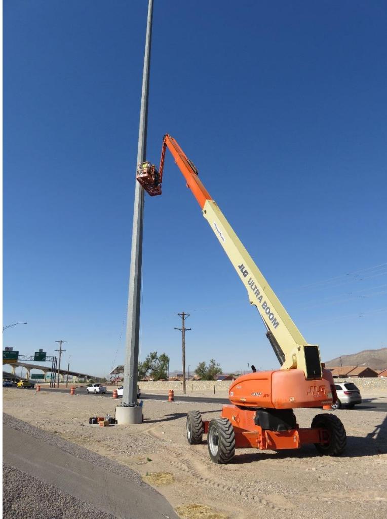
Figure 6.47: JLG Ultra Boom Lift used to Instrument the Selected HMIP in El Paso
