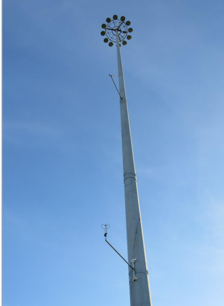
Figure 6.52: Instrumented HMIP in Galveston
