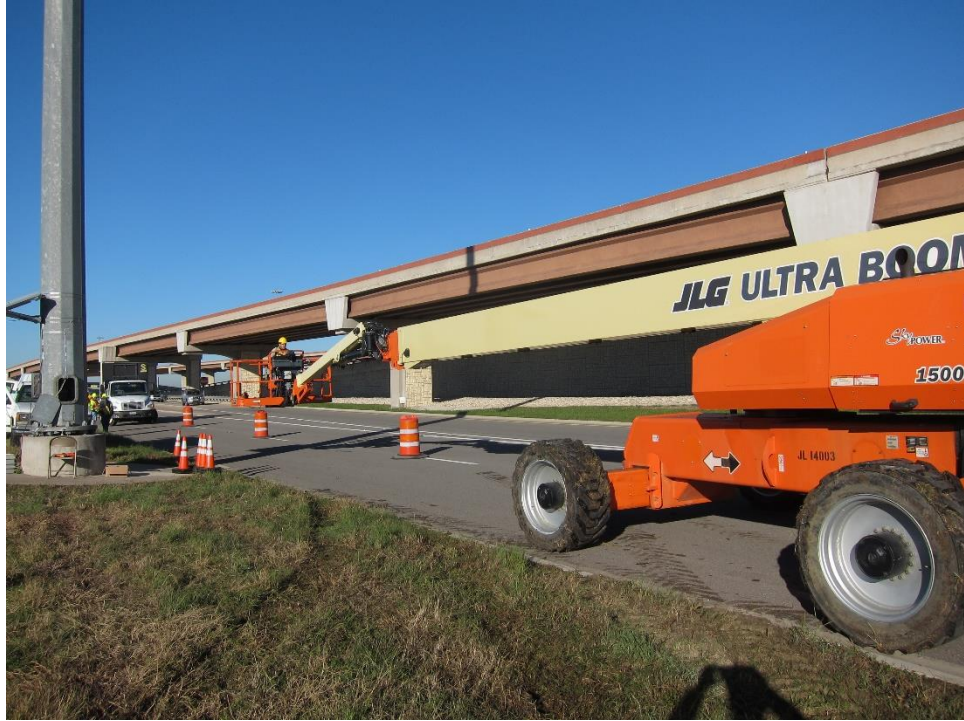
Figure 6.28: JLG Ultra Boom Lift used to Instrument the Selected HMIP in Austin
