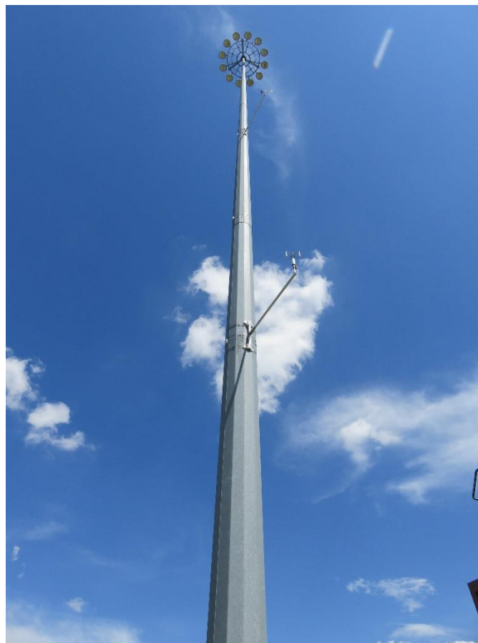
Figure 6.50: Instrumented HMIP in Dallas
