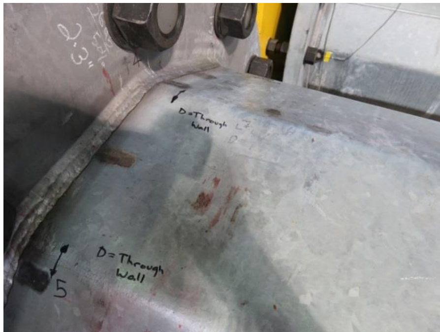
Figure 5.39: Sample of Crack Markings for a Specimen with Severe Cracking in a Fatigue Test
