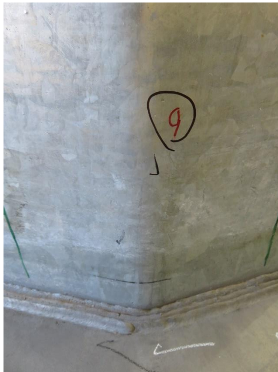
Figure 8.18: State of Cracks: Specimen 33-3-12-TX-A2 – Bend 9
