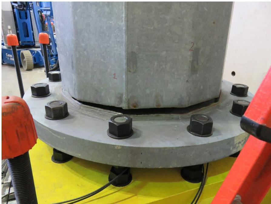
Figure 5.105: Tension Side of the Damaged Specimen 33-3-12-TX-A1 Following the Ultimate Strength Test
