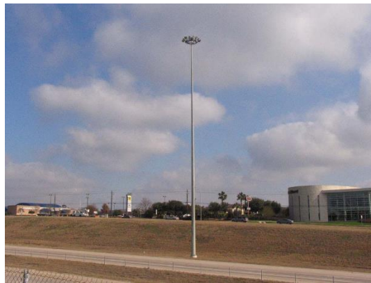
Figure 2.1: Typical High Mast Illumination Pole (Rios 2007)
