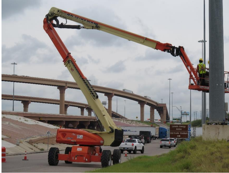
Figure 6.53: JLG Ultra Boom Lift used to Instrument the Selected HMIP in Laredo
