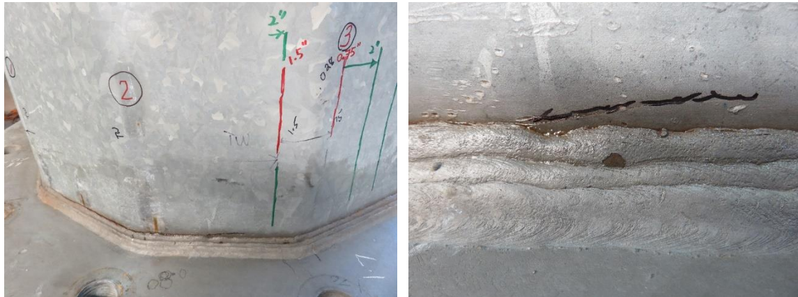
Figure 8.22: Cracks Propagating Away from the Weld Toe: Specimen 33-3-12-TX-A2 – Bend 2
