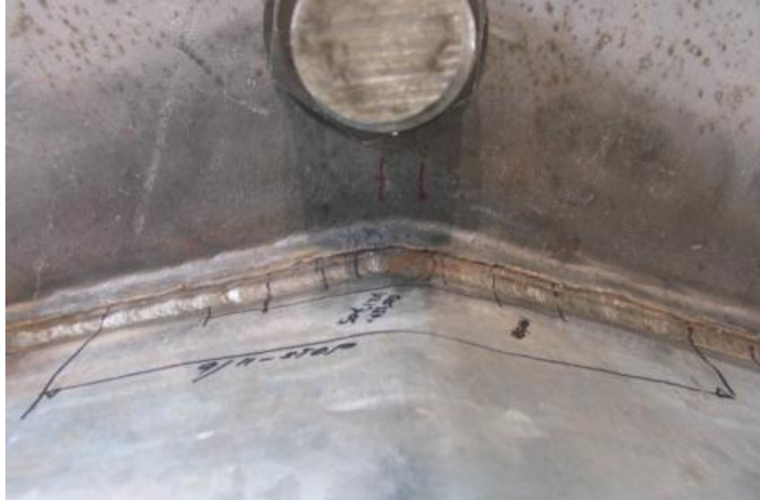
Figure 8.7: Bend 11 of the Field-Repaired Specimen with Failure through Weld
