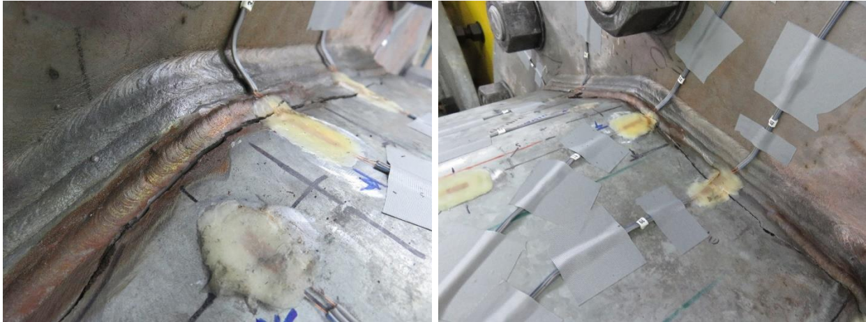
Figure 8.49: Weld-Repaired Specimen 33-3-12-TX-A2 – Bend 8 Following the Fatigue Test: Close-up View
