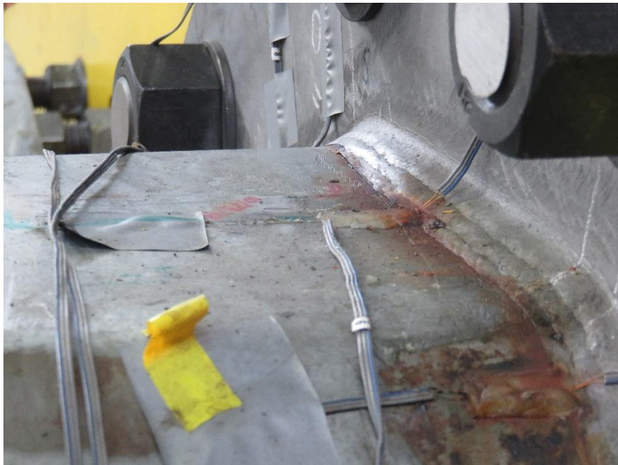
Figure 5.62: Specimen 33-3-12-TX-A6 following the Fatigue Test 2 at the Stress Range of 3 ksi (Fatigue Cracks Close to Bend 5 [Flat 4-5] after 169.0 Million Cycles)
