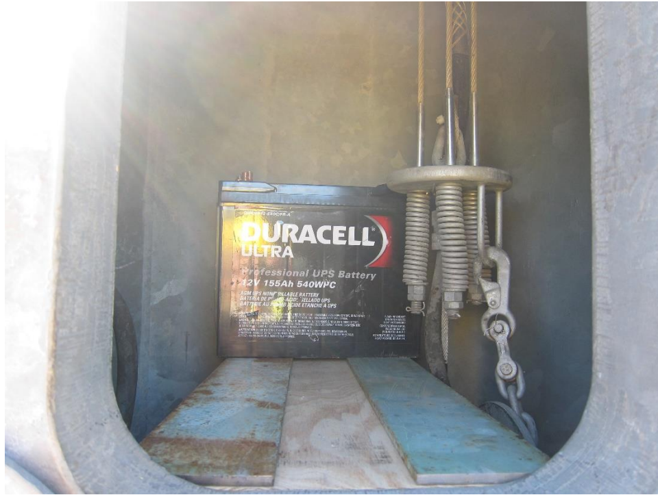
Figure 6.40: Battery Situated inside the HMIP
