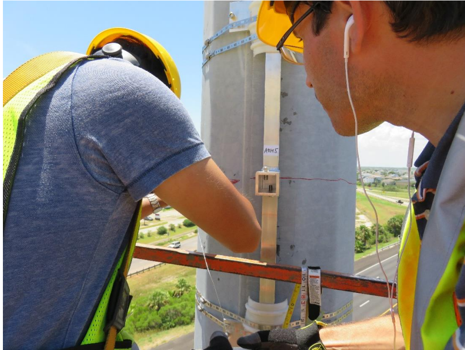
Figure 6.34: Threading the Fishing Wire inside the HMIP
