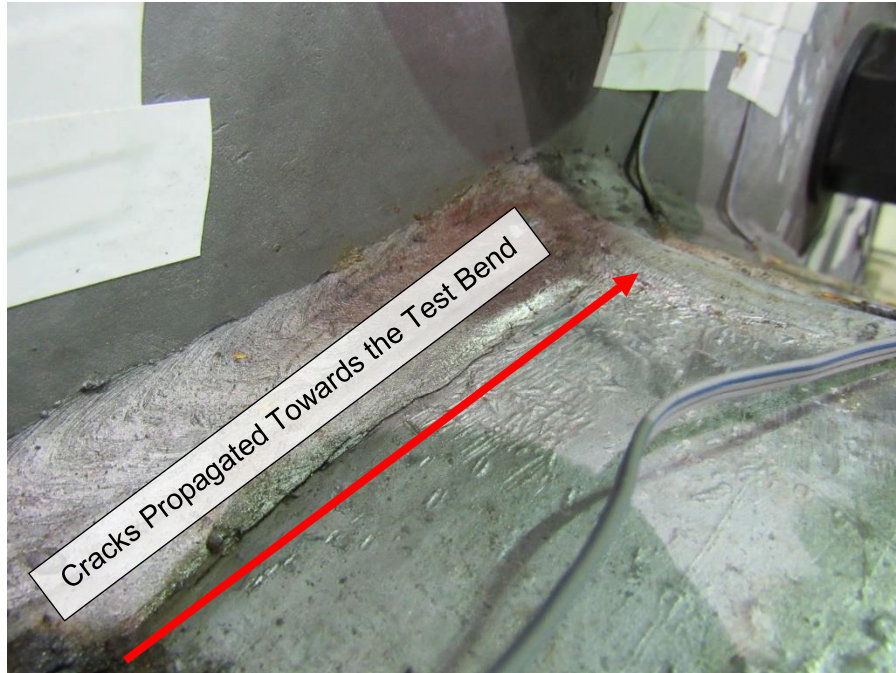
Figure 5.52: Specimen 33-3-12-TX-A2 following the Fatigue Test 1 at the Stress Range of 6 ksi (Fatigue-Crack Propagation after 19.4 Million Cycles)
