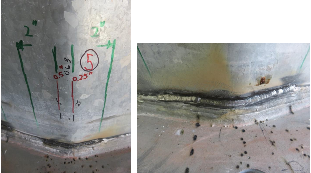
Figure 8.40: Specimen 33-3-12-TX-A2 – Bend 5 Following the Weld-Repair
