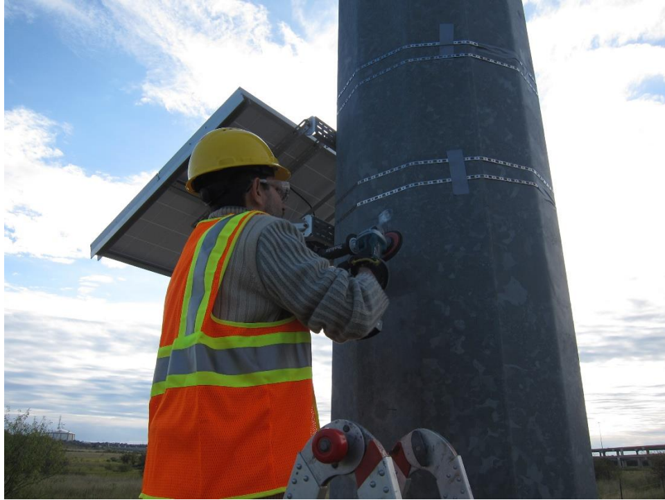
Figure 6.35: Preparation of the Surface to Install Strain Gages
