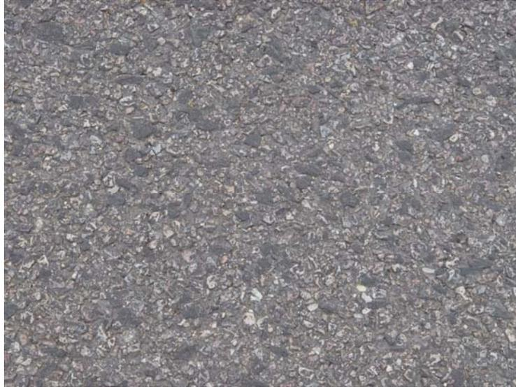
*Figure 6.11: IH30 PFC placed in 2006 in its current condition (September 2014)*
