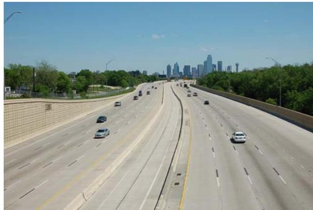
Figure 6.4: Aspect of the IH30 section showing transversely tined CRCP (2006)
