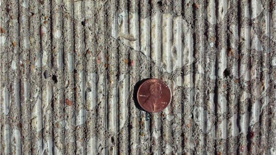
*Figure 5.46: Diamond-ground surface on IH 35W (Section 1)*
