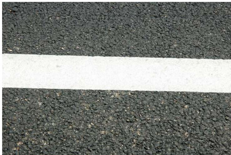
*Figure 6.12: IH30 PFC placed in 2010, just after construction (August 2010)*
