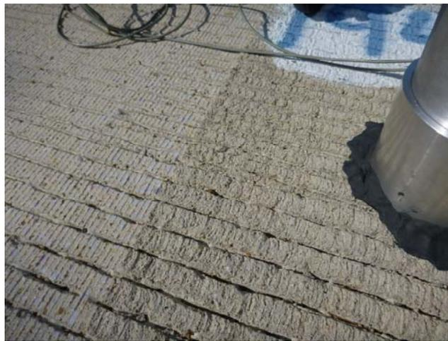
*Figure 5.54: 1-in. transverse tined surface at TTI test track*
