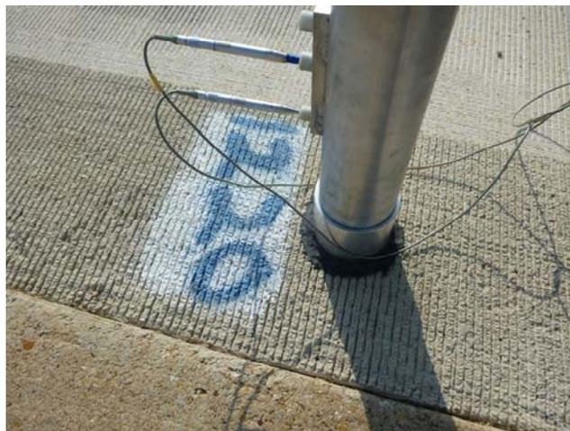
*Figure 5.55: 1/2-in. transverse tined surface at TTI test track*
