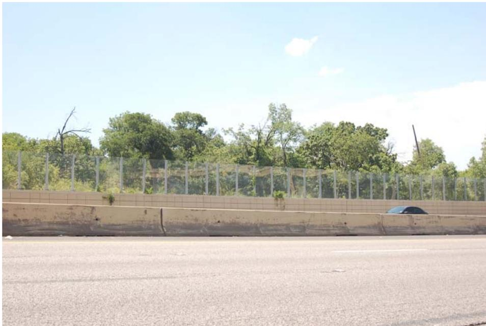
*Figure 5.25: Noise wall along IH30 section*
