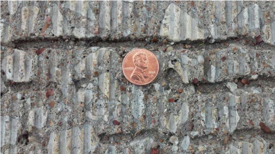
*Figure 5.47: Diamond-ground surface on IH 35W (Section 3)*
