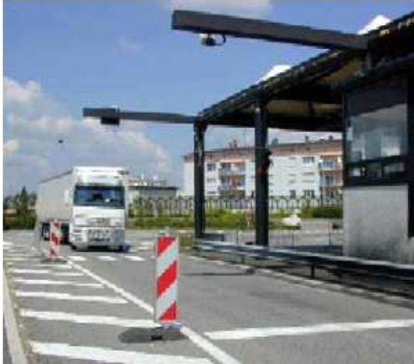
Source: Switzerland Federal Customs Administration, 2013 Figure 5.11 Overhead radio beacons in Switzerland
