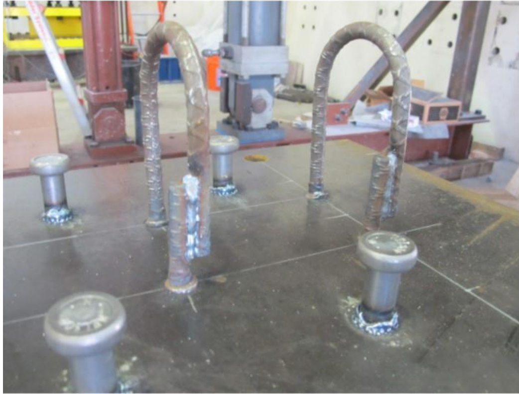
Figure 7.7 Rebar and Studs Welded to Base Plate
