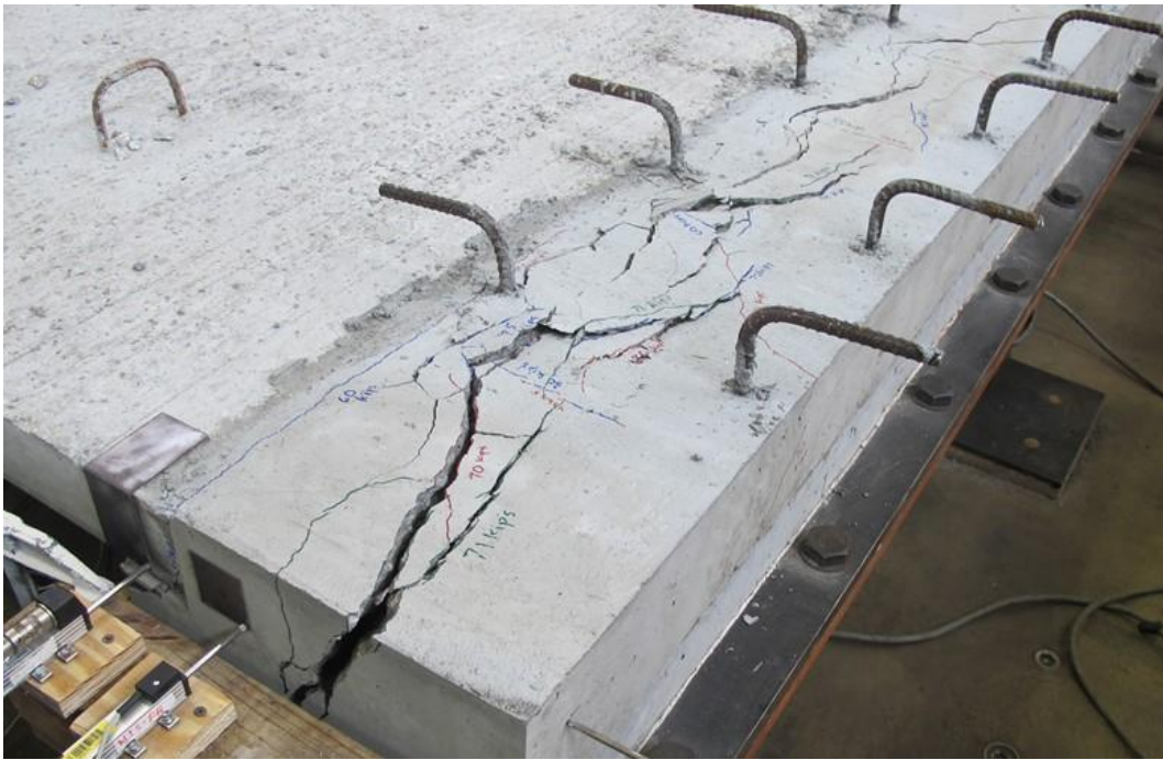
Figure 7.32 Cracking in Closure Pour (Original Detail) at 84 kips
