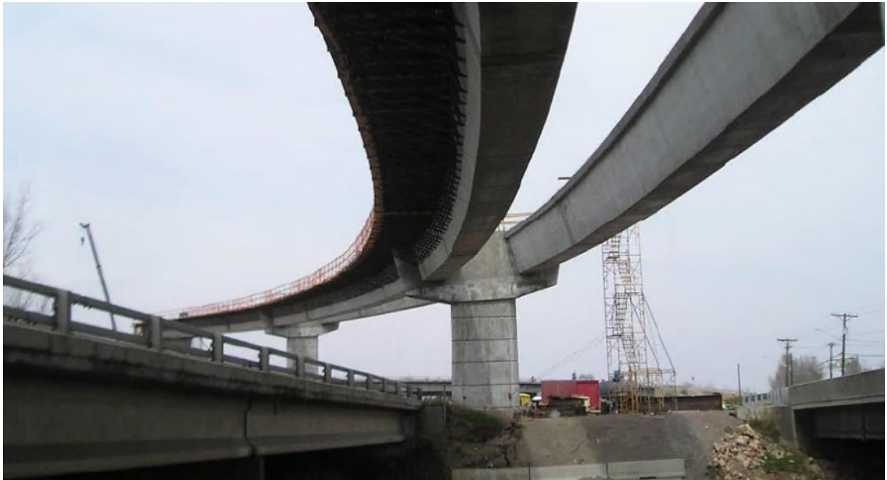
Figure 10.12 Stage-2-a PCP Panels between Girders Placed and Shoring Tower Removed (Reese and Nickas 2010)
