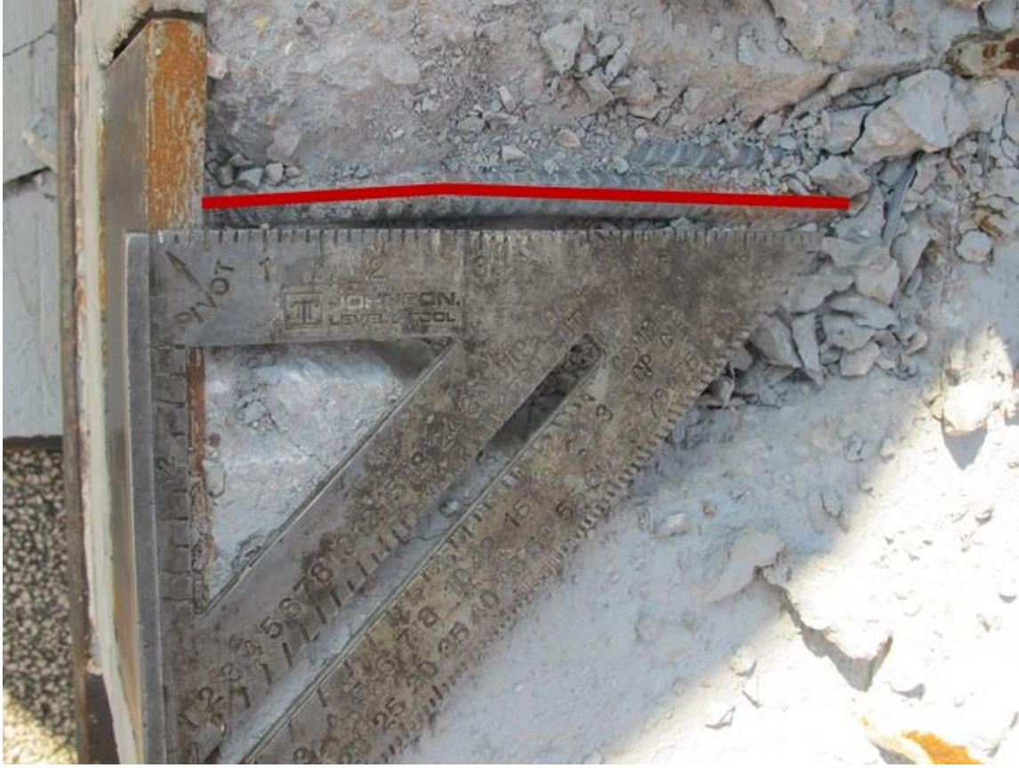
Figure 7.38 Bending of Cap Plate Long. Reinforcement
