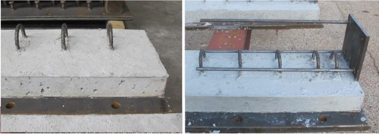
Figure 7.23 (a) Original R-Bar Layout and (b) Modified Corner R-Bar Layout
