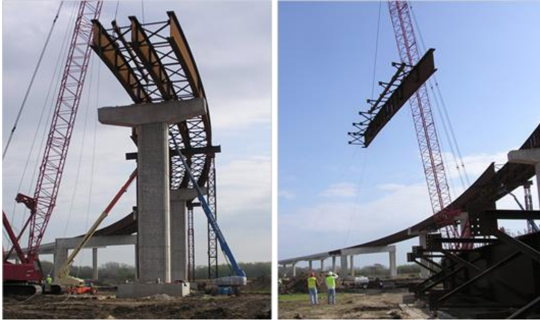
Figure 1.1: Splicing of Curved I-Girders to Form a Continuous Girder (Photo Courtesy of T. Helwig)
