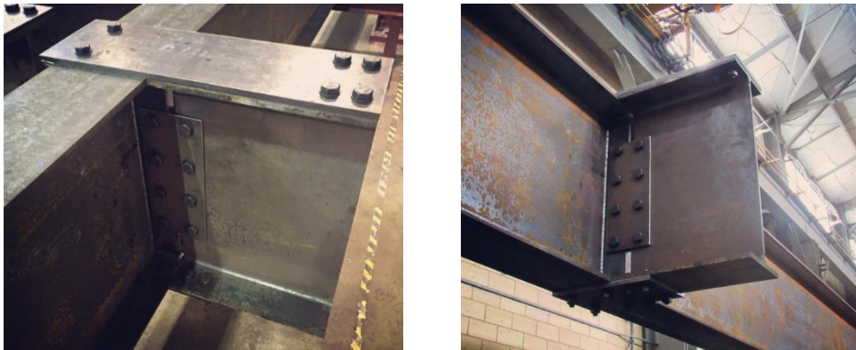
Figure 5.15 Eccentric Loading Brackets
