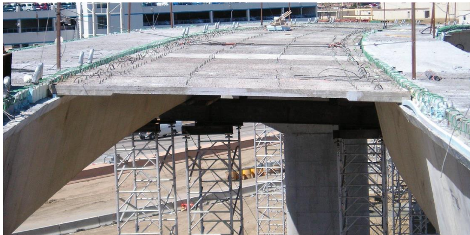
Figure 1.9: Longer span PCP's for Colorado Curved U-Beams (Reese and Nickas 2010)
