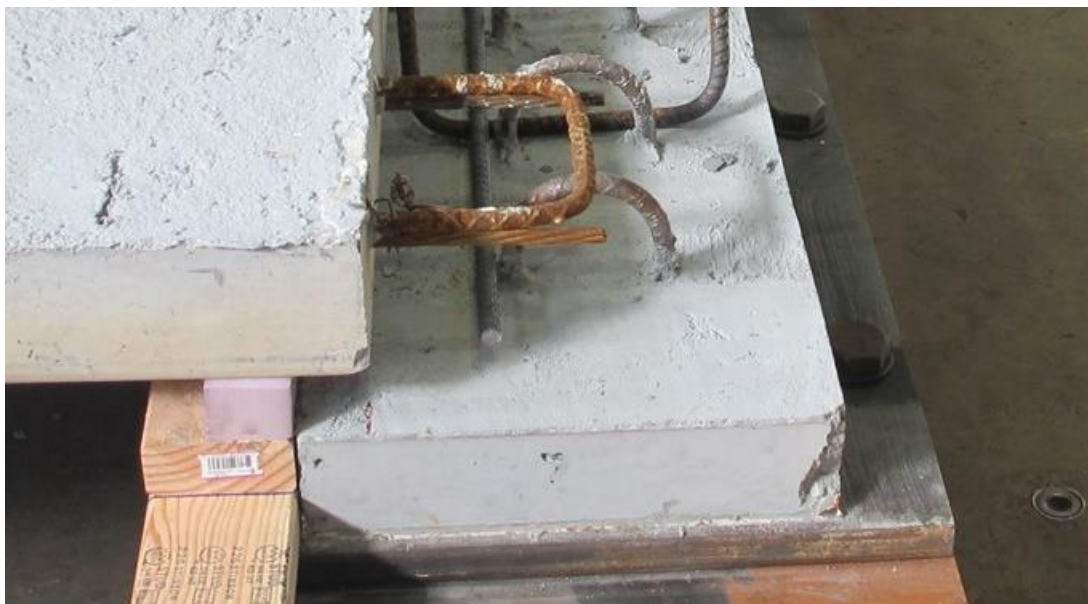
Figure 7.9 Installation of Precast Panel
