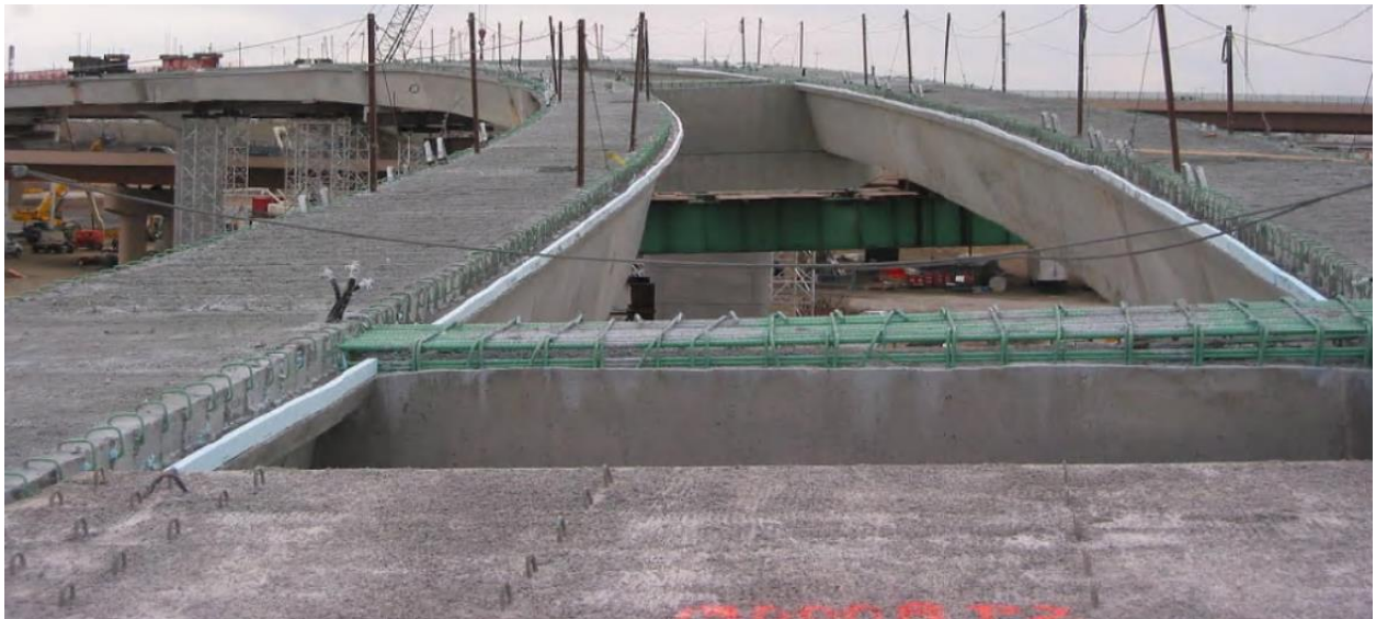
Figure 10.11 Stage-1-c PCP between Webs Placed and Lid Slab with Closure Pour Cast in Place and Cured prior to Post-tensioning (Reese and Nickas 2010)
