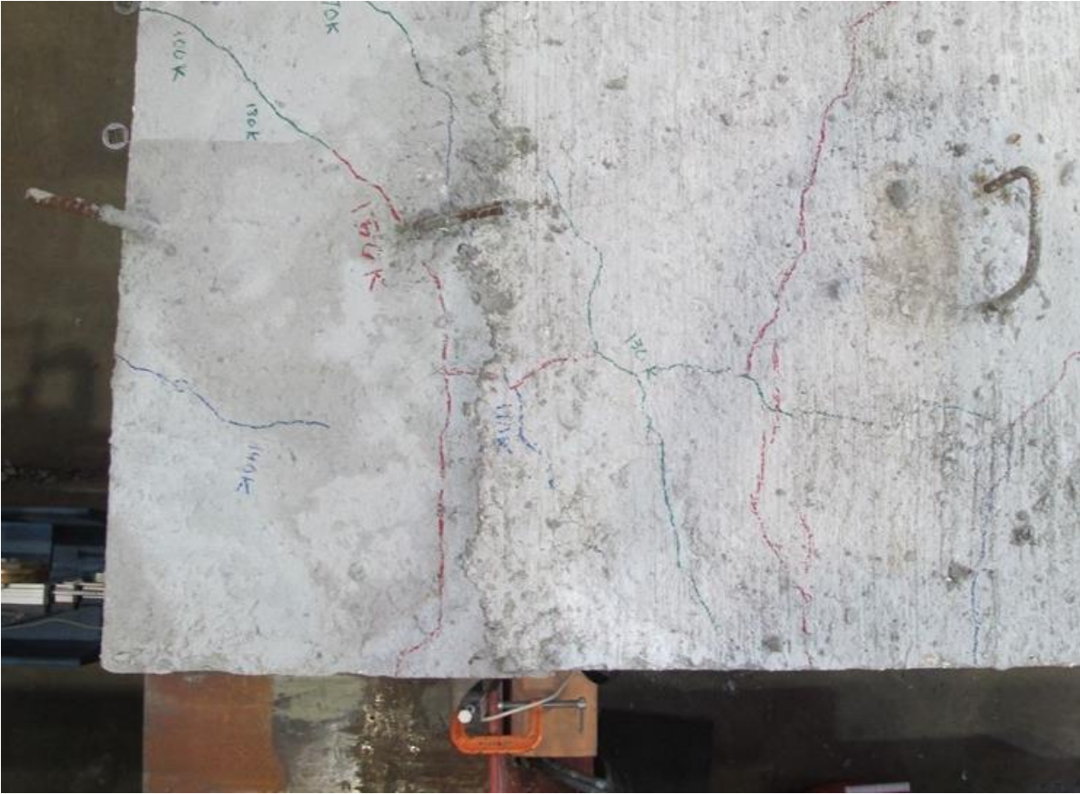
Figure 7.52 Cracking at SW Corner of Precast Panel
