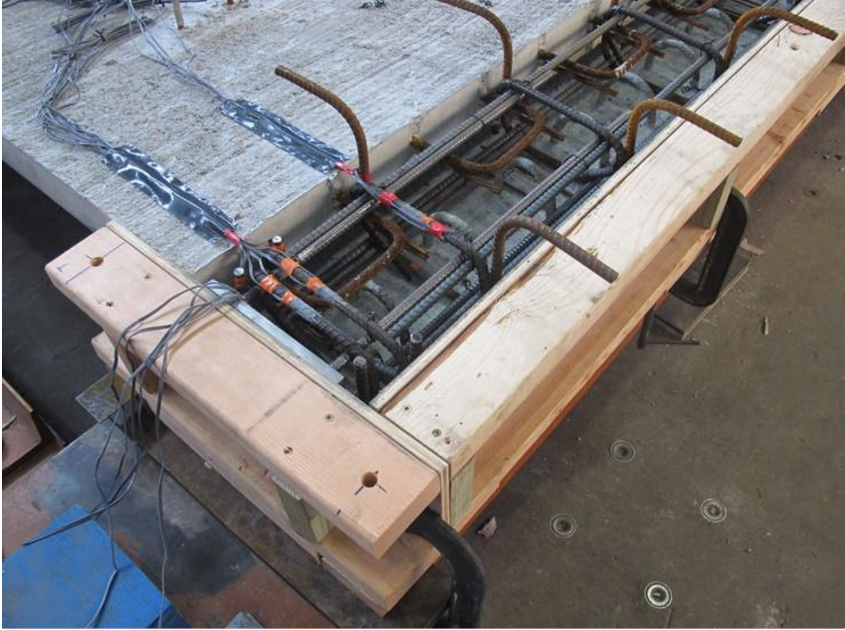
Figure 7.16 Closure Pour with Additional Shear Reinforcement at Corner
