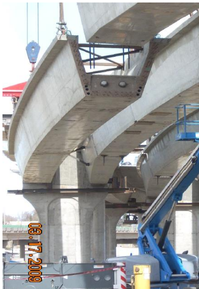
a) During Lifting
