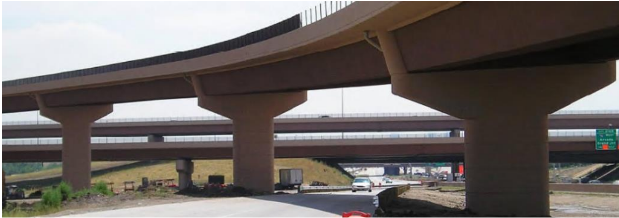
Figure 10.13 Stage-2-b Deck Placed or Cast in Unshored Conditions (Reese and Nickas 2010)
