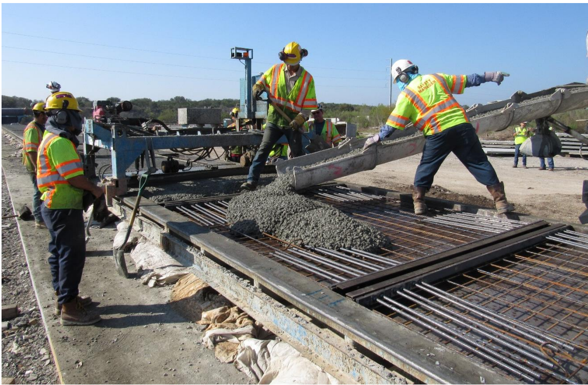
Figure 4.4: Casting Prestressed PCPs with Embeds
