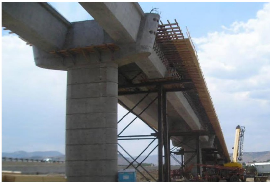
Figure 10.10 Stage-1-b Cast of Splice, Pier Diaphragm, and Expansion Diaphragm (Reese and Nickas 2010)
