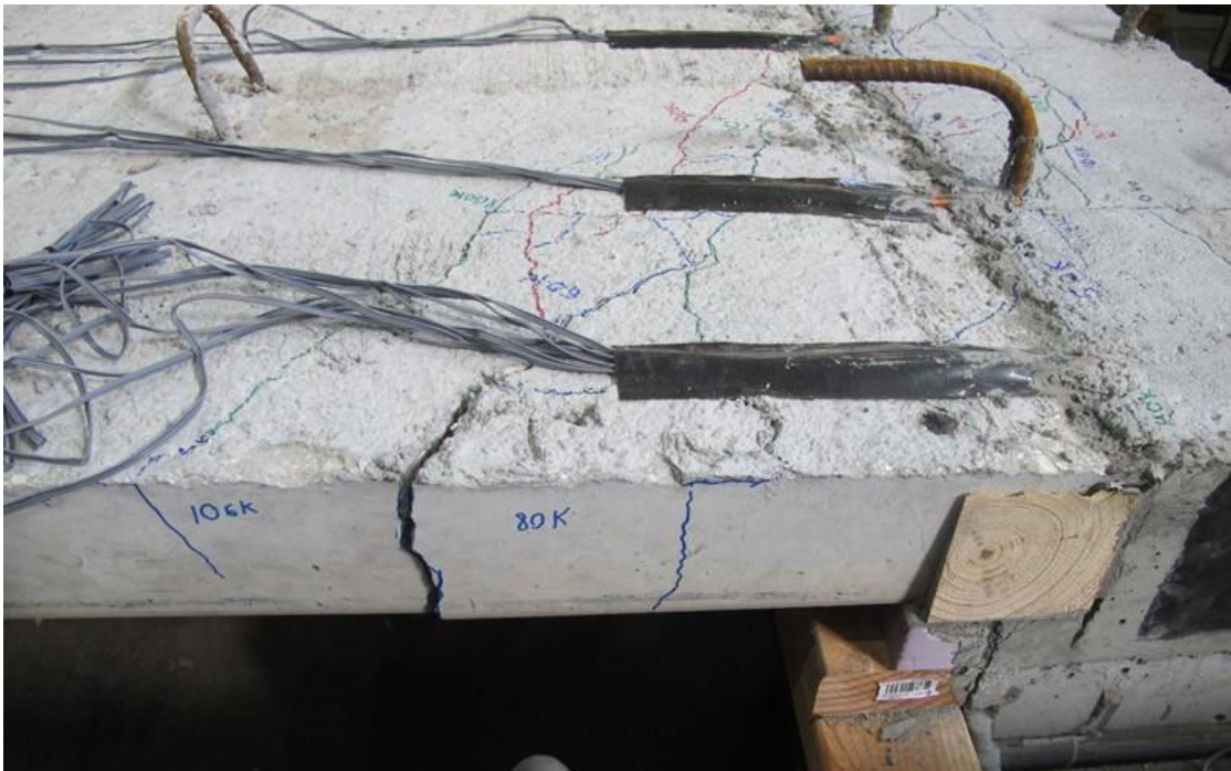
Figure 7.40 Cracking in Precast Panel at 113 Kips of Shear
