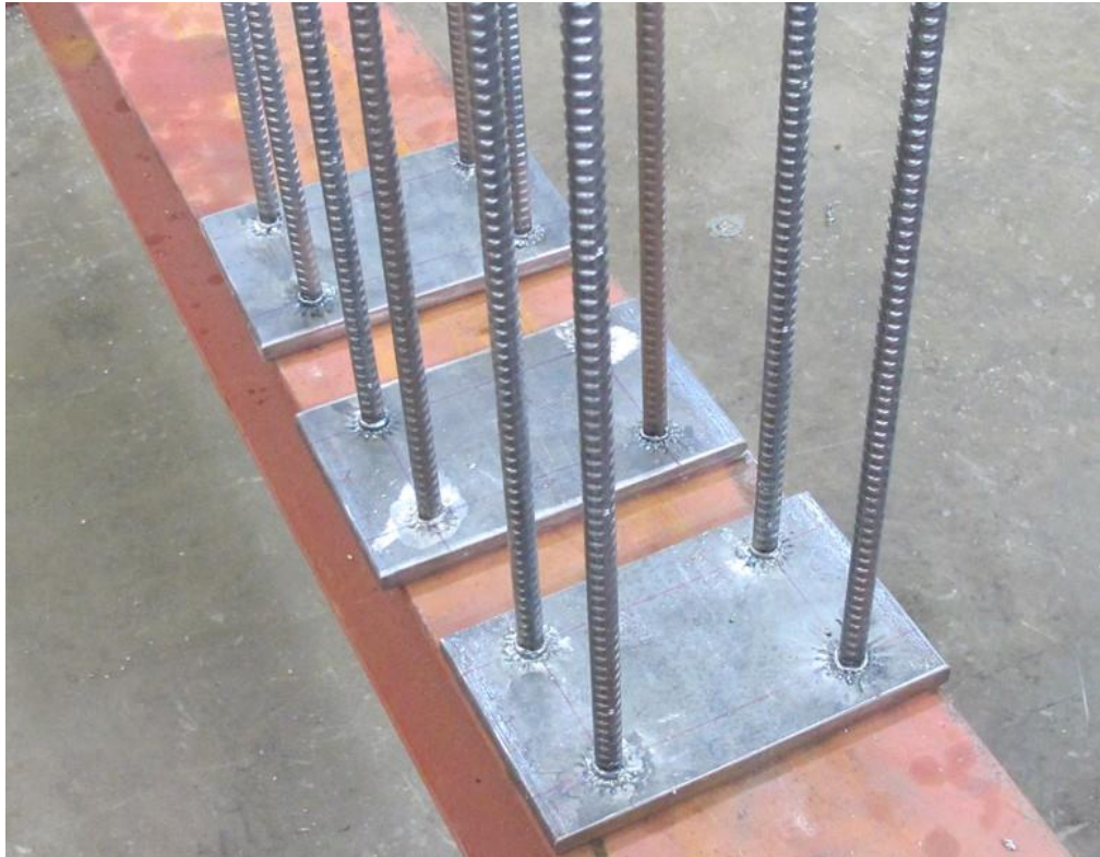
Figure 7.13 Fabricated Cap Plate
