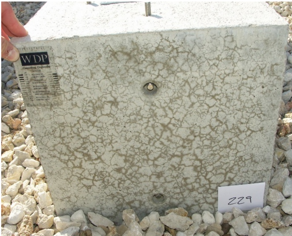
Figure 6-5: Example of Crack Rating = 4.5
