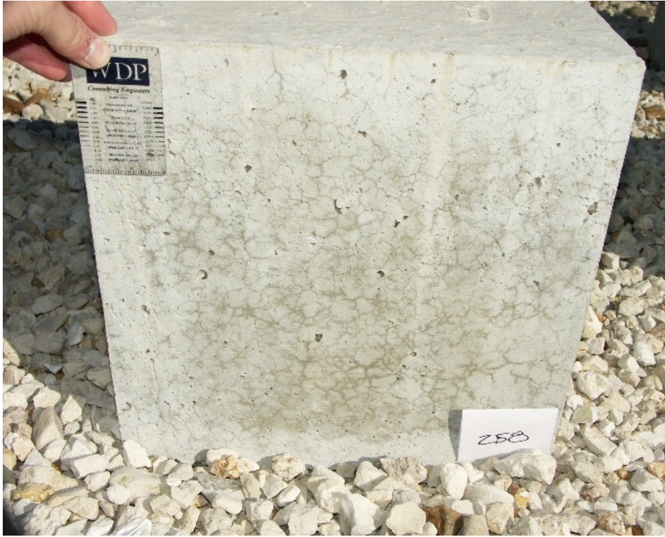
Figure 6-4: Example of Crack Rating = 3
