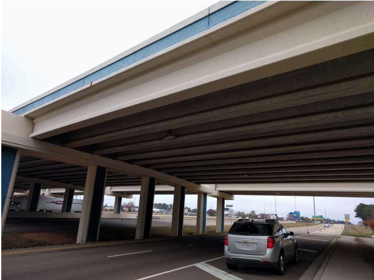
Figure 2-13: Overall view of site facing north (visible exterior girder is referred to as G1)
