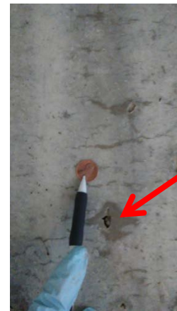
Figure 2-21: Surface defects on cracked girder at Dallas site (2)
