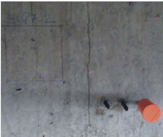
Figure 2-9: Overall photo of G7 with corresponding humidity measurement probes and crack map G7-2
