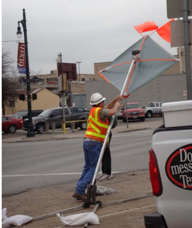
Figure 5.1: Incorrect shoulder placement
