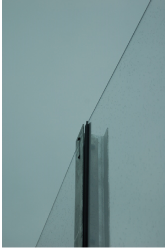
Figure 7.12: Gap between vertical gasket and metal support
