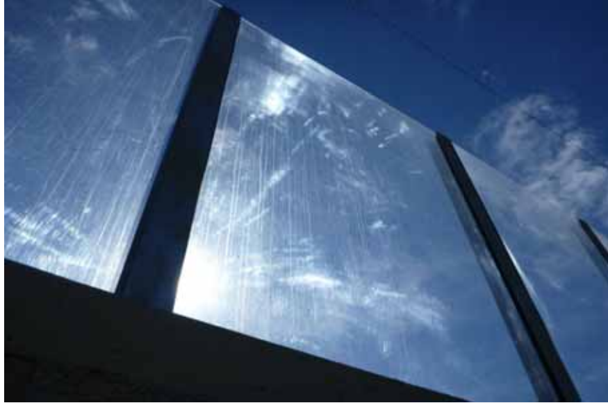
Figure 7.24: Cleaned panel showing traces of the cleaning operation
