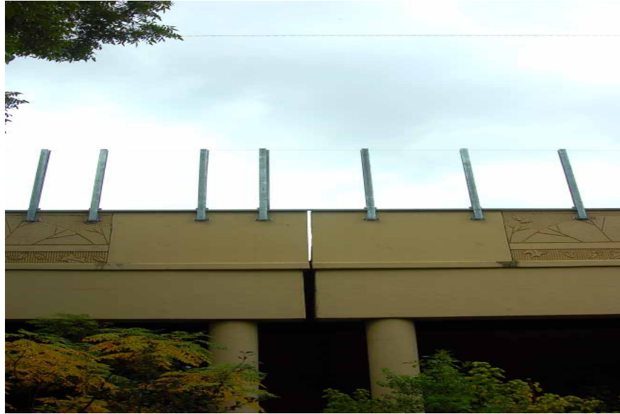
Figure 7.15: Gap in existing concrete wall at bridge expansion joint as seen from Coombs Creek
