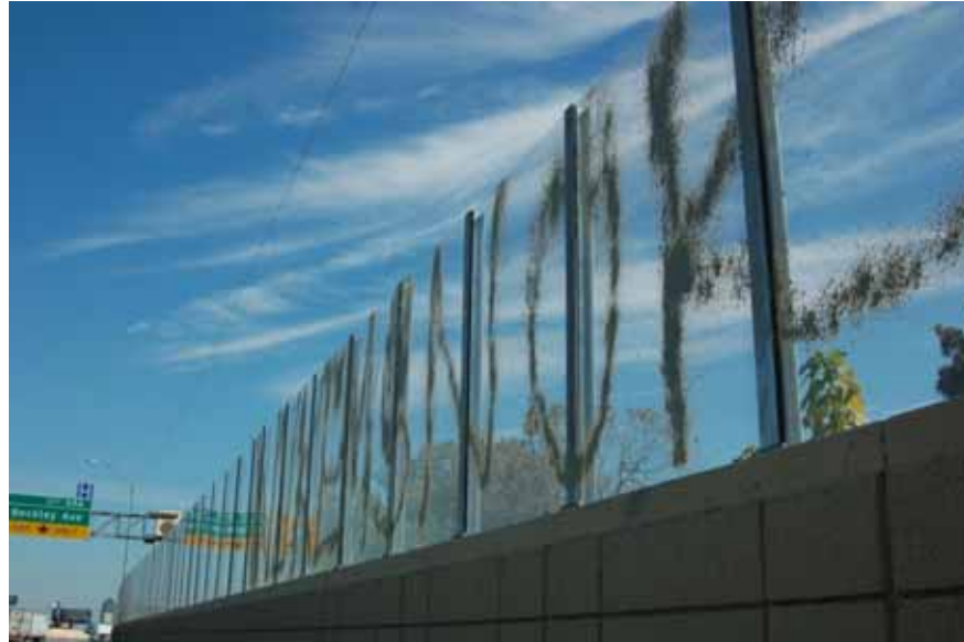
Figure 7.17: Graffiti as seen from the highway shoulder on November 11, 2013
