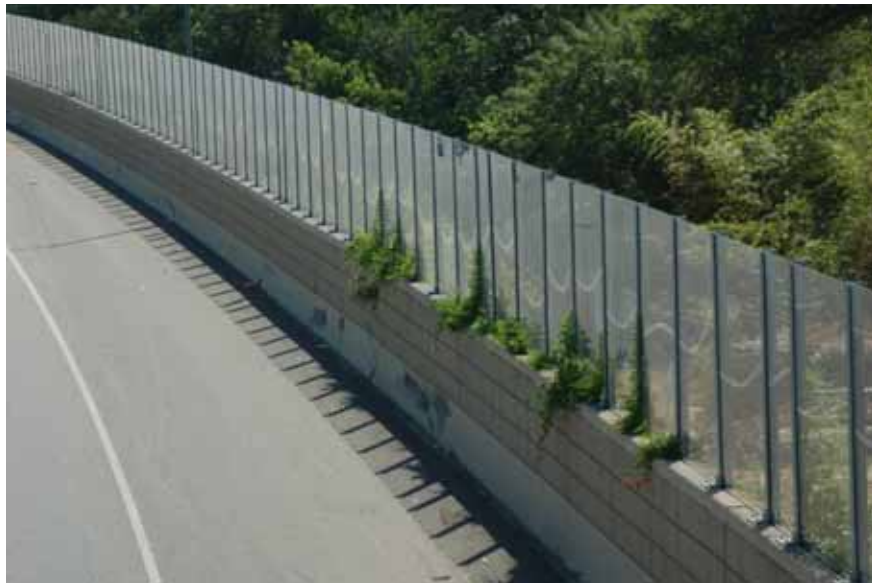
Figure 7.35: Vegetation from the creek side growing through the openings in the gaskets under noise barrier
