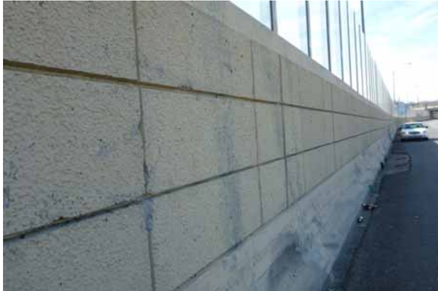
Figure 7.26: Remnants of the graffiti on the concrete wall below the panels
