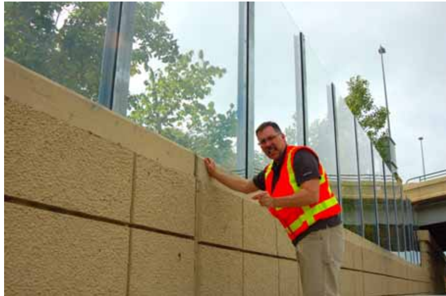
Figure 7.14: Armtec’s Mark McIlheran inspecting the wall, showing the gap size between a panel and the gasket
