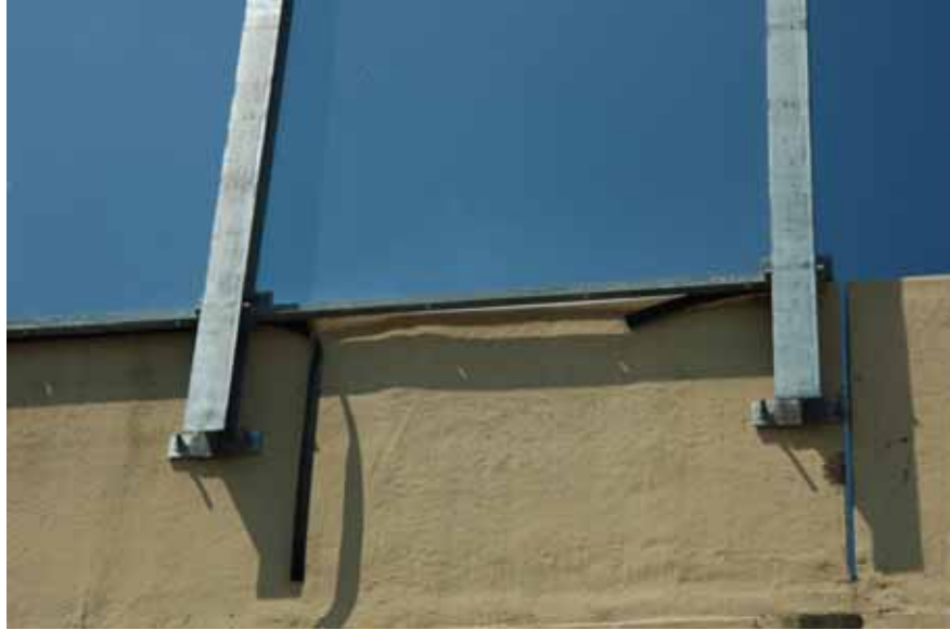
Figure 7.32: Broken horizontal rubber gasket
