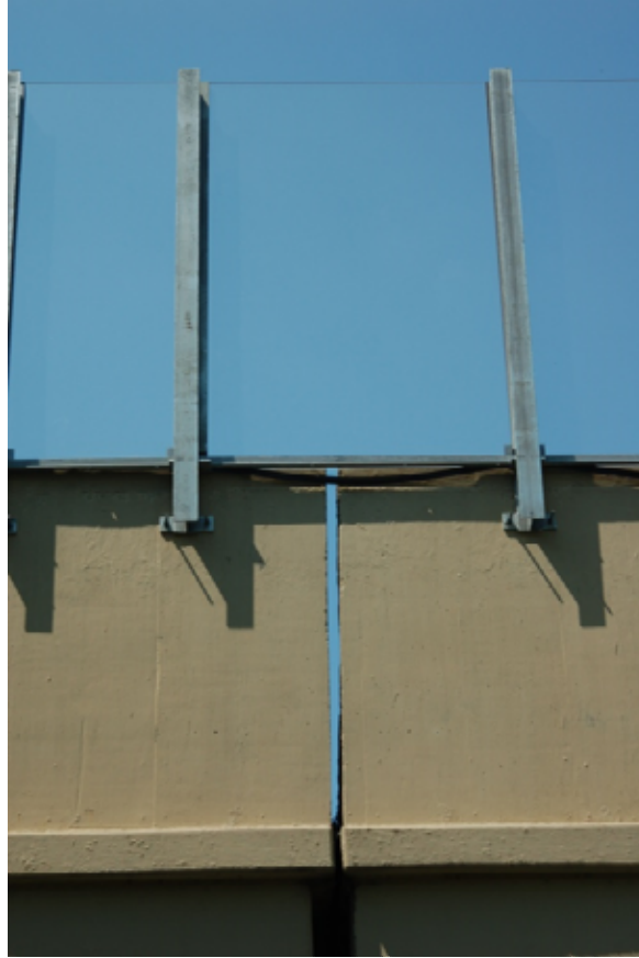
Figure 7.37: Expansion joint opening due to lack of sealant
