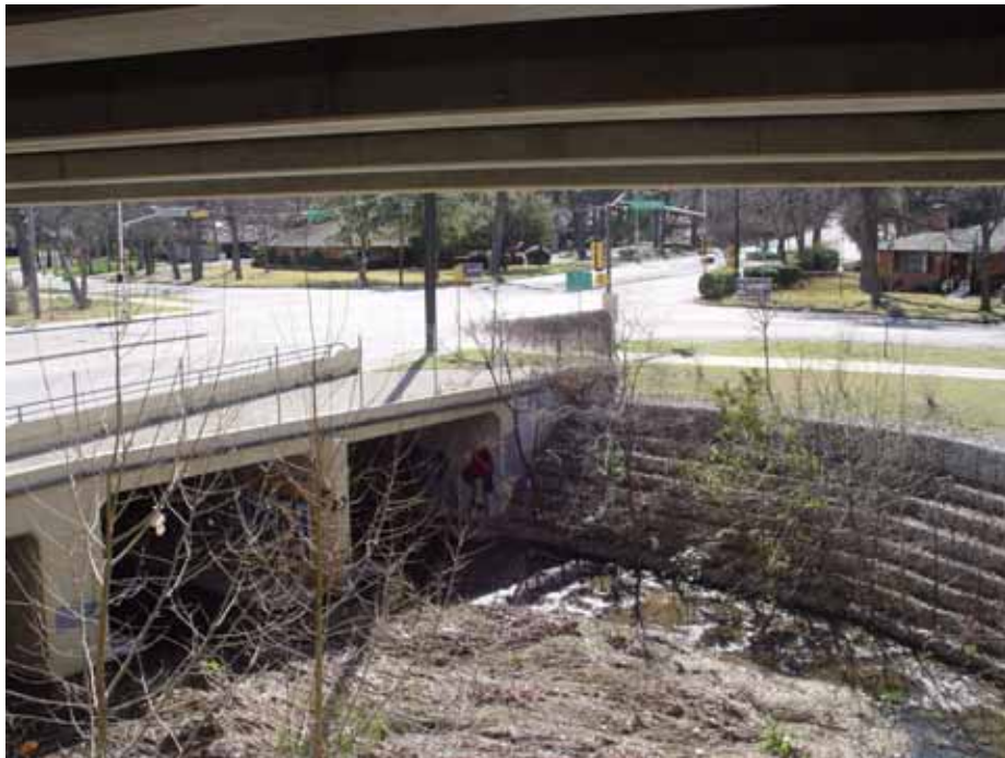
Figure 3.6: Coombs Creek, seen from the Sylvan Avenue underpass (Site 1)
