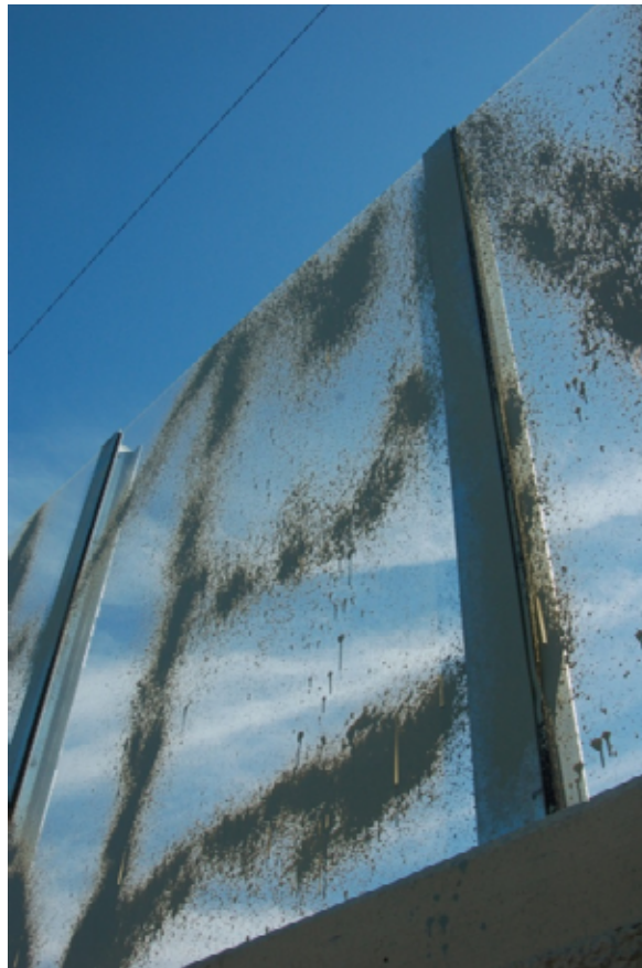
Figure 7.20: Graffiti as seen from the highway shoulder on November 11, 2013
