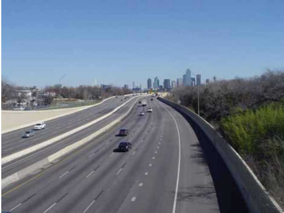
Figure 3.3: View of IH 30 towards the east from Edgfield Avenue Bridge, showing the south-side concrete wall on the right
