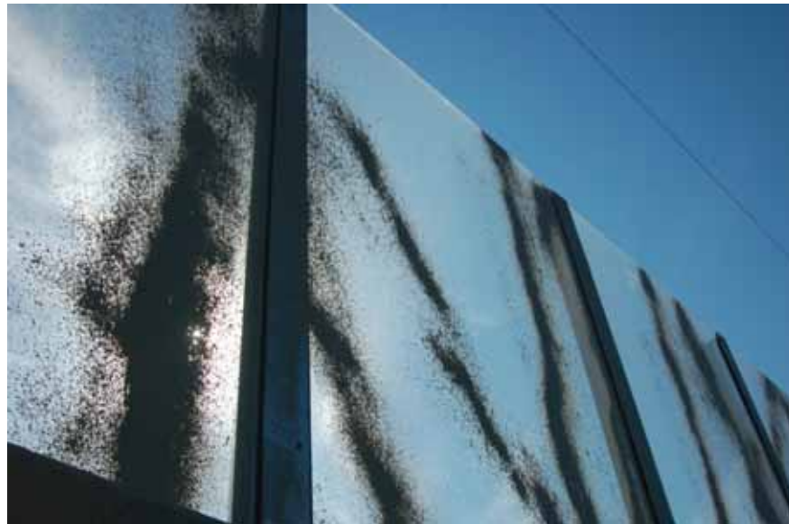
Figure 7.18: Graffiti as seen from the highway shoulder on November 11, 2013
