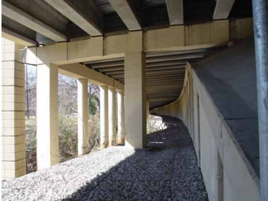
Figure 3.5: IH 30 underside of elevated highway structure, seen from below Sylvan Avenue
