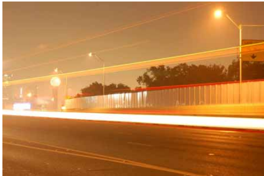
Figure 7.8: Sound wall as seen from westbound lanes looking towards downtown
