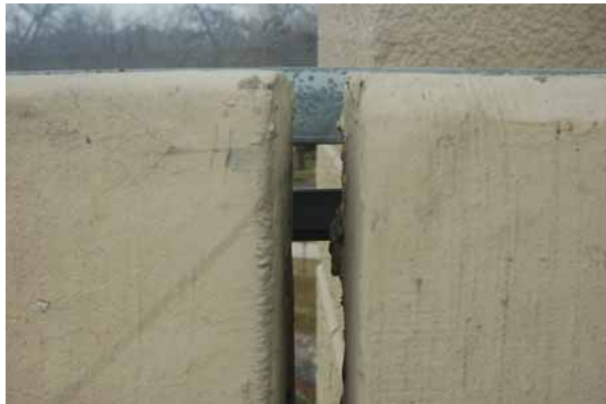
Figure 7.16: Gap in existing concrete wall at bridge expansion joint as seen from the highway side
