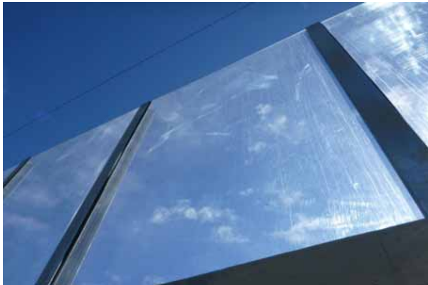
Figure 7.25: Cleaned panel showing traces of the cleaning operation
