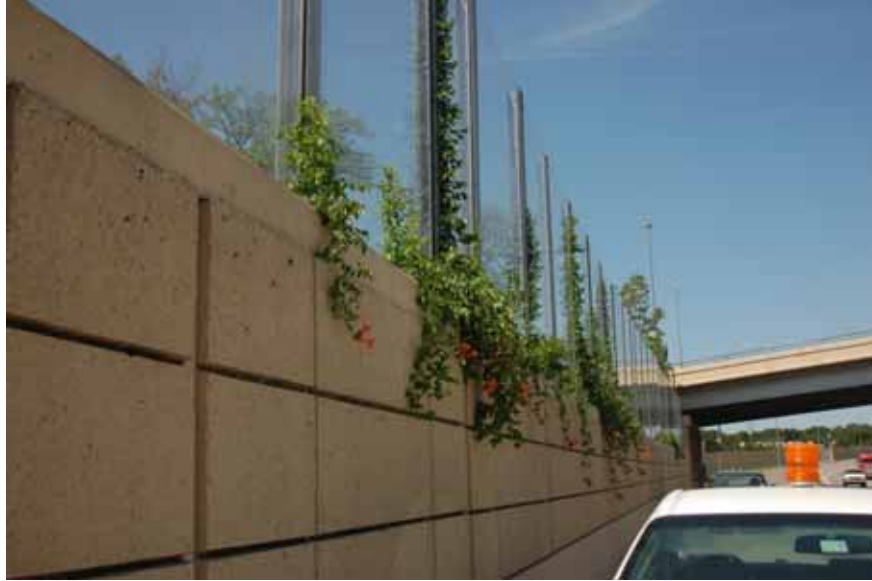
Figure 7.36: Vegetation from the creek side growing through the openings in the gaskets under noise barrier
