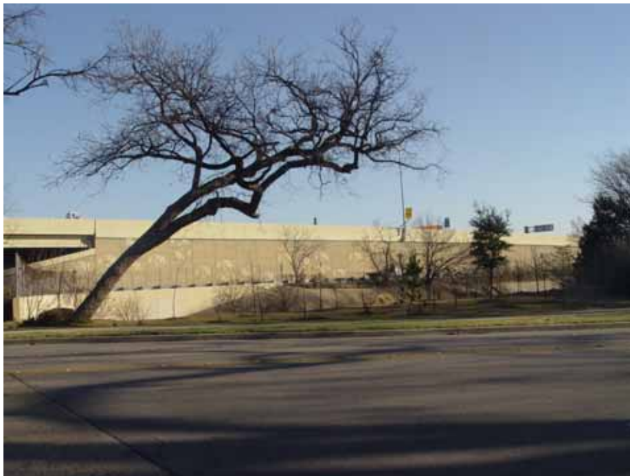
Figure 3.9: South side wall on IH 30 at Site 2
