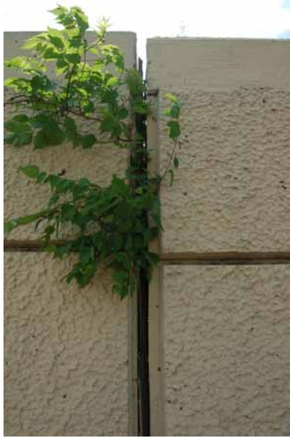
Figure 7.39: Vegetation from the creek side growing through the openings in the concrete structure
