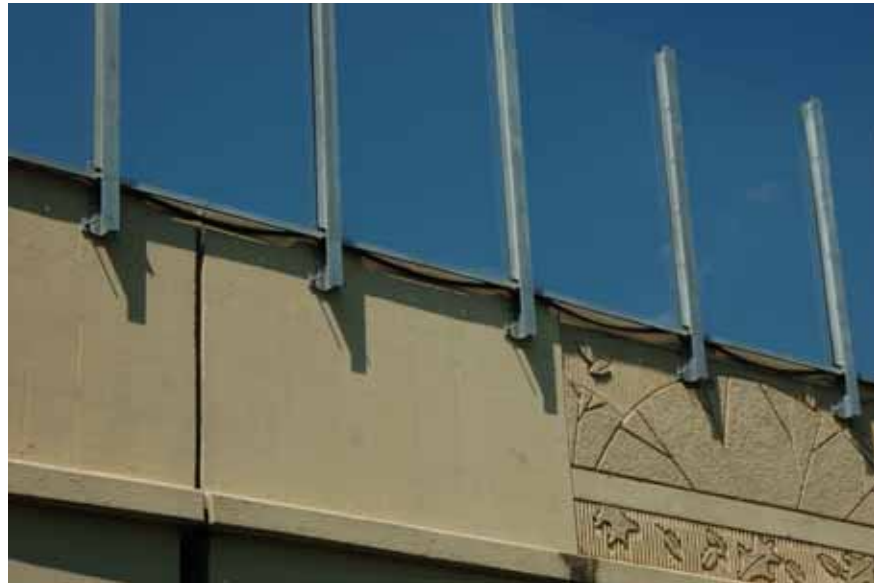
Figure 7.28: Sagging of horizontal rubber gaskets
