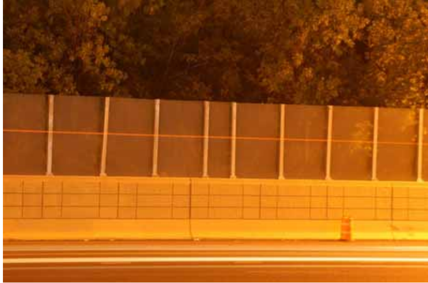
Figure 7.9: Some vertical supports off-plumb
