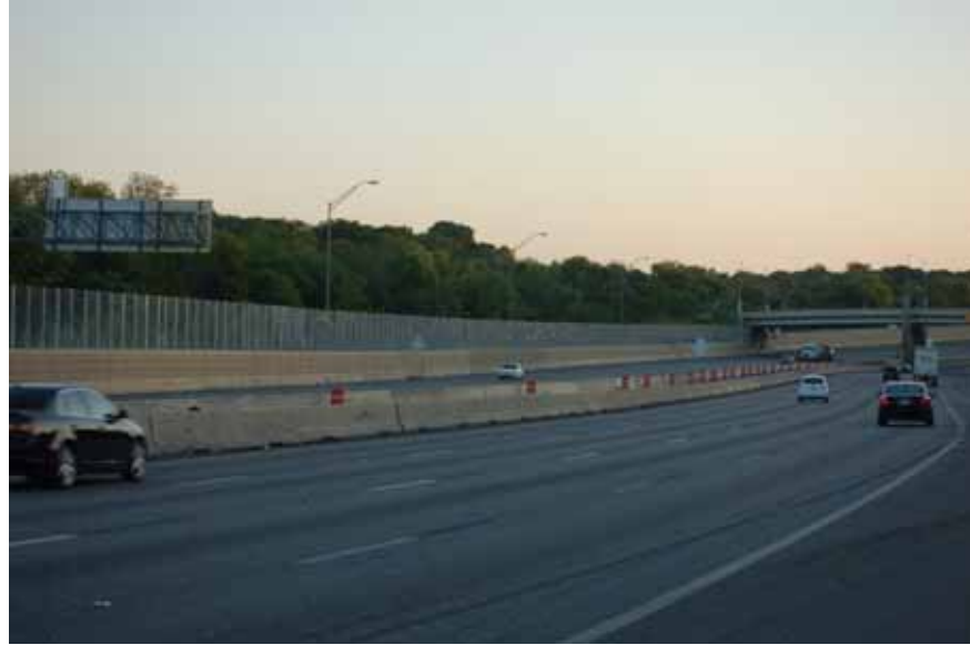
Figure 7.7: Sound wall as seen from westbound IH 30 looking towards Edgefield Avenue Bridge
