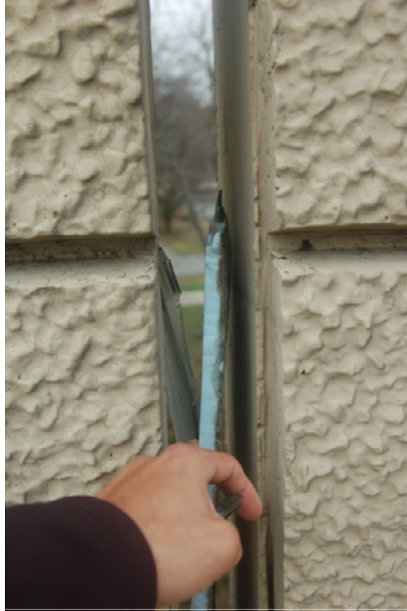
Figure 7.38: Damaged, old sealant material in the expansion joints of bridge structure
