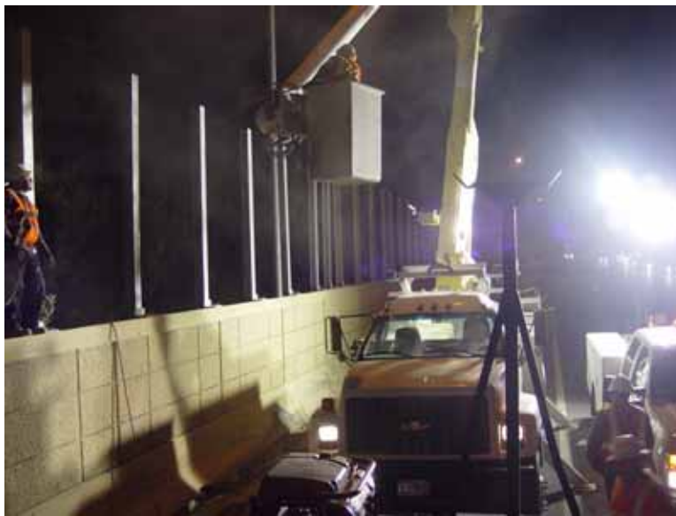
Figure 7.2: Vertical support placement
