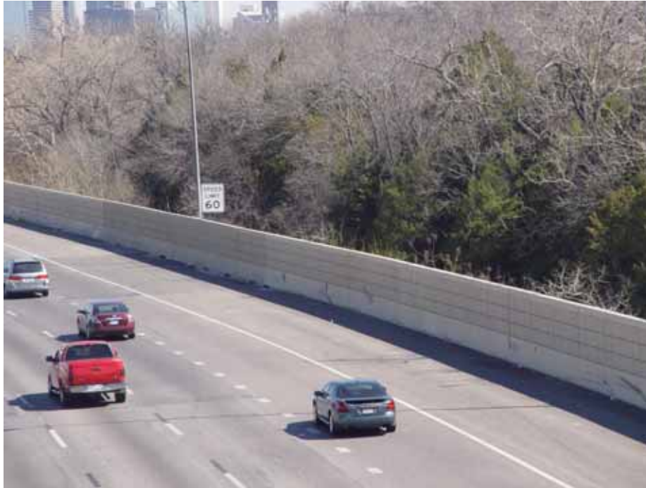
Figure 3.8: South side wall on IH 30 at Site 1
