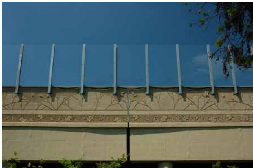
Figure 7.29: Sagging of horizontal rubber gaskets
