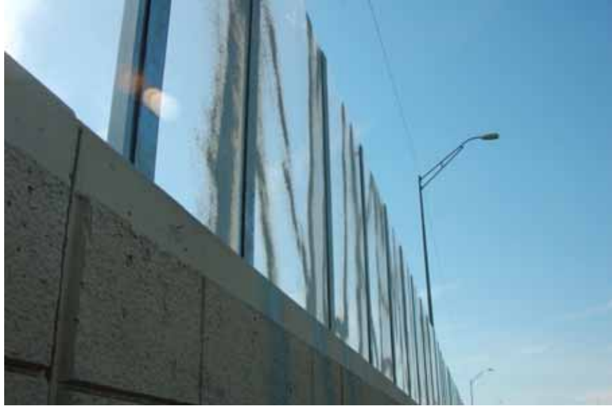
Figure 7.19: Graffiti as seen from the highway shoulder on November 11, 2013. The damage extends to the concrete wall under span #144.
