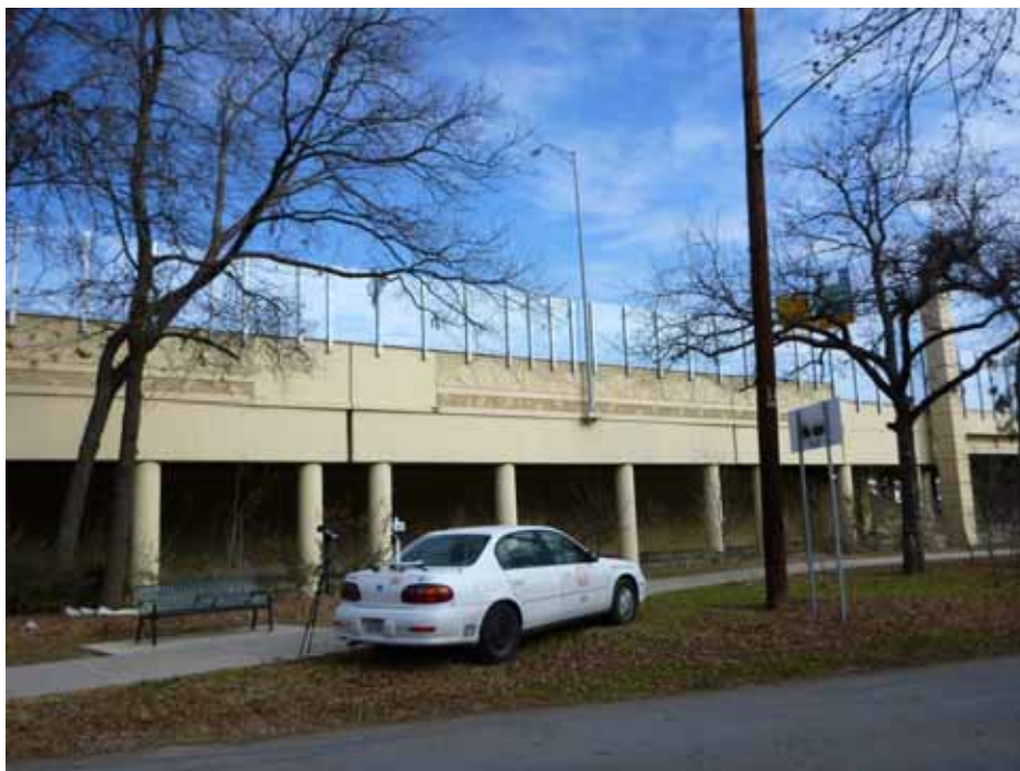
Figure 5.20: Noise measurement at Coombs Creek Trail Park (Location B) after noise barrier installation
