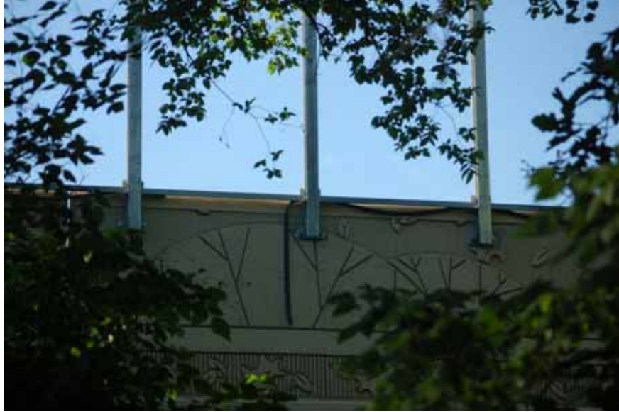
Figure 7.34: Broken horizontal rubber gasket
