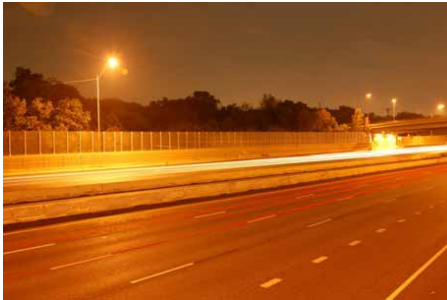
Figure 7.6: Sound wall as seen from westbound IH 30
