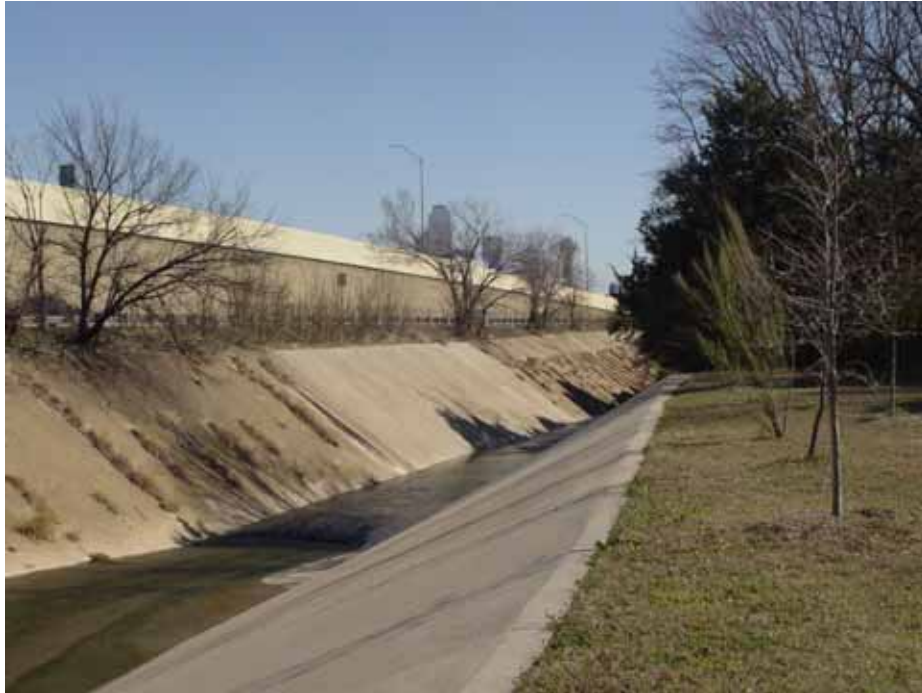
Figure 3.7: Coombs Creek, east of Sylvan Ave (Site 2); elevated highway structure in the background
