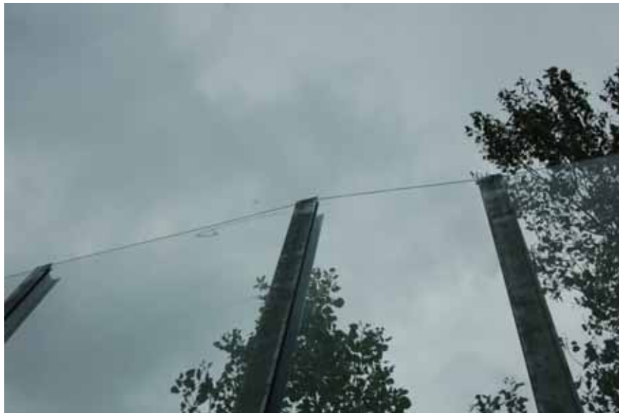
Figure 7.10: Vertical support off-plumb
