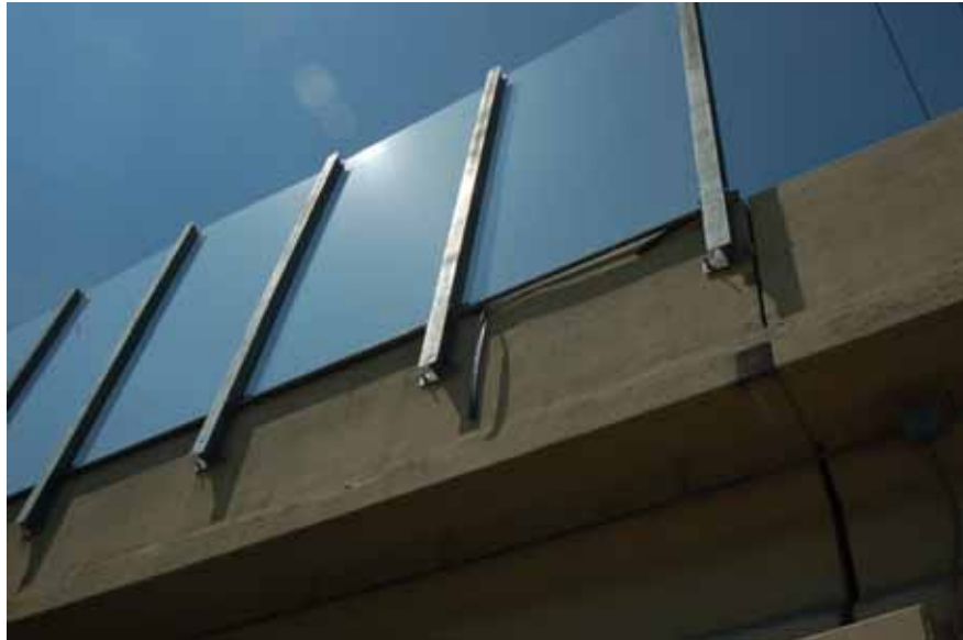
Figure 7.33: Broken horizontal rubber gasket
