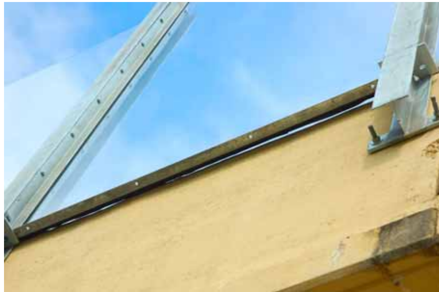
Figure 7.13: Gap between horizontal gasket and metal support
