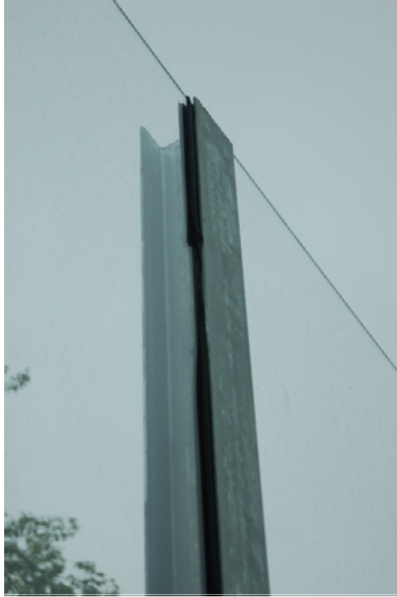
Figure 7.11: Gasket shown protruding from metal support
