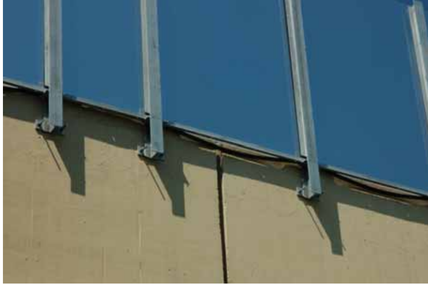
Figure 7.30: Sagging of horizontal rubber gaskets
