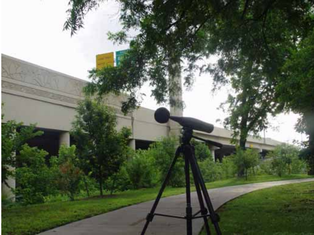
Figure 5.19: Noise measurement at Coombs Creek Trail Park (Location B) prior to noise barrier installation
