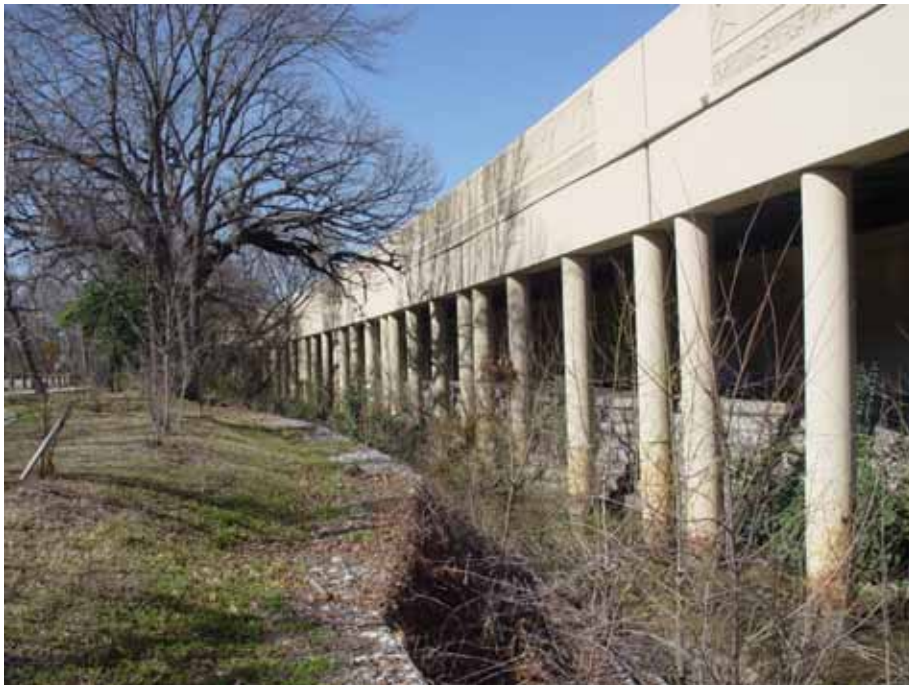
Figure 3.4: IH-30 elevated highway structure and concrete wall, seen from Coombs Creek (Site 1)
