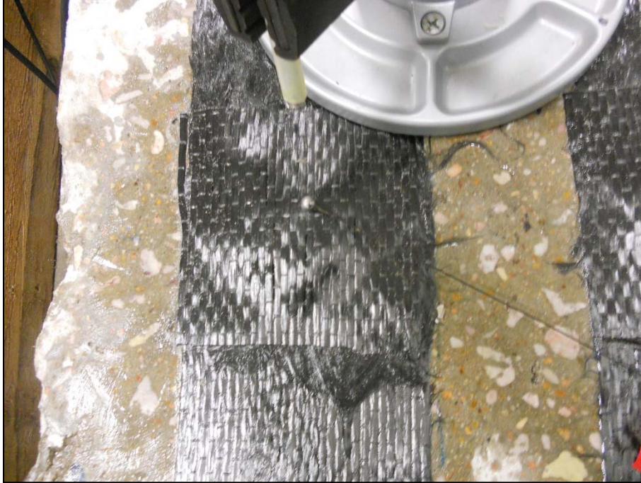
Figure 7-9: Anchor defect detection using the sounding method
