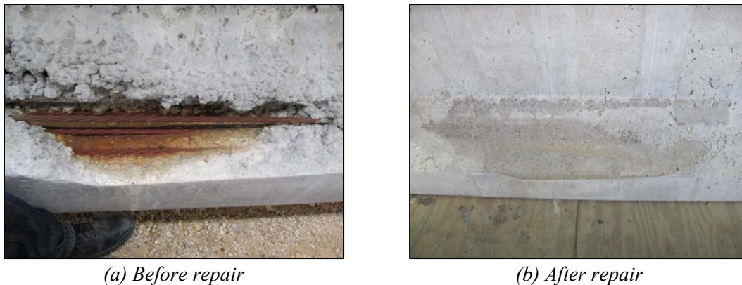
Figure 4-1: Honeycomb repair
