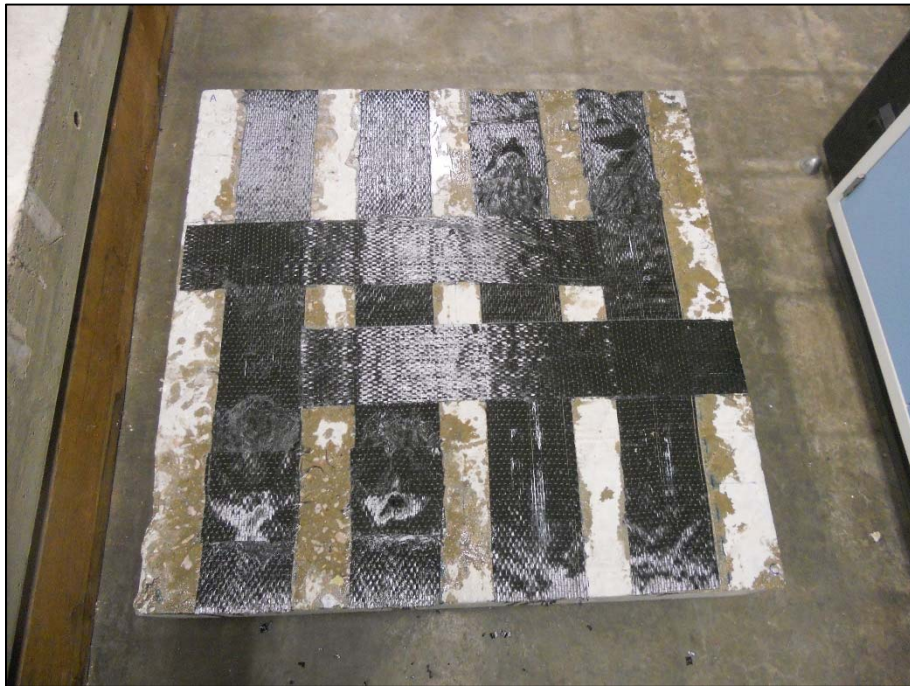
Figure 7-8: Concrete slab after installation of CFRP strips and anchors
