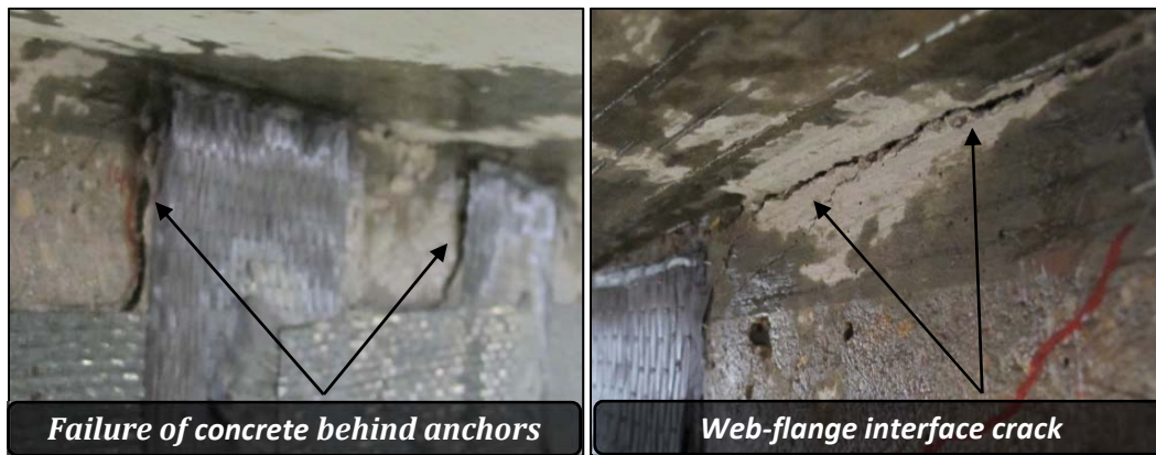
Figure 3-28: Flange-web crack interface (24-3-8-3)
