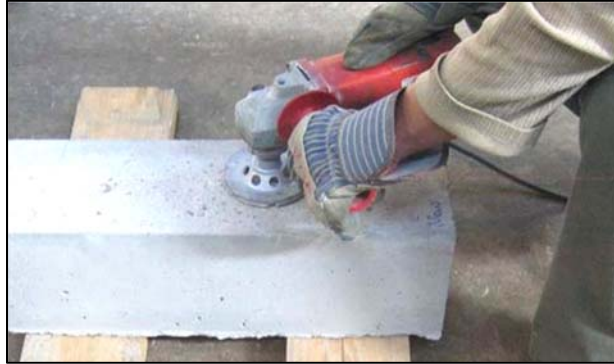
(a) Grinding a concrete surface
