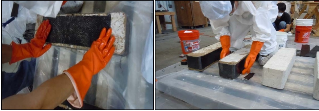
Figure 6-11: Applying CFRP strips
