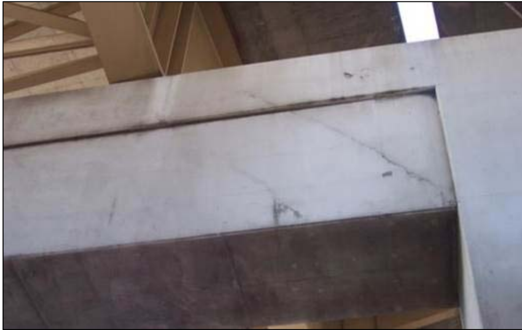
Figure 5-1: Shear crack in pile cap girder
