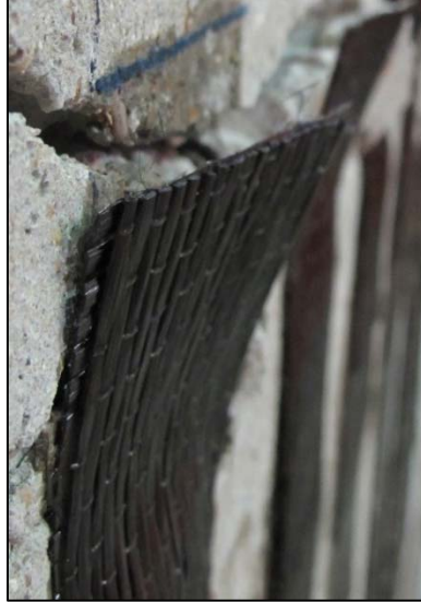
Figure 5-27: CFRP anchor post-failure
