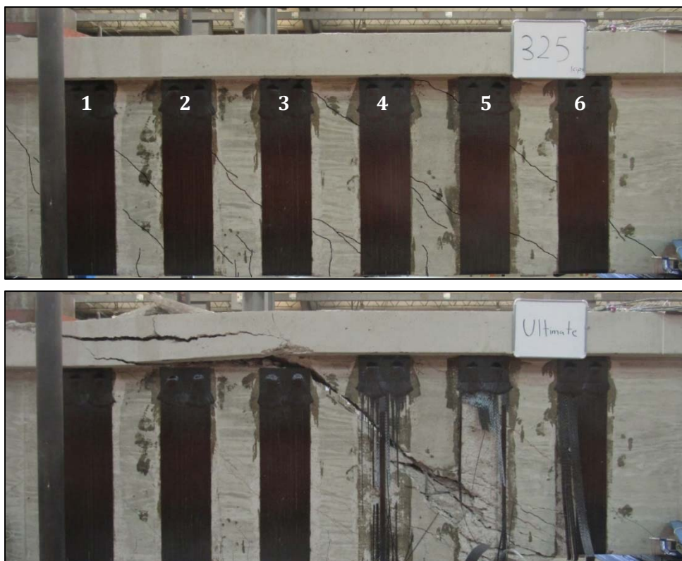
Figure 3-58: Test 48-3-14-7 before (top) and after (bottom) failure [west side]
