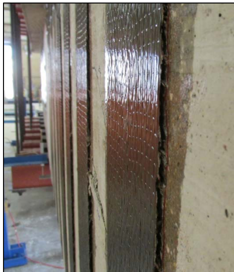
Figure 3-47: Debonding of strips in 48-3-14-3
