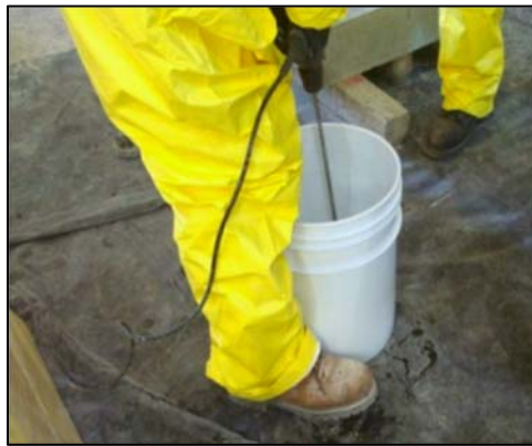
Figure 6-9: Mixing the epoxy components (Huaco, 2009)
