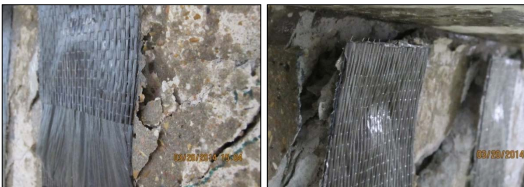
Figure 3-26: Concrete crushing behind anchors (24-3-8-2)
