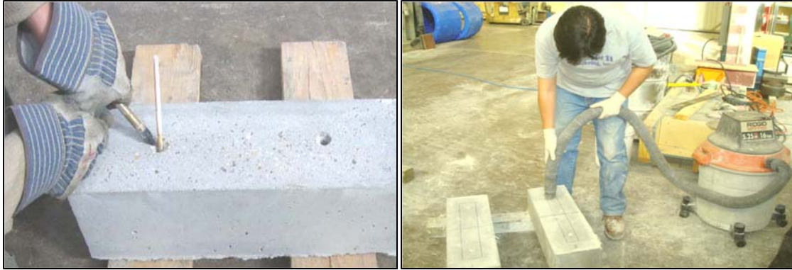
(d) Cleaning holes with compressed air or vacuum cleaner Figure 6-6: Specimen preparation before CFRP installation
