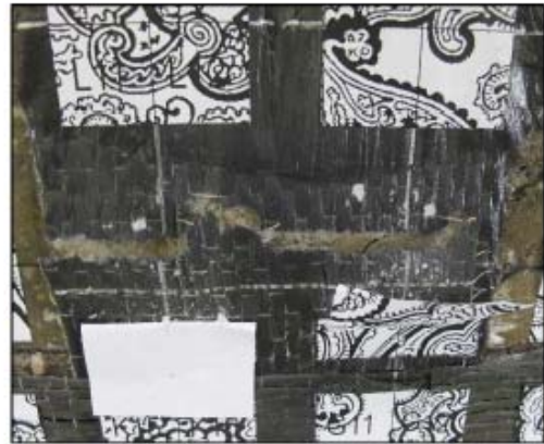
(c) Strip 6 fracture (east side)
