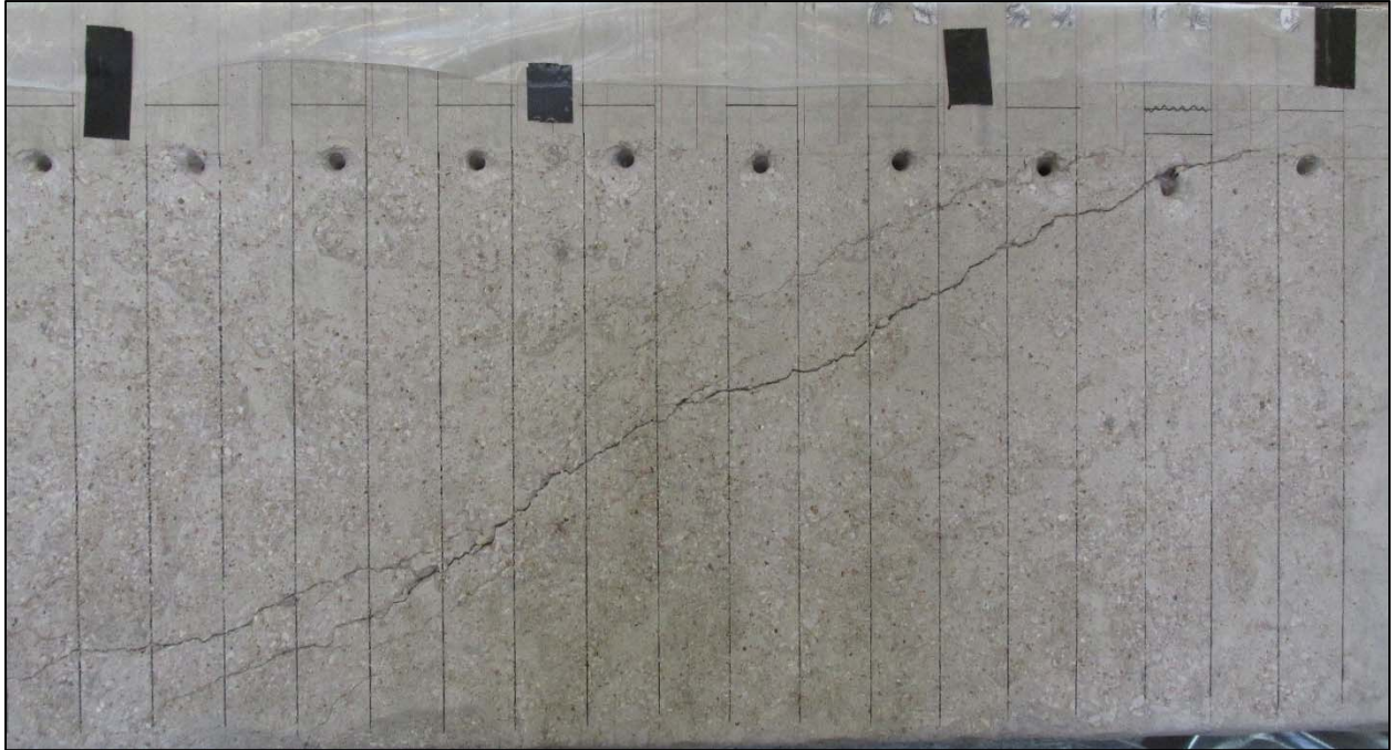
Figure 5-18: S-C-VA-HN crack pattern prior to CFRP installation
