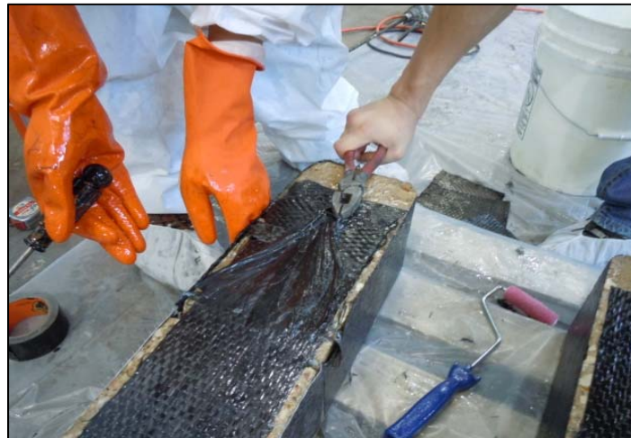
Figure 6-12: Fanning the anchor
