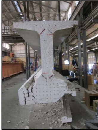
(a) Reaction end of beam (Cut at mid-section of 100-ft. beam)
