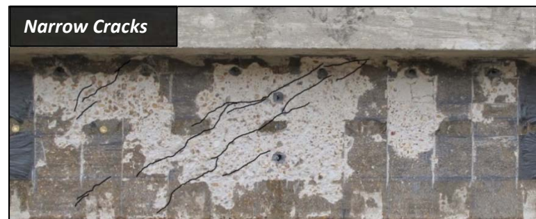
(c) 24-3-14-1 (after strips removed)
