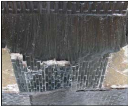
(b) Strip 6 fracture (west side)
