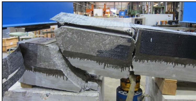
Figure 6-26: Beam specimen failure
