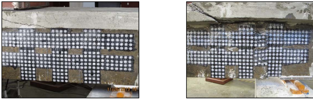
(b) Concrete Crushing Failure
