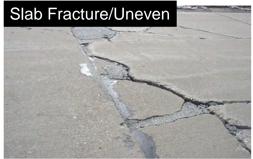
Extreme fatigue cracking/unstable base
