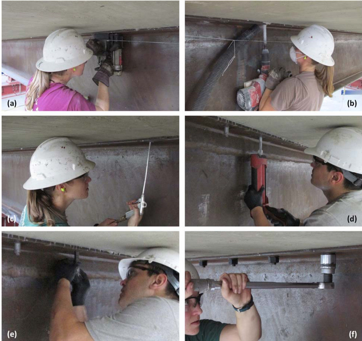
Figure 8.3 Connector Installation
