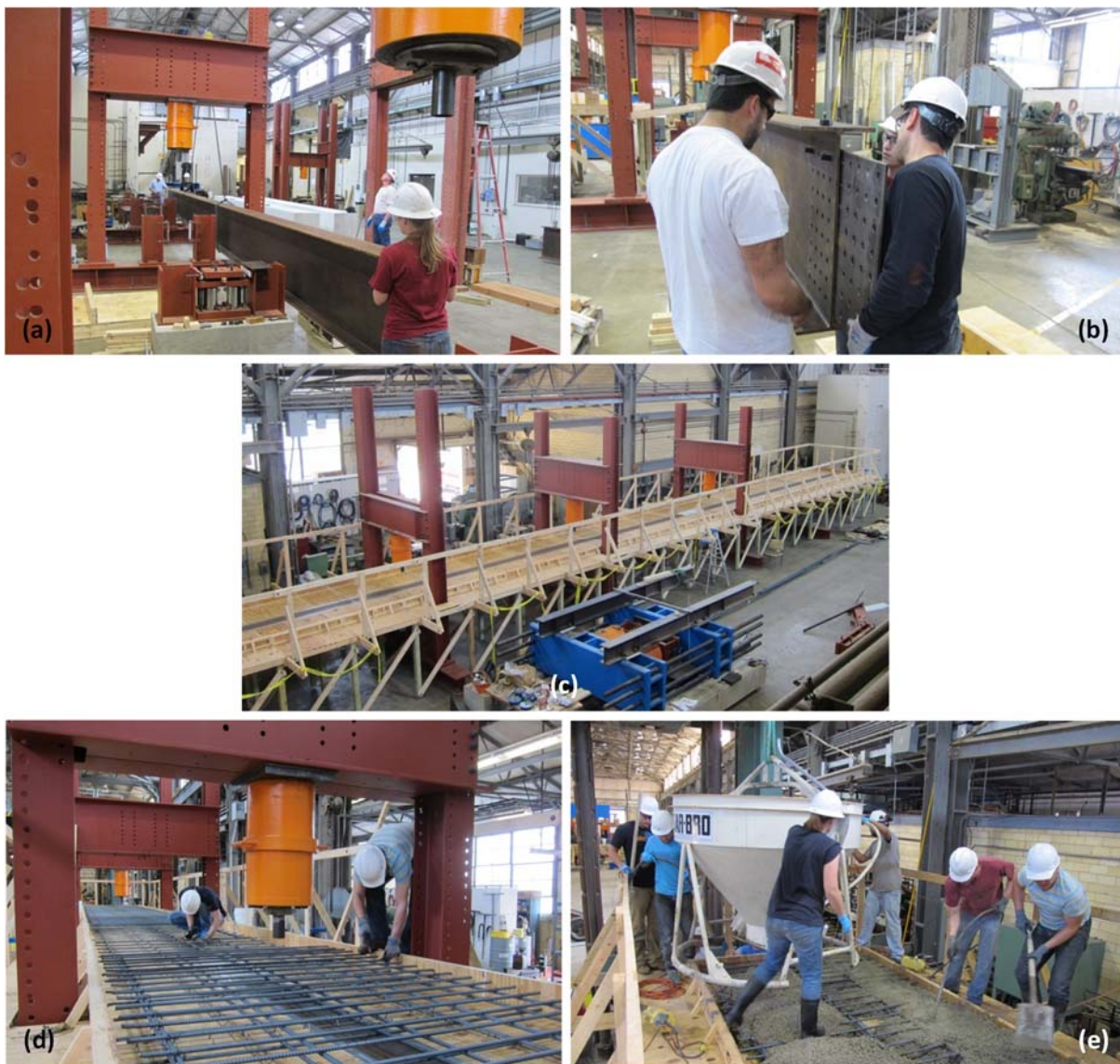
Figure 6.3 Specimen Construction – (a) Steel erection, (b) Splice plates, (c) Deck formwork, (d) Deck reinforcement, and (e) Deck casting
