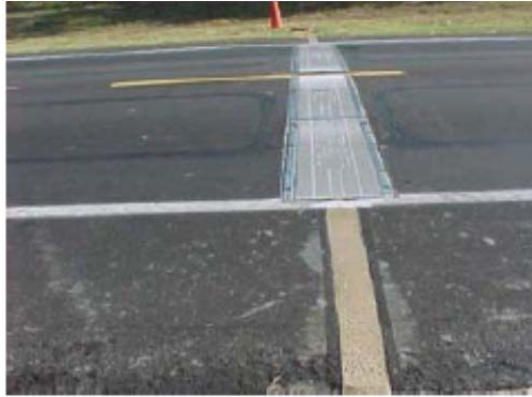
Figure 3.4: Bending Plates for WIM systems (Florida DOT, 2007)
