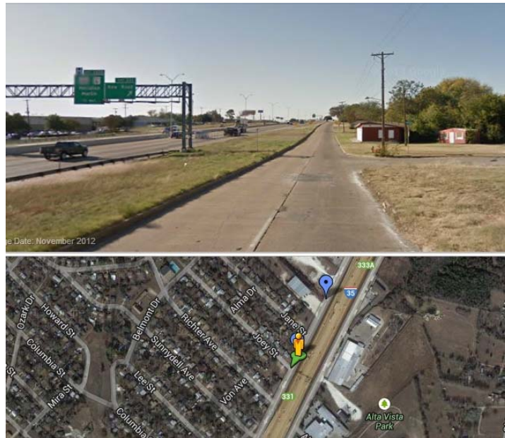
Figure 2.21: Picture and Aerial View of IH35-2
