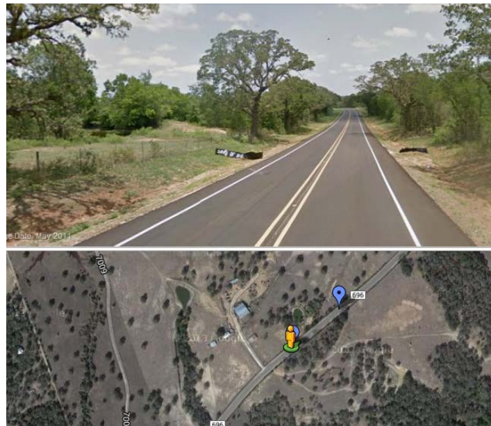
Figure 2.6: Picture and Aerial View of FM696-3
