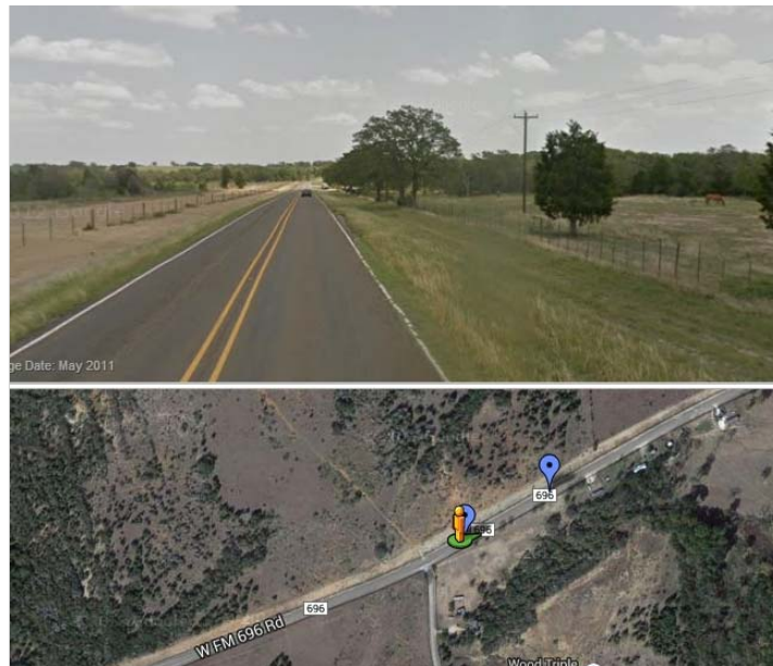
Figure 2.4: Picture and Aerial View of FM696-1
