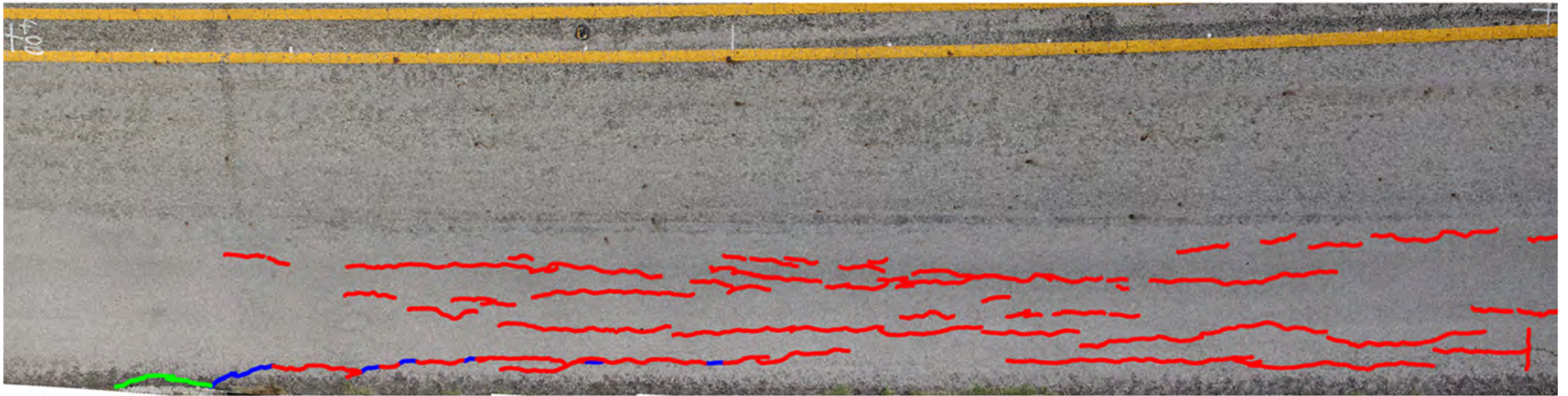
Manual Crack Map
