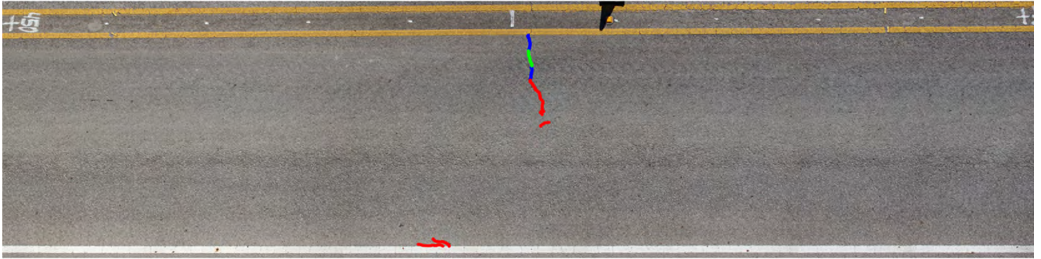
Manual Crack Map
