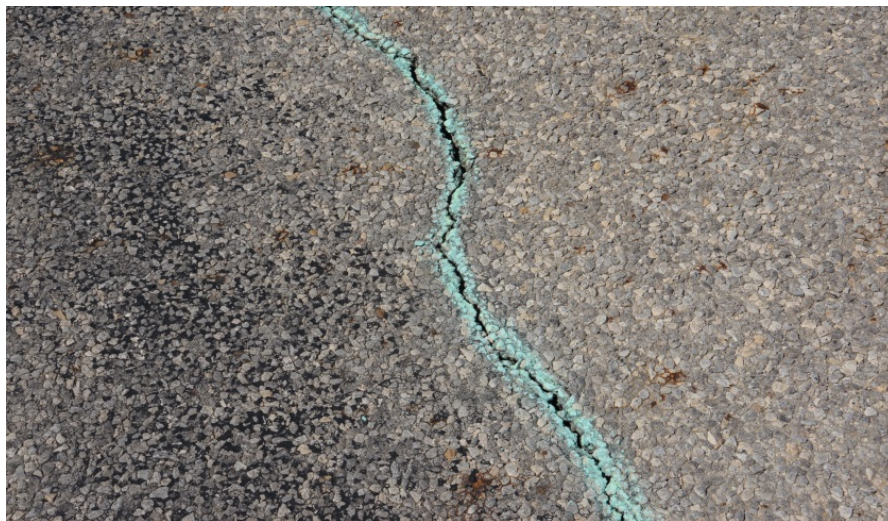
Figure 2.36: Crack Marked in Green (>6mm Width) on FM 1331-1
