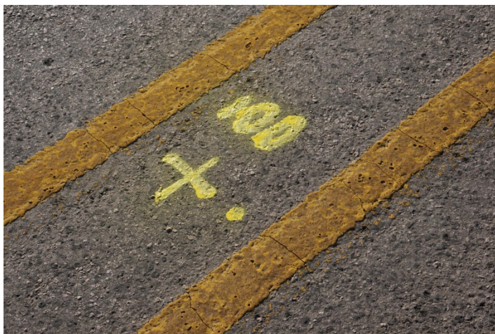
Figure 2.26: Special Marking to Indicate 50-ft Increments from the Beginning of the Test Section
