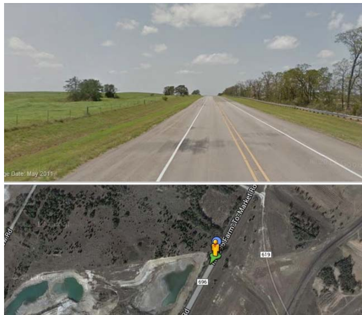
Figure 2.8: Picture and Aerial View of FM696-5
