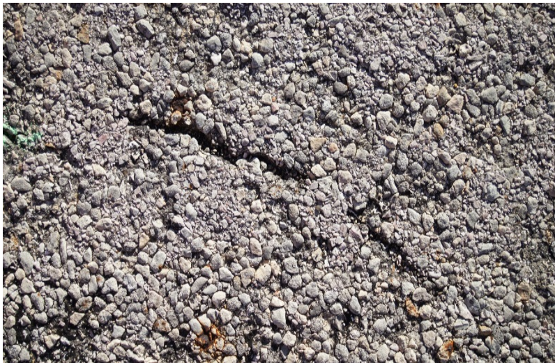
Figure 2.38: Phantom Cracks Created by Loss of Aggregates on FM 1063
