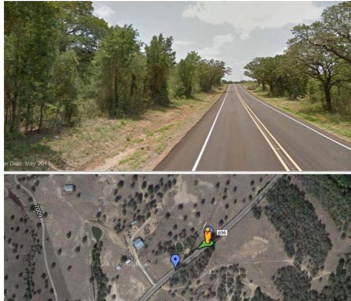
Figure 2.7: Picture and Aerial View of FM696-4
