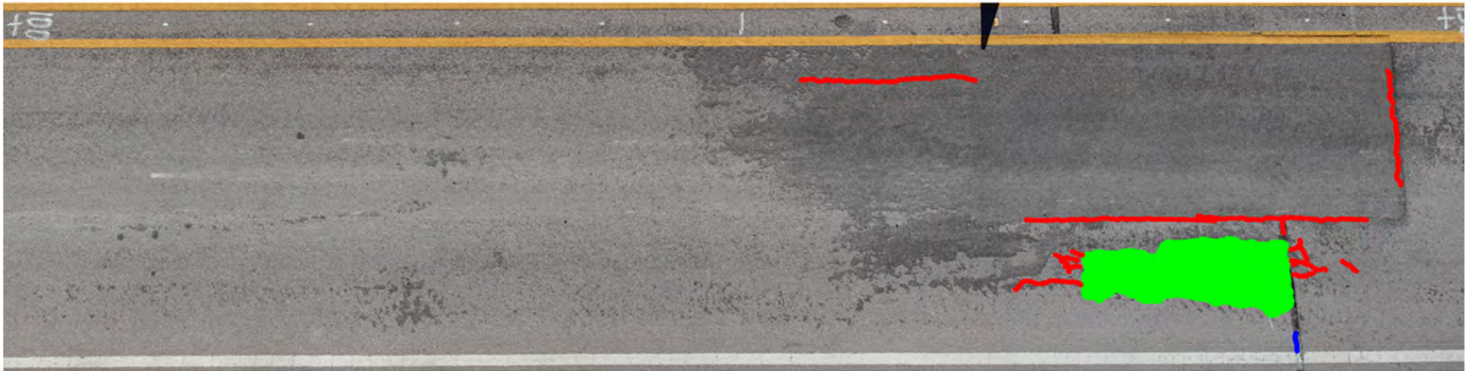
Manual Crack Map
