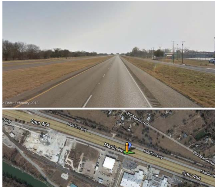
Figure 2.17: Picture and Aerial View of Spur484-1
