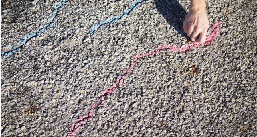
Figure 2.35: Cracks Marked with Chalk in Different Colors according to Crack Width, (Red < 3mm, Blue 3–6mm) on FM 1063
