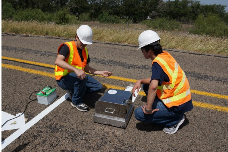
Figure 2.28: Placement of CTM, Inside Wheel Path
