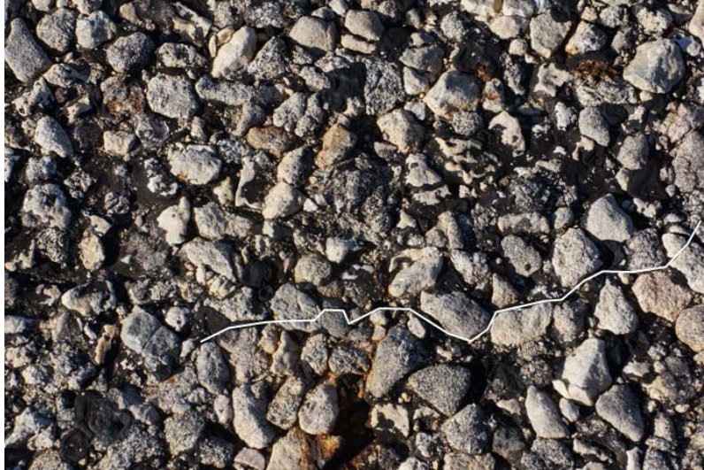
Figure 2.37: Phantom Cracks Marked in White on FM 1063
