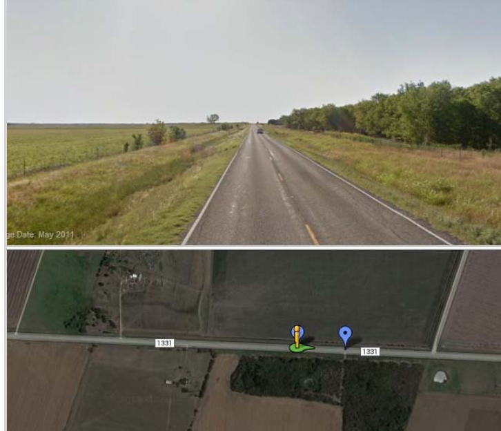
Figure 2.11: Picture and Aerial View of FM1331-2
