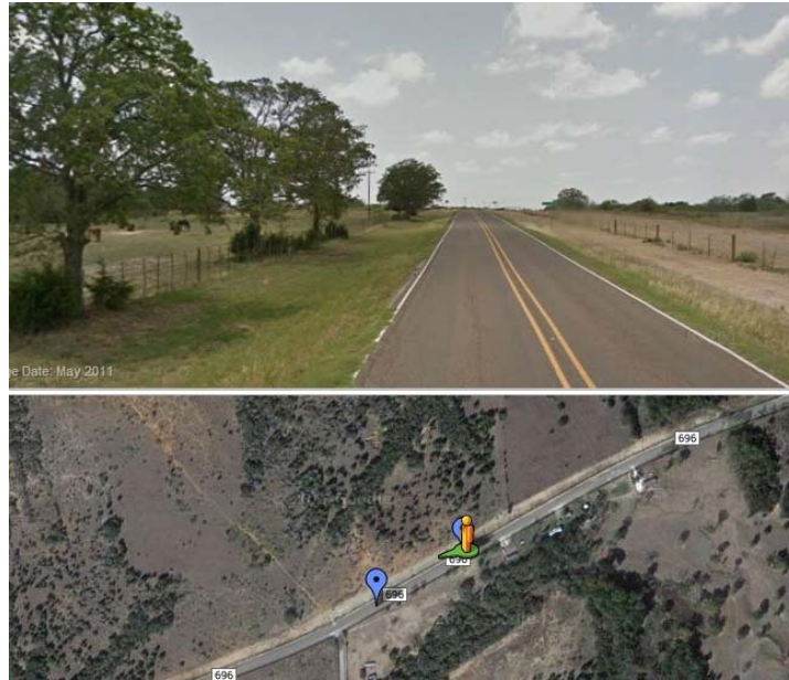
Figure 2.5: Picture and Aerial View of FM696-2
