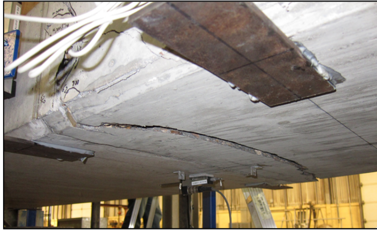
Figure 5.14: Differential displacement at the splice region of Test Girder 1
