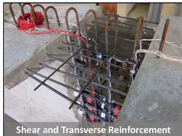
Figure 4.18: Splicing procedure – (a) concrete pedestals; (b) placing girder segments; (c) verifying girder placement; (d) coupling ducts; (e) spliced interface reinforcement; (f) shear and transverse reinforcement
