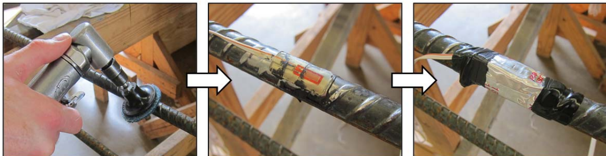
Figure 4.26: Strain gauge installation procedure
