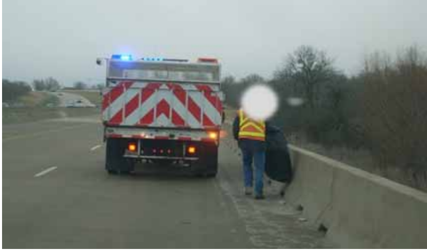
Figure 22: Work Procedures of Observation 13
