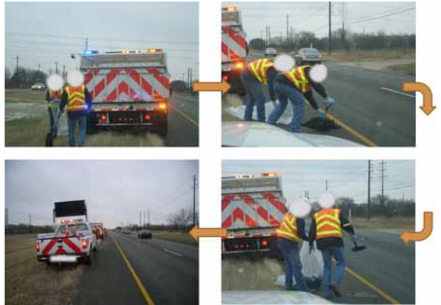
Figure 9: Work Procedures of Observation 1
