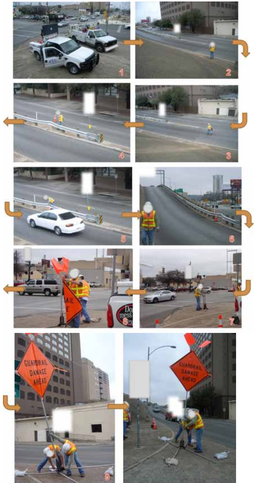
Figure 12: Work Procedures of Observation 3
