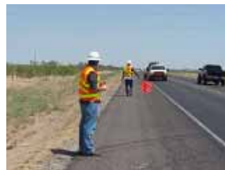
Figure 17: Traffic Control Devices Used in This Operation
