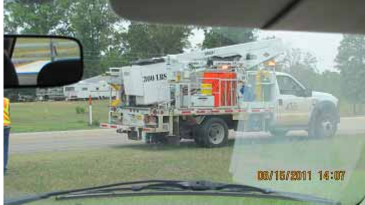
Figure 38: The Other Side of Truck Used for Installing Signs
