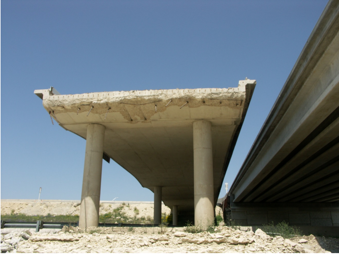
Figure 10.10: Left: Original Bridge over IH 35 at Amity Road; Right: Replacement Bridge
