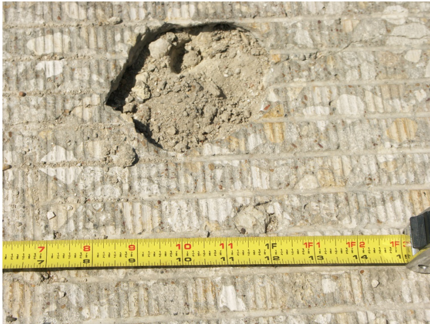
Figure 10.2: Popout in Pavement Surface
