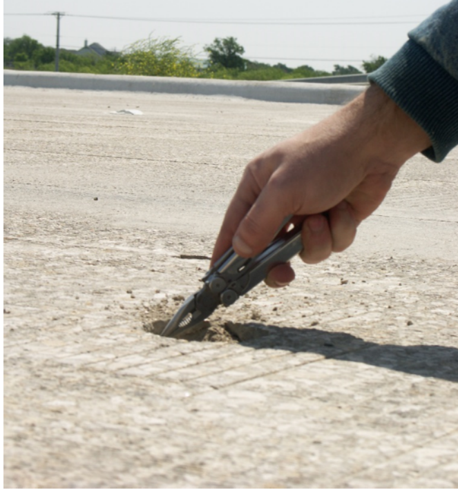
Figure 10.4: Removing Loose Material from Popout
