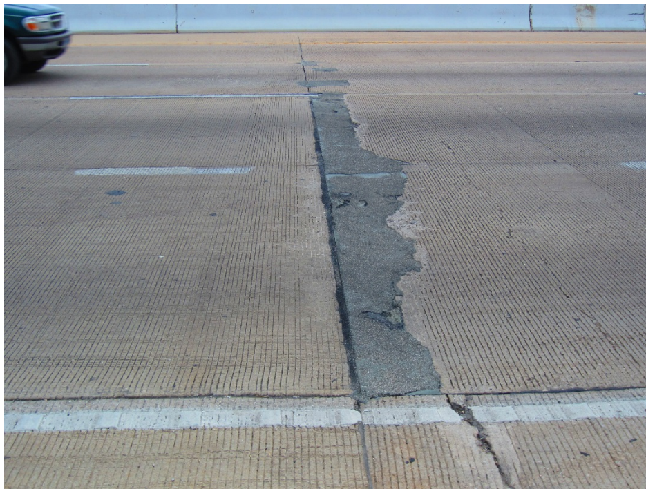
Figure 10.1: Pavement Cracking and Spalling on Texas 183
