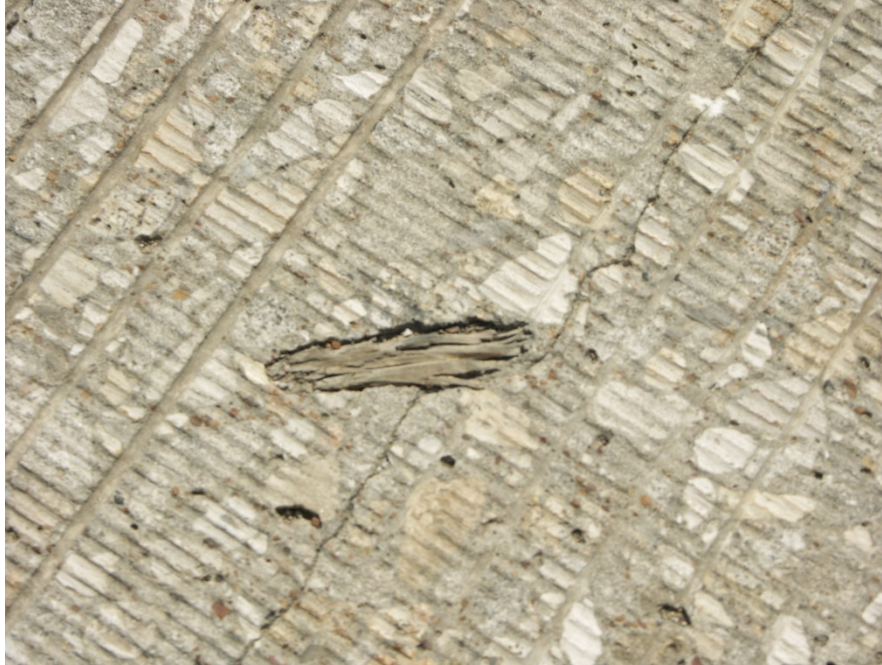
Figure 10.3 Deleterious Material in Pavement Surface
