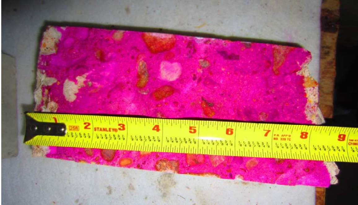
Figure 10.13: Phenolphthalein Staining of Amity Bridge Concrete
