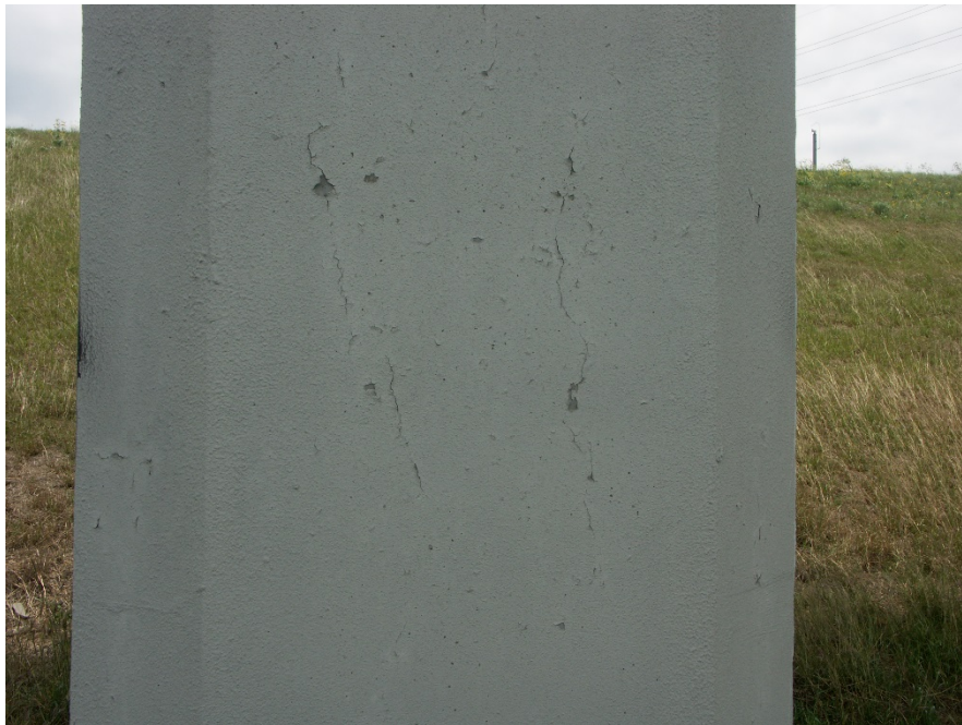
Figure 10.8: Column Cracking as Seen from Roadway
