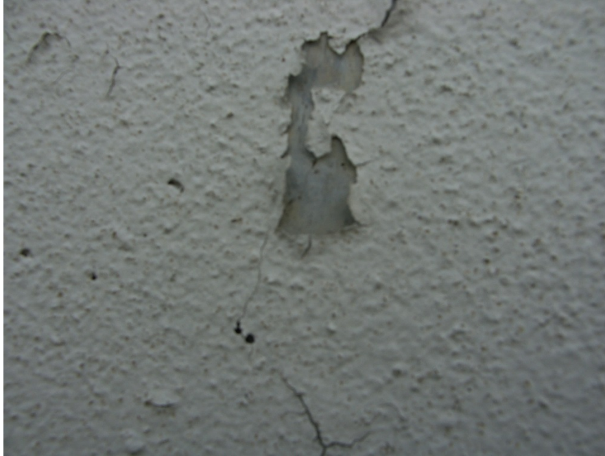
Figure 10.9: Close-up of Column Cracking
