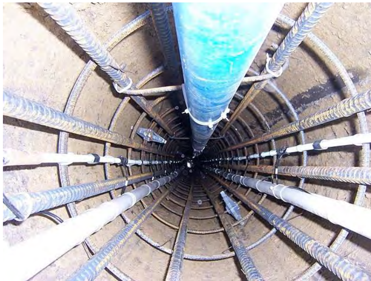
Figure E.22: Connections for inclinometer casings in instrumented shafts.
