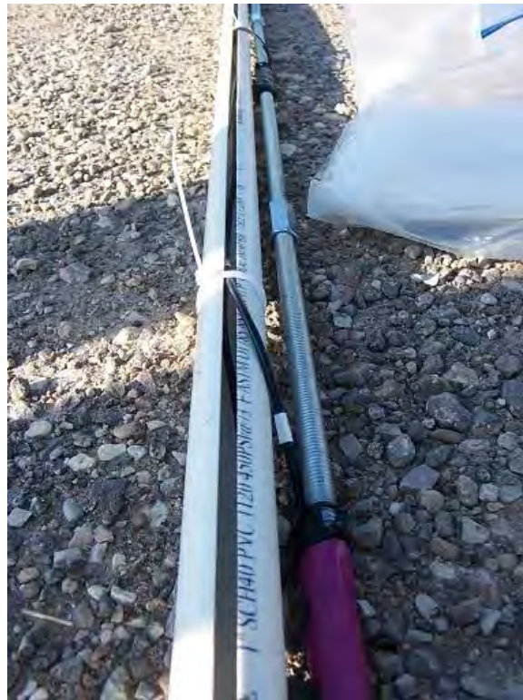
Figure E.15: Attaching slotted PVC pipe to sister bars with zip ties.
