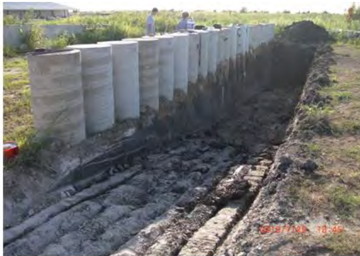
Figure E.35: Excavation process as of 7/29/2010.
