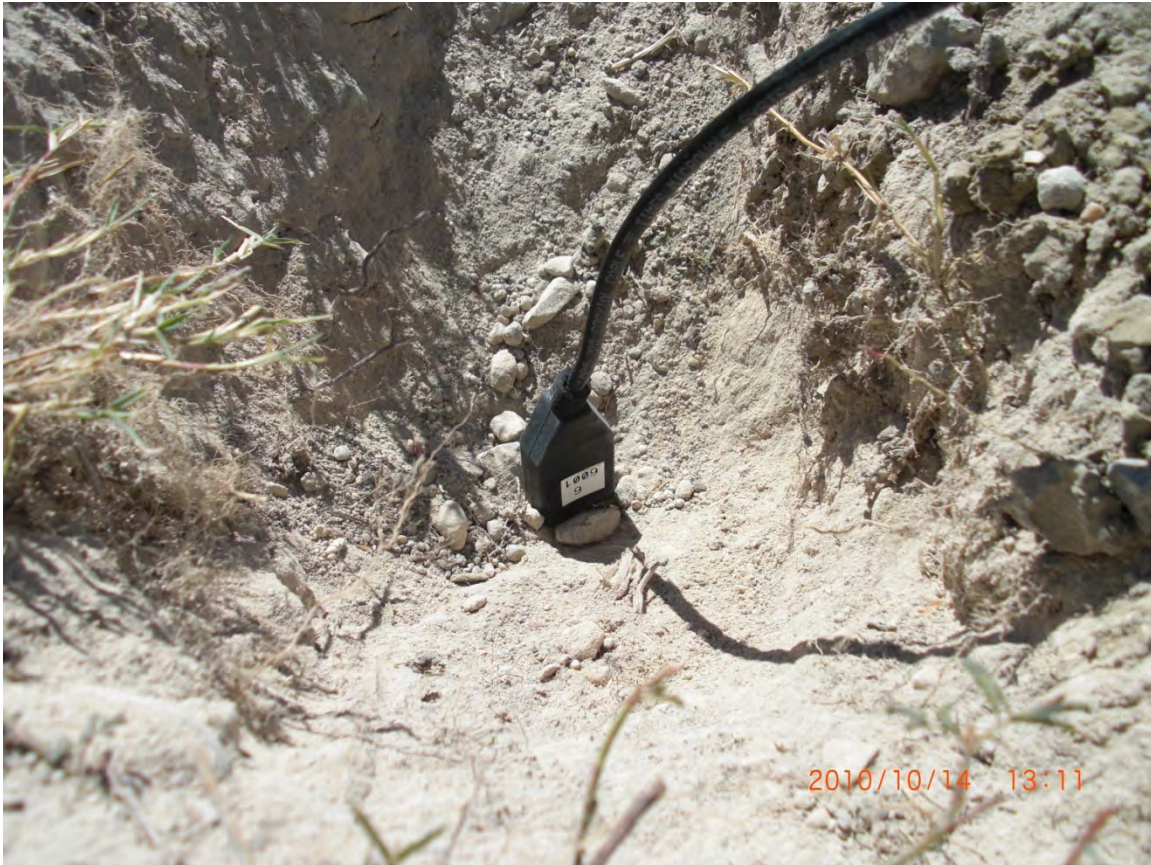
Figure 5.6: A sample probe installation from the ground surface.
