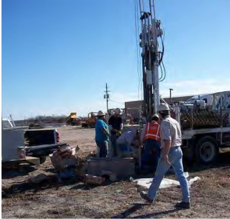
Figure E.24: The piezometer installed in borehole B-3 being lowered into position.
