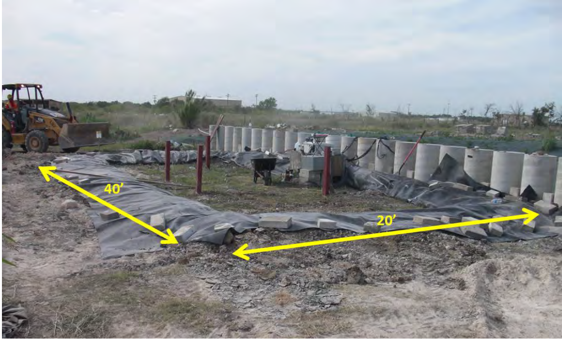
Figure E.50: Completed inundation berm.
