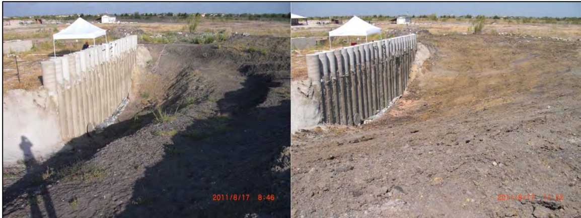
Figure 6.5: Excavation slopes are reshaped on August 17, 2011.
