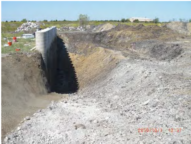
Figure E.41: Excavation process as of 10/1/2010.
