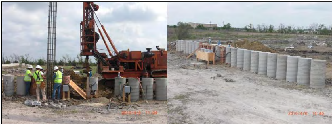
Figure 3.10: Construction of test wall, April 2010.
