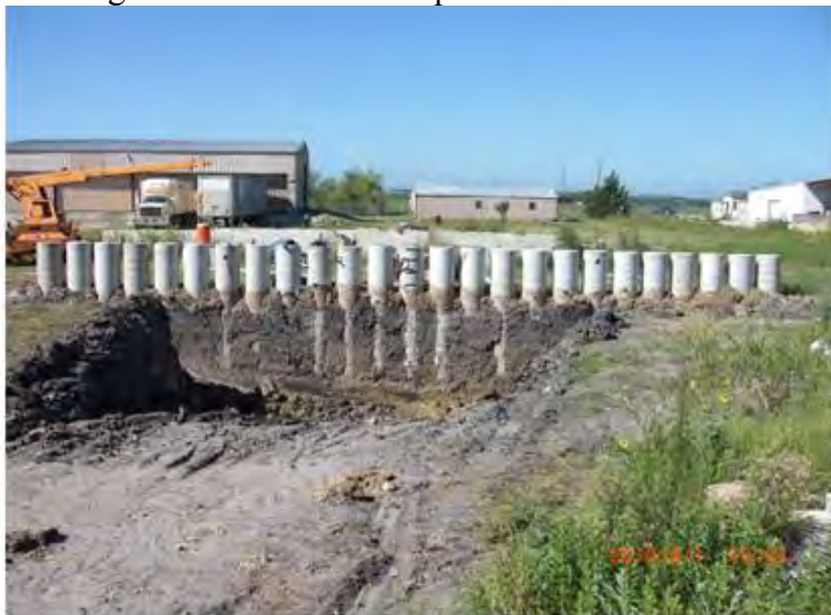
Figure E.37: Excavation process as of 8/1/2010.
