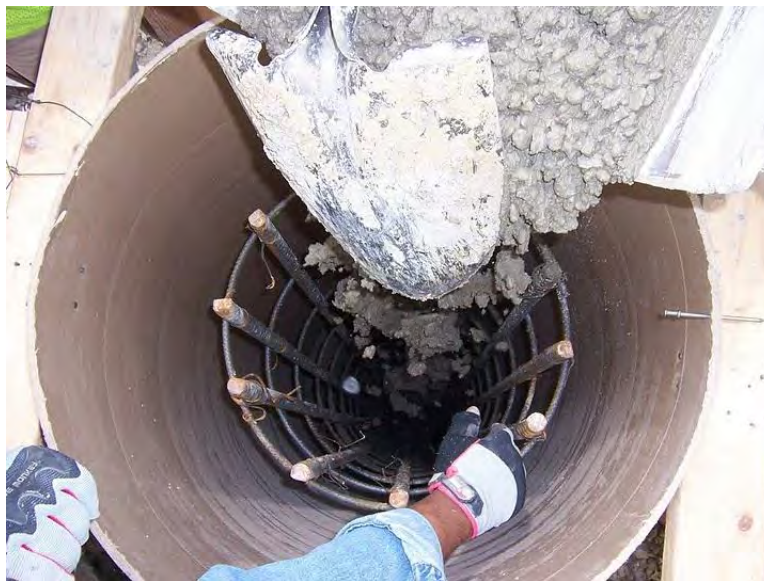
Figure E.10: Free fall method for pouring concrete.
