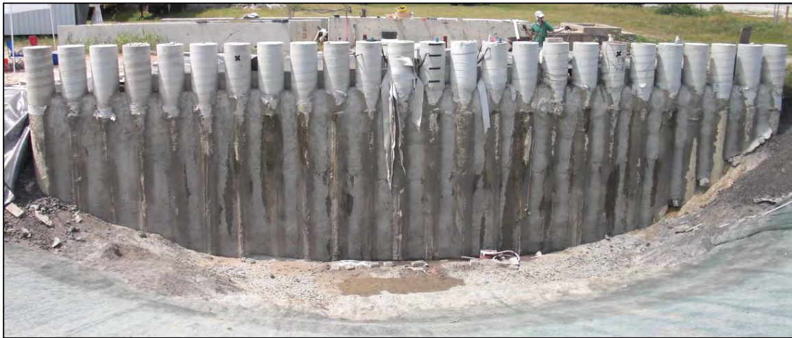
Figure 7.37: Water infiltration into the excavation was first observed 90 minutes from the start of inundation.
