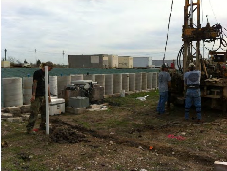
Figure E.26: Piezometer being installed in borehole A.
