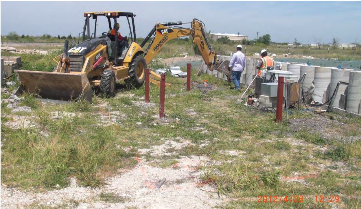
Figure E.45: Excavation of trench for inundation berm.
