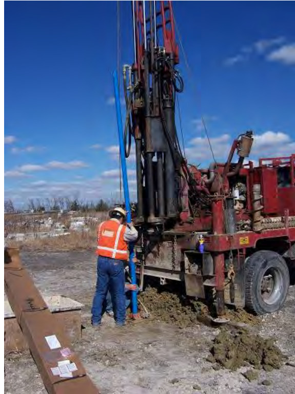
Figure E.20: Installation of the inclinometer casing in borehole B-2.
