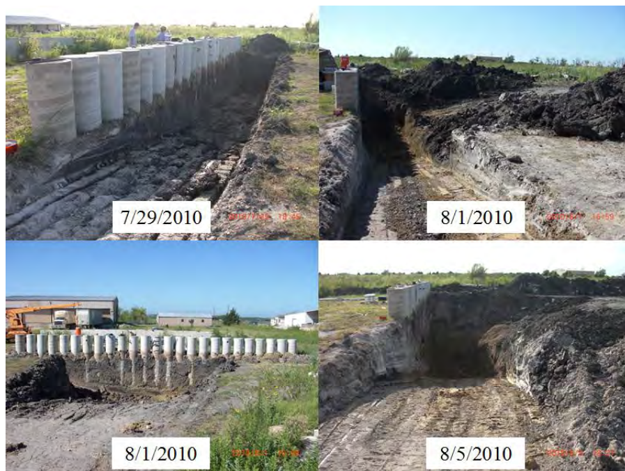
Figure 5.1: Photos of initial excavation progress (7/29/2010 – 8/5/2010).
