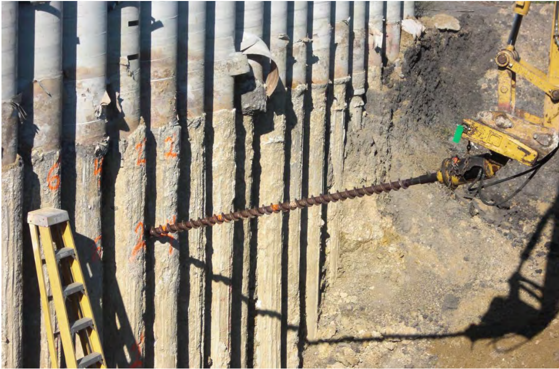
Figure 5.4: A hole being drilled by Craig Olden, Inc
