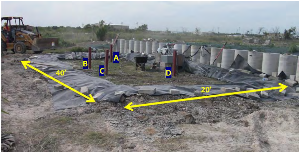
Figure E.27: The four standpipe piezometers installed behind the wall in the inundation berm.
