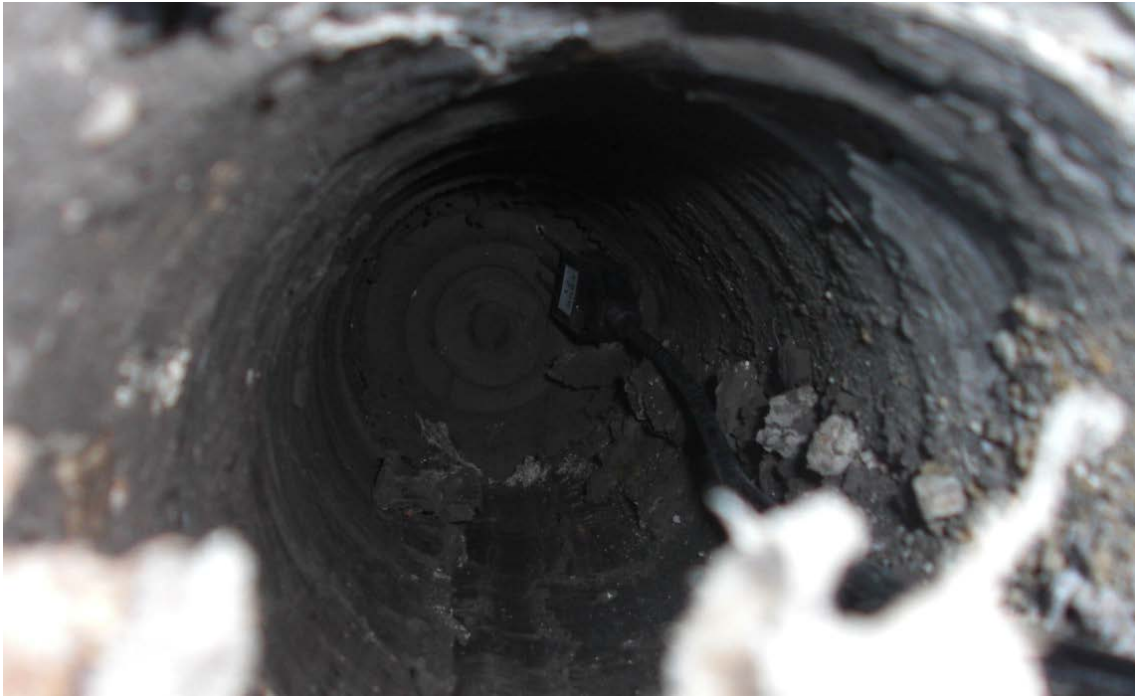
Figure 5.7: A sample probe installation where the probe could not be pushed completely into the soil
