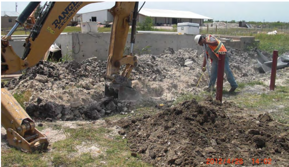
Figure E.47: Compacting soil with backhoe bucket.
