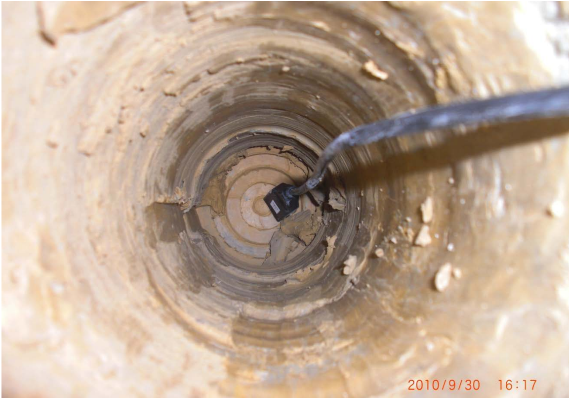
Figure 5.3: A sample installation of a probe installed through the facing of the wall
