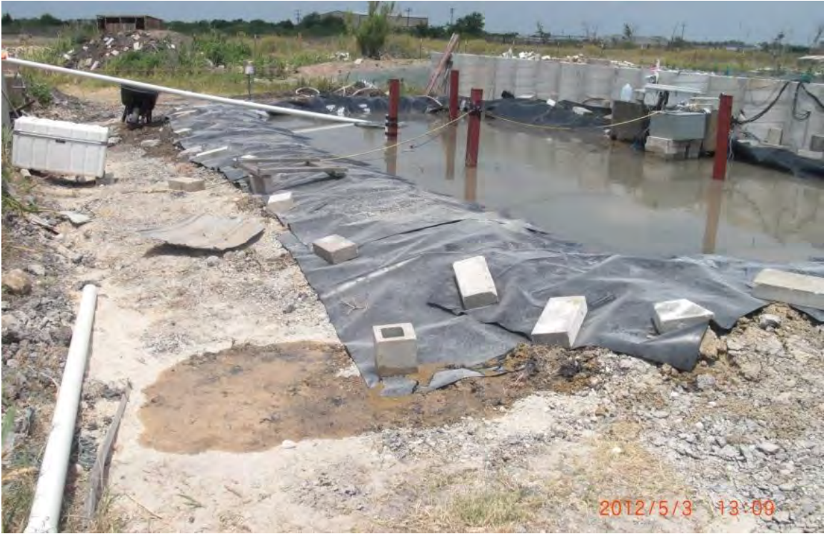
Figure E.52: Leakage from southeast corner of inundation zone.
