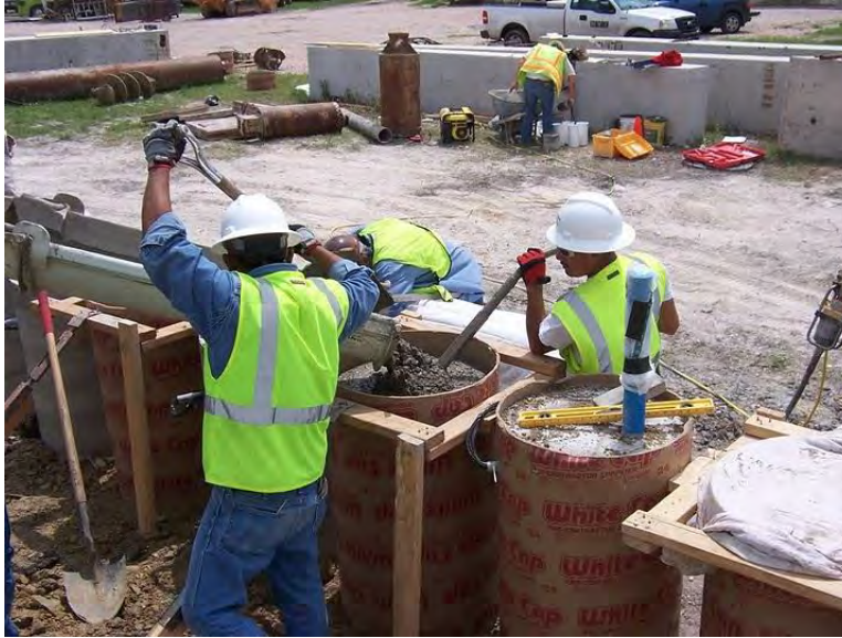
Figure E.11: Vibratory compaction of top of shaft.
