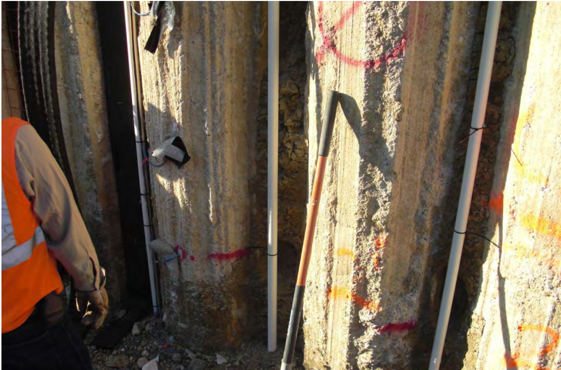
Figure 5.5: The PVC pipe protection for the TDR probe cables to minimize damage from the shotcrete
