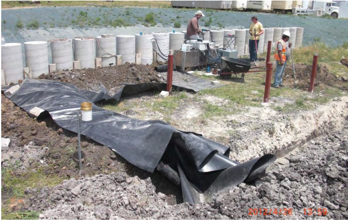
Figure E.46: Installation of geomembrane in trench.
