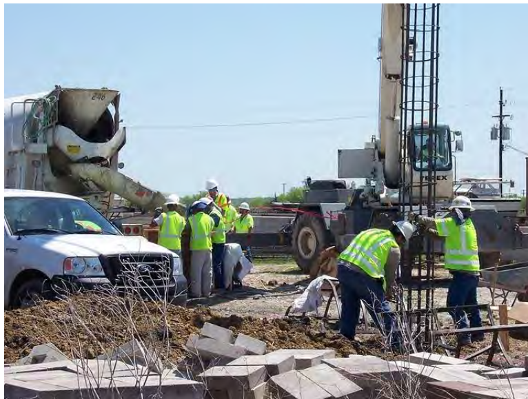
Figure E.9: Rebar cage placed into drilled shaft.
