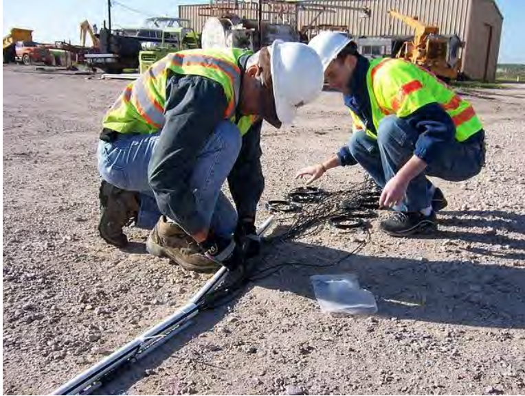
Figure E.14: Securing cables inside slotted PVC pipe.
