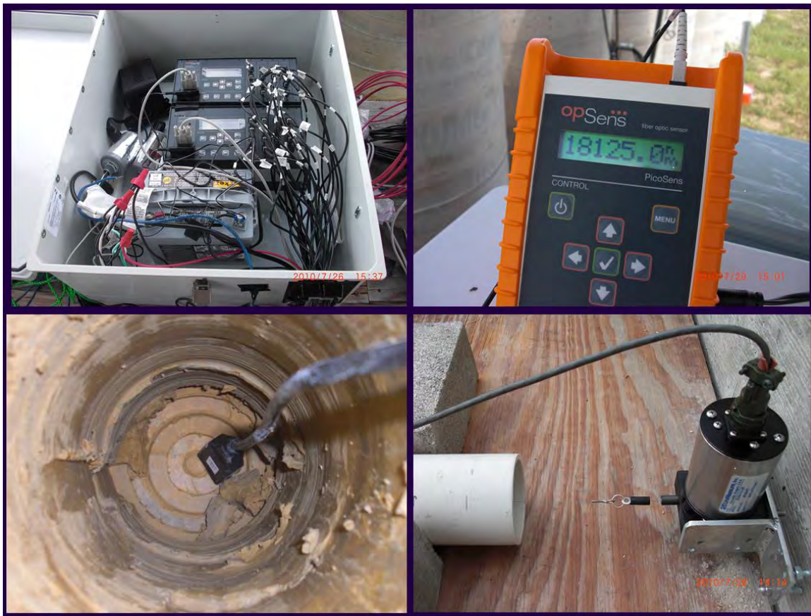
Figure 3.9: Instrumentation on the project site. Clockwise from top left: temperature resistant datalogger and enclosure for continuous strain readings; signal conditioner for individual strain readings; linear potentiometer; TDR probe installed through facing.
