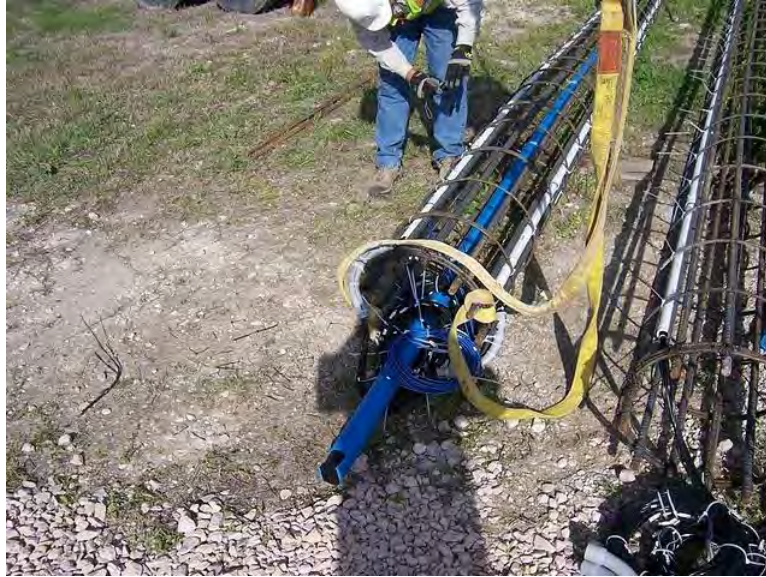
Figure E.17: Placement of cable assemblies during transport of rebar cage.
