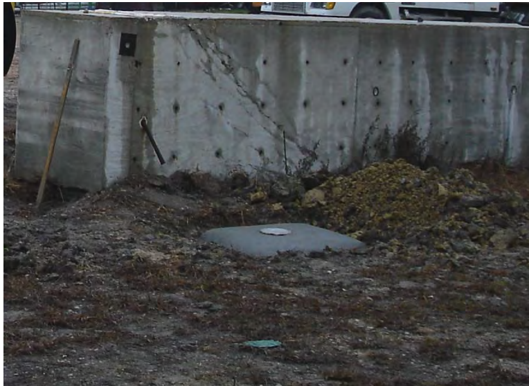
Figure E.25: The piezometer installed and covered in borehole B-3.
