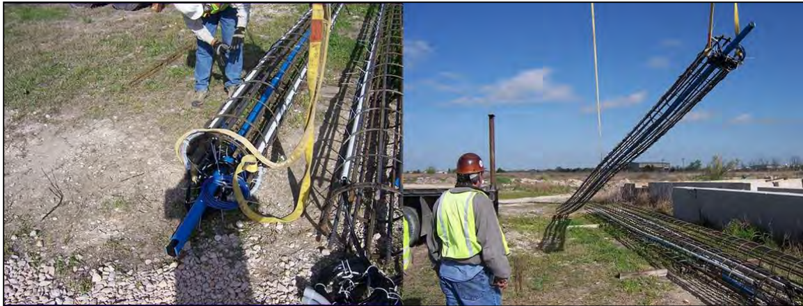
Figure 3.11: Lifting an instrumented cage with two cranes.
