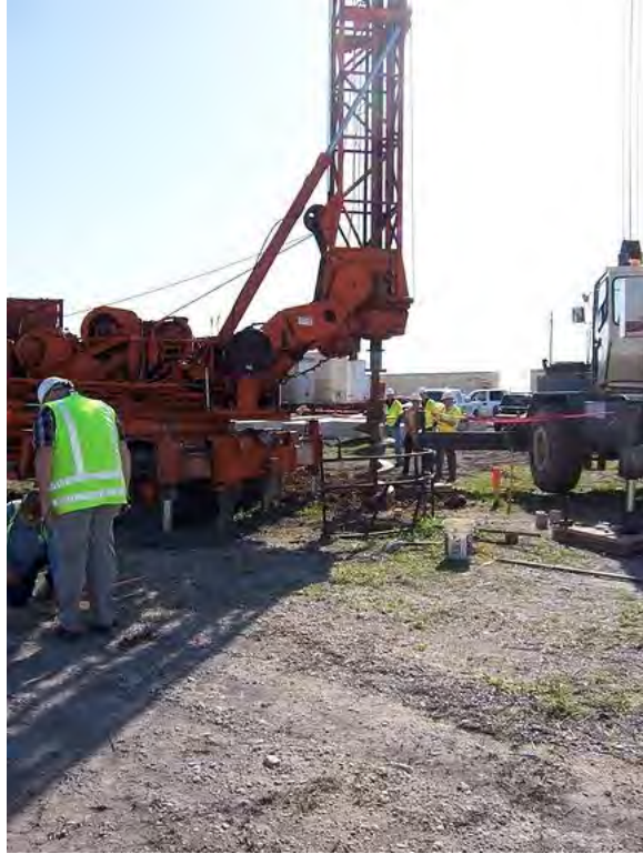
Figure E.3: Rig mobilized to drill the shafts.
