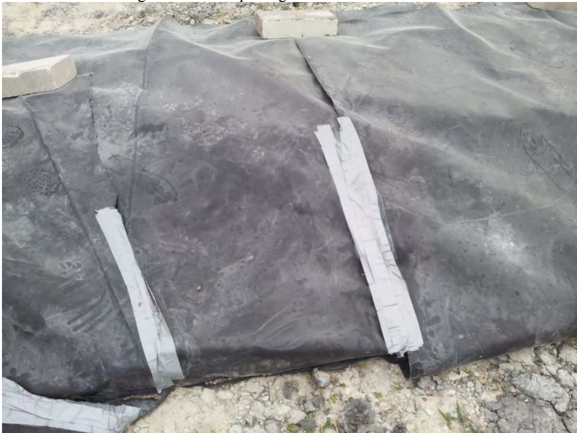
Figure E.49: Detail of geomembrane seam.
