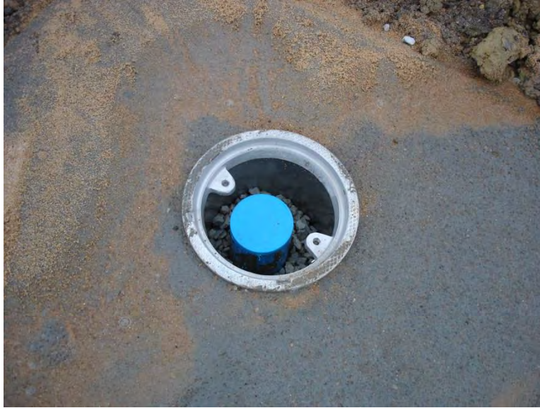
Figure E.21: The inclinometer casing installed behind the wall.
