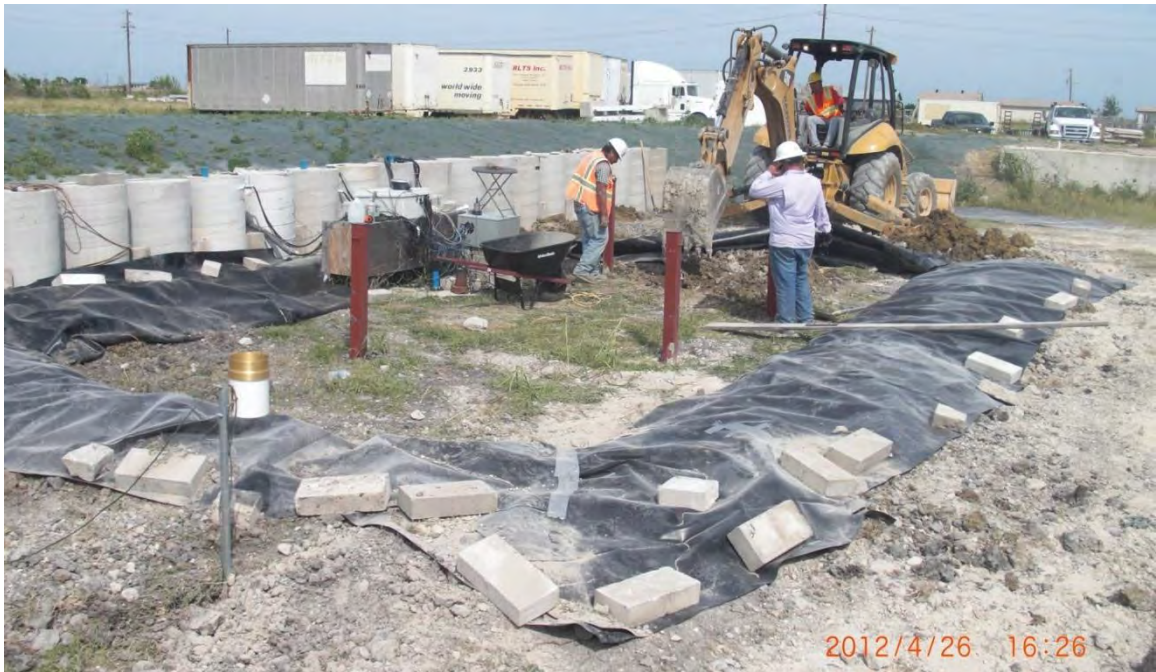
Figure E.48: Compacting soil with backhoe bucket.
