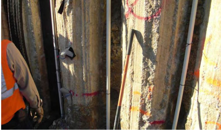
Figure E.31: The PVC pipe protection for the TDR probe cables to minimize damage from the shotcrete.
