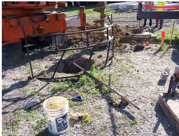
Figure E.5: Plumb-bob for verifying verticality of drilled shaft.
