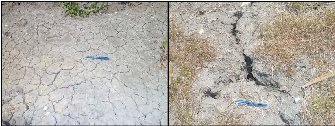
Figure 57. Examples of In-Situ Desiccation Cracking
