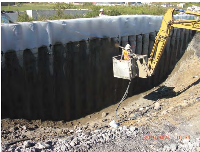
Figure E.34: Placement of shotcrete.
