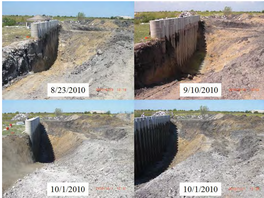
Figure 5.2: Photos of later excavation progress (8/23/2010 - 10/1/2010).
