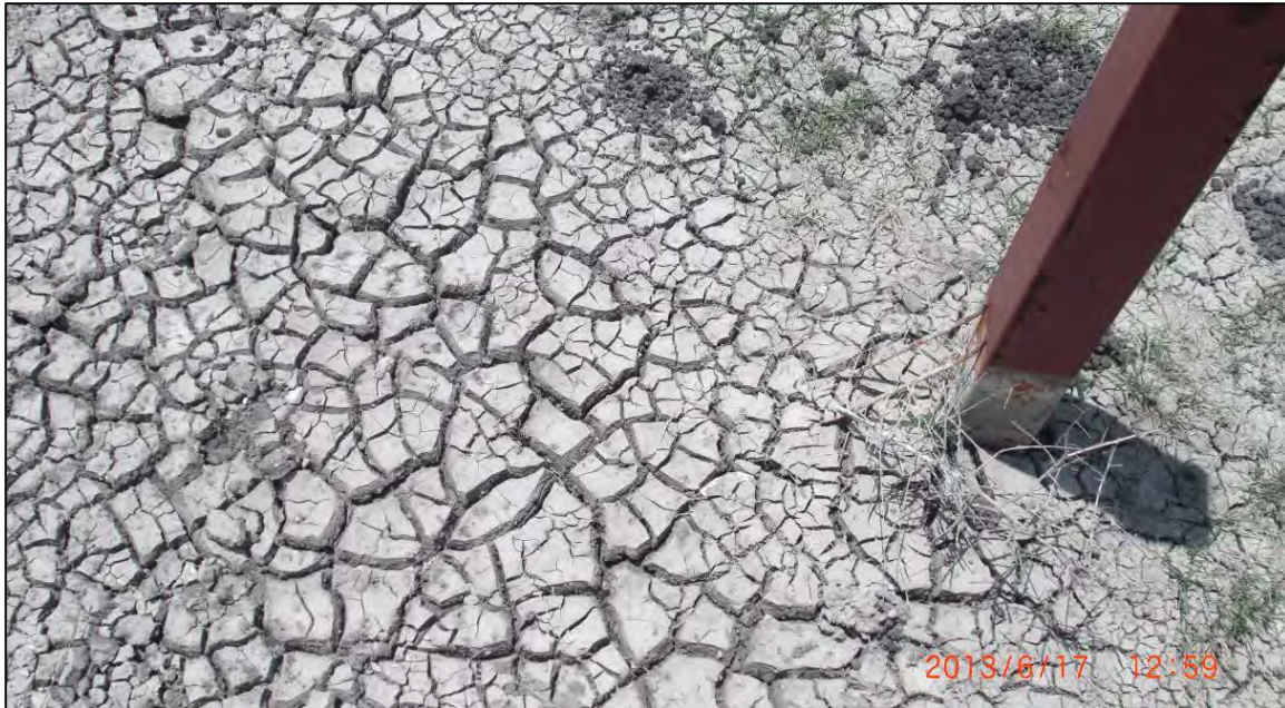
Figure 7.5: Inundation zone on June 17, 2013, two weeks into second drying cycle. Stand pipe piezometer casing is 4" across.
