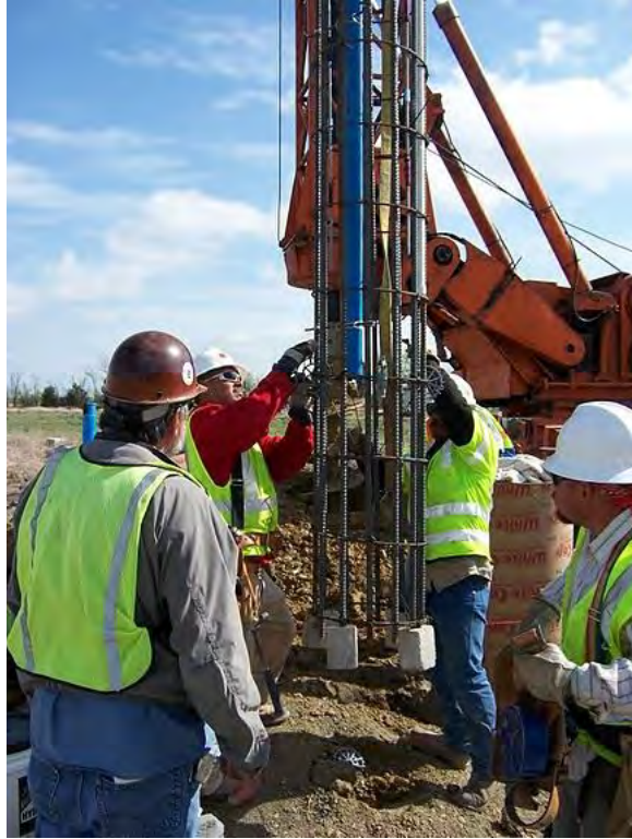
Figure E.8: Installing spacers to the rebar cage.
