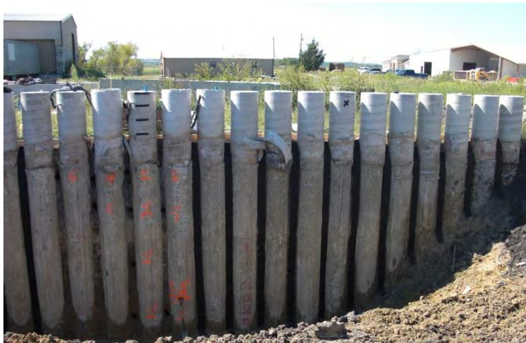
Figure E.33: Installation of the drains on facing of the wall.
