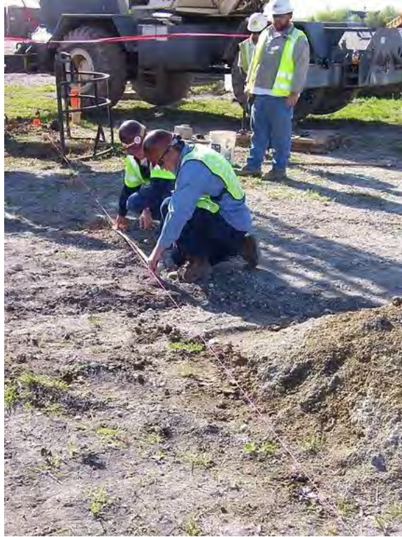
Figure E.4: String line used to mark wall location.
