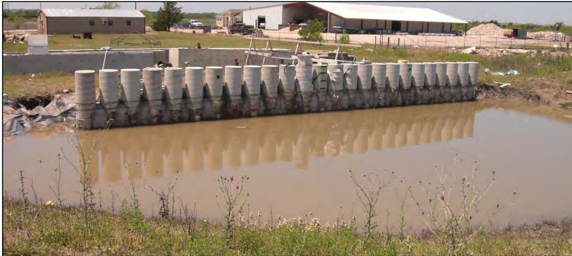
Figure 7.4: Flooding in response to a large storm before the May 6, 2013 data surveys. Water level in the excavation reached ground surface.
