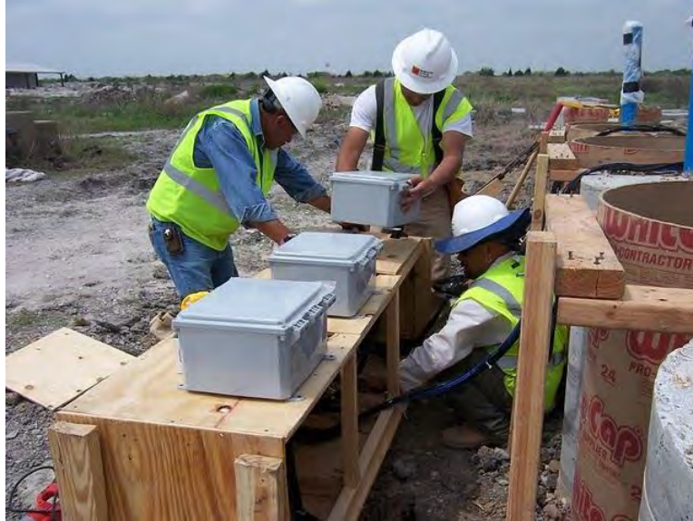
Figure E.19: Construction of platform to house loose cables and hold electrical enclosures.
