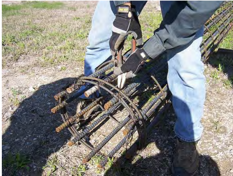
Figure E.2: Additional transverse reinforcement for picking up rebar cages.
