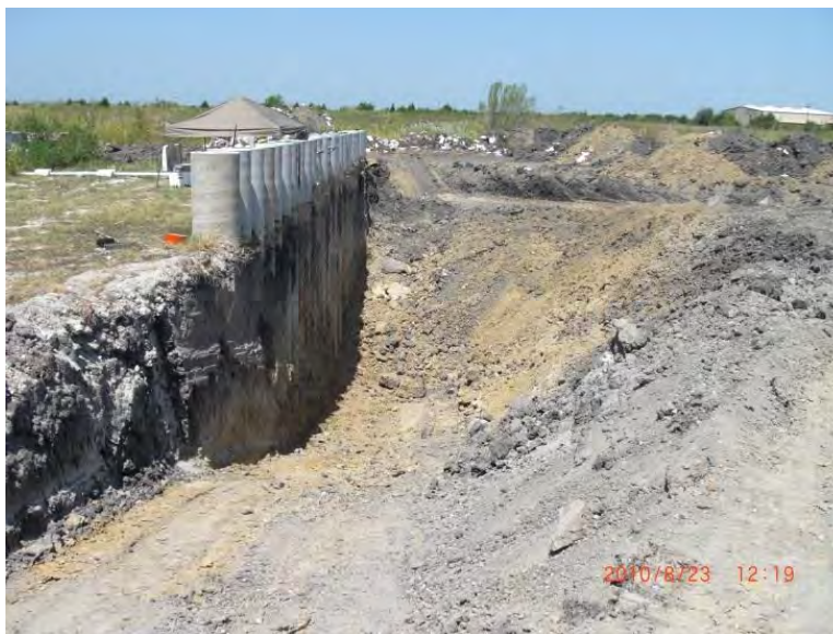
Figure E.39: Excavation process as of 8/23/2010.
