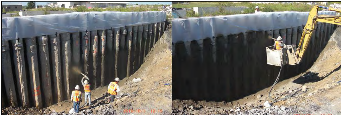
Figure 6.1: Installation of Shotcrete Facing on October 1, 2010.
