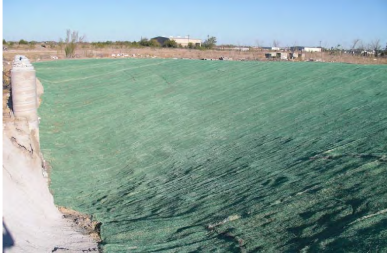
Figure E.42: Excavation after Ranger Excavating reshaped the slopes and applied erosion control.
