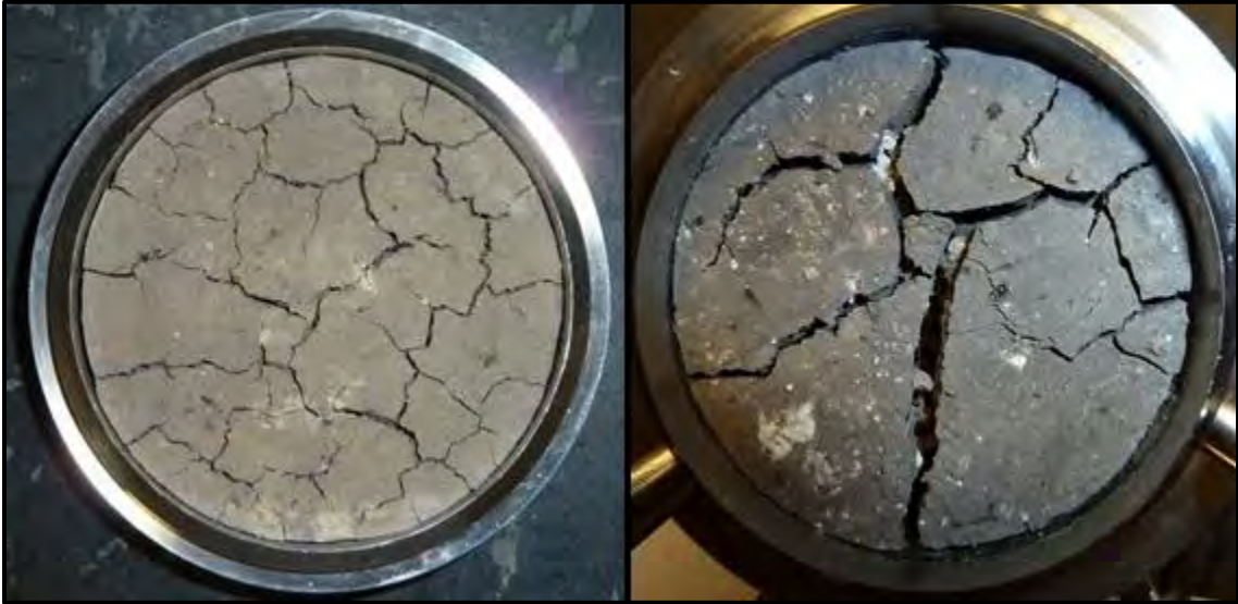
Figure 56. Examples of Extreme Cracking from Shrink Stage of Cyclic Swell Test
