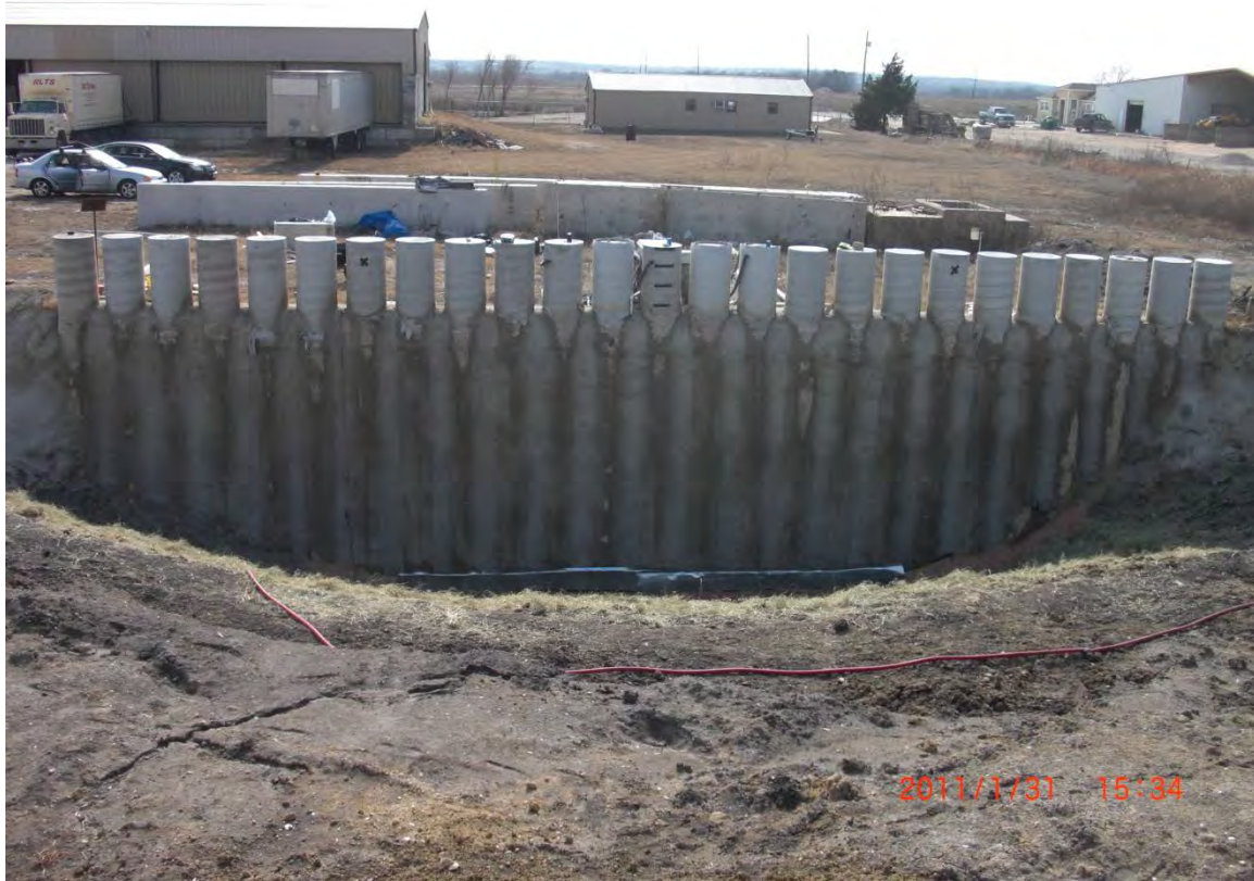
Figure 3.1: A view of the test wall after excavation and installation of the shotcrete facing
