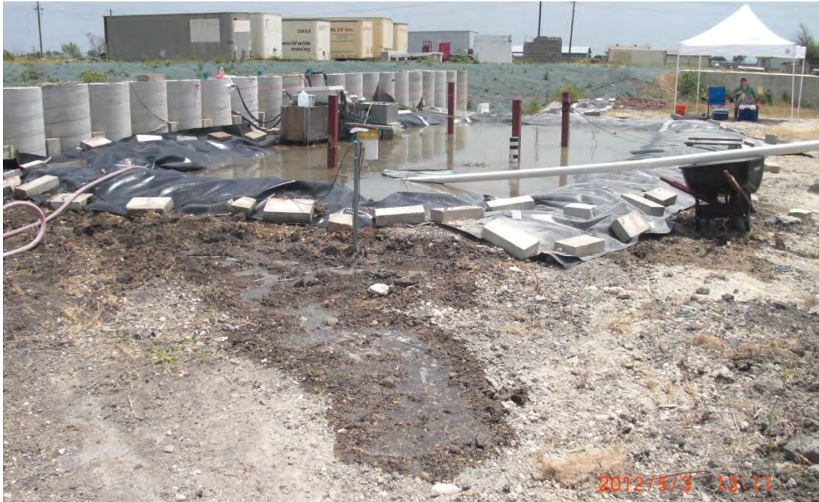
Figure E.53: Leakage from west side of inundation zone.
