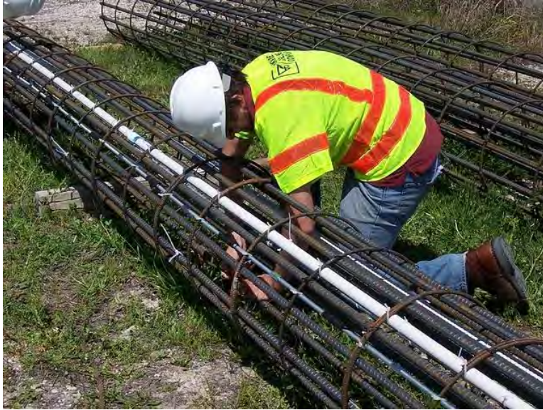
Figure E.16: Sister bars and PVC pipes being tied to rebar cage.
