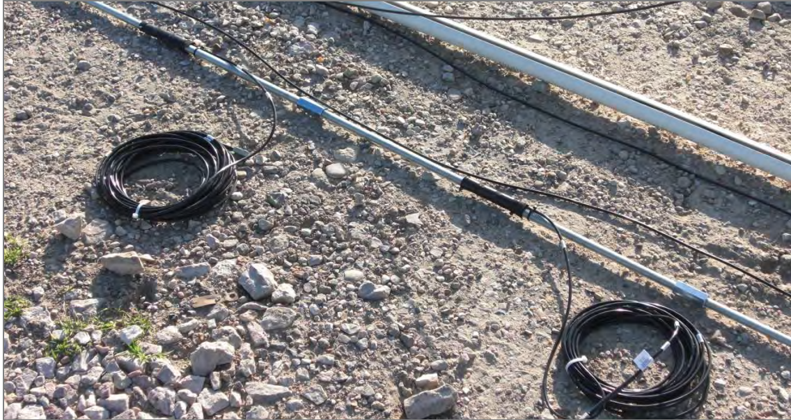
Figure 3.15: Strain gauges attached to the sister bar before installation within the shafts
