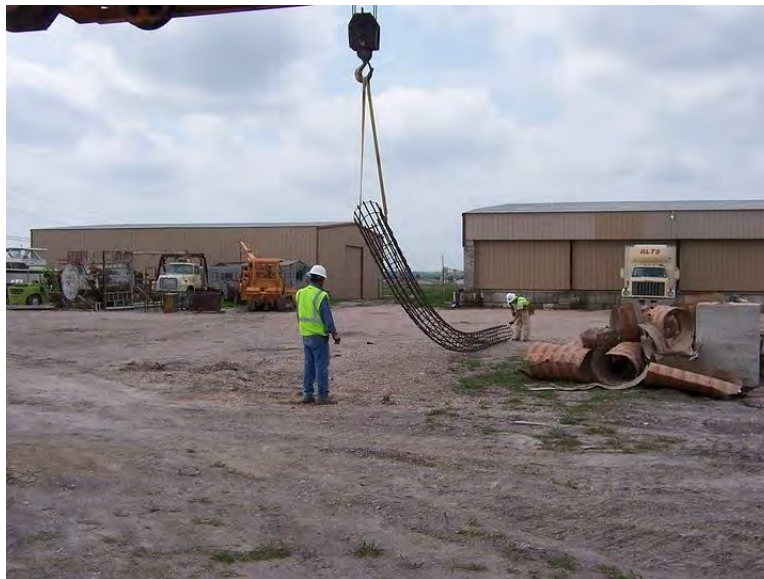
Figure E.6: One-point pickup for non-instrumented shafts.
