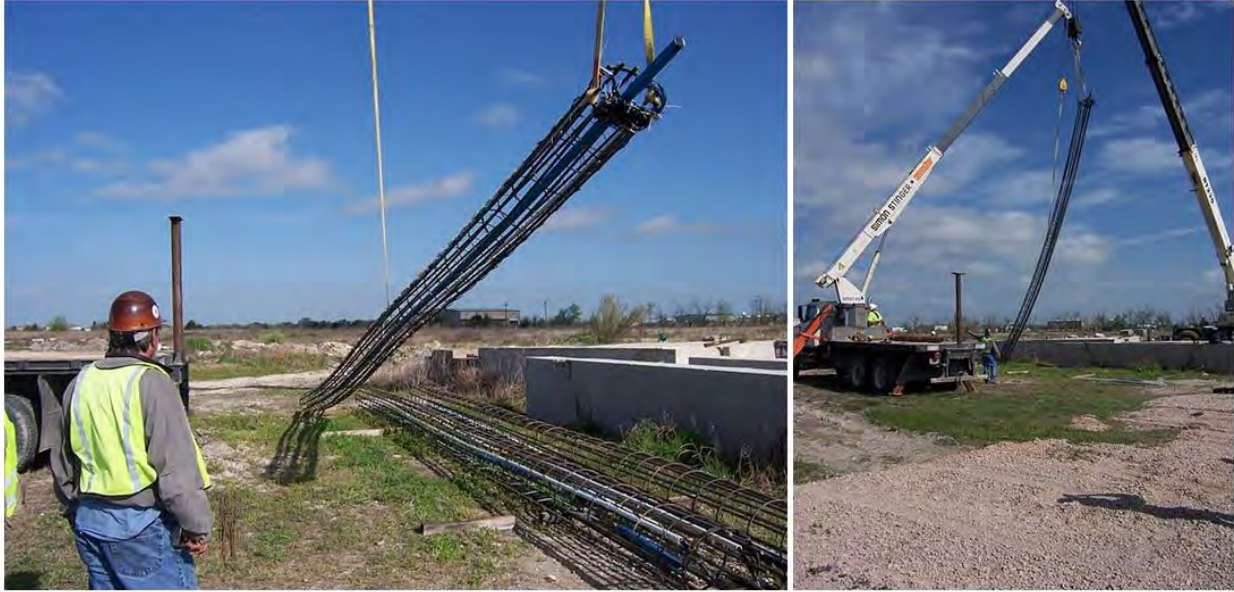
Figure E.7: Two-point pickup for instrumented shafts.
