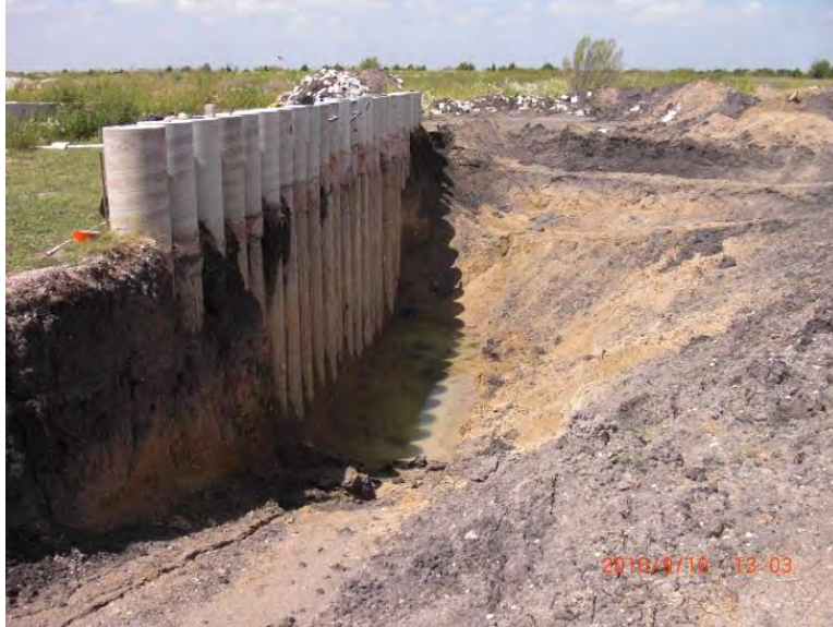
Figure E.40: Excavation process as of 9/10/2010.
