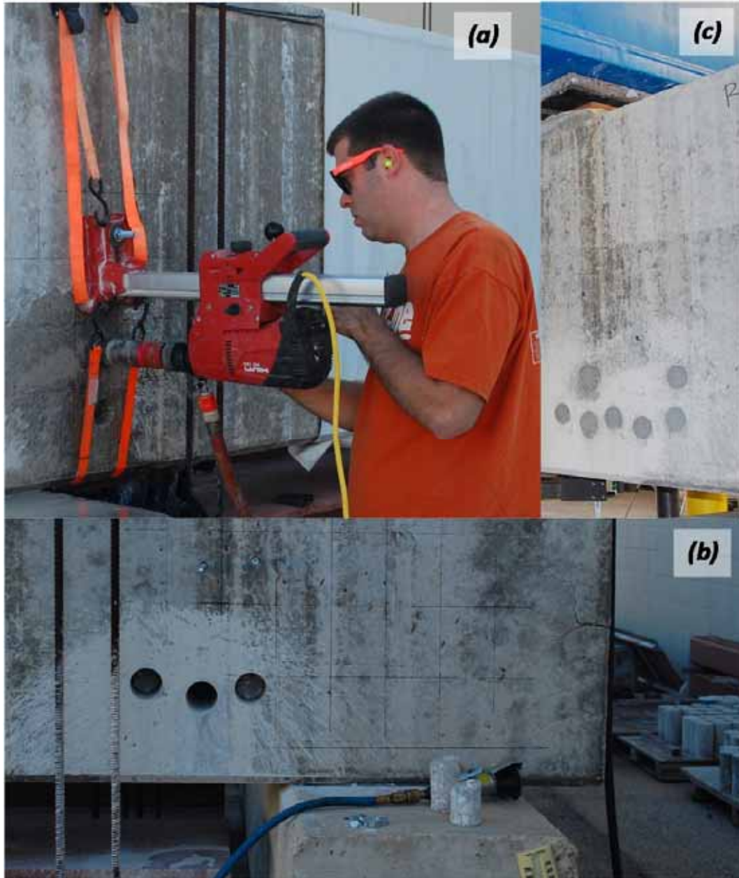
Figure 6.1: Extraction of 2 in. (51 mm) diameter cores from second reactive specimen and repaired core holes.
