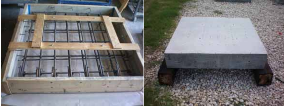
Figure 3.5: Bridge deck forms (left) and completed specimen on rail ties (right).
