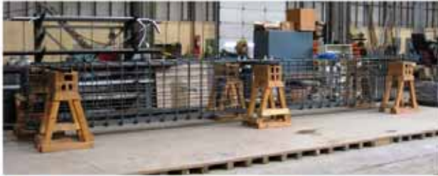
(a) Construct reinforcement cage
