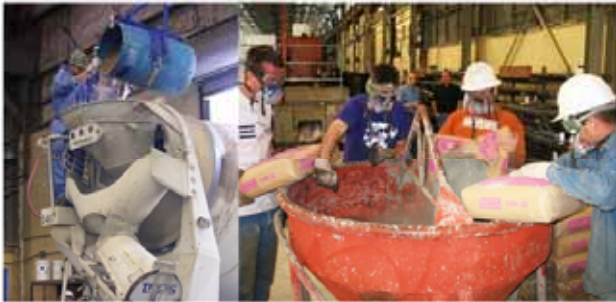
(c) Mix concrete
