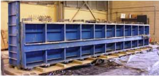
(b) Erect formwork, place cage inside
