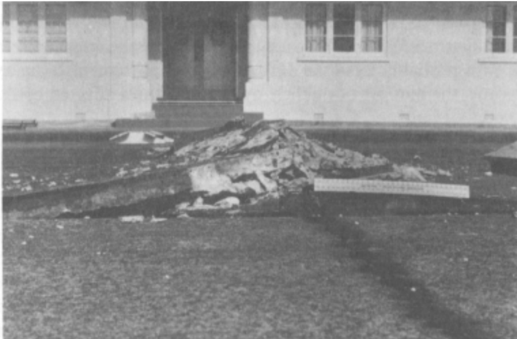
Figure 2.3: Crushing failure of pavement from ASR, from Swamy 1992.
